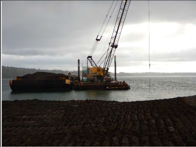
Comment: Placing 3" minus backfill in SMA-2
