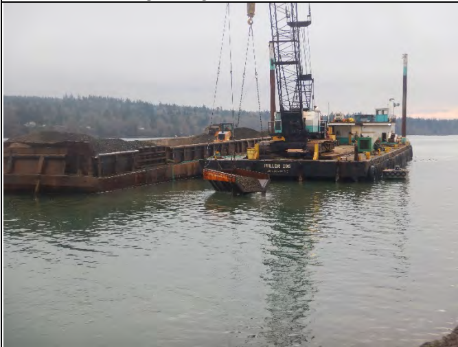
Comment: Placing 3" minus backfill in SMA-2 with rock box
