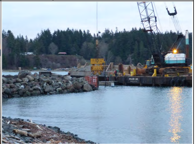
Comment: Pulling temporary piles at transload facility
