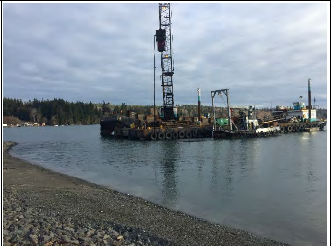
Comment: Removal of remaining pilings (diver-assisted)
