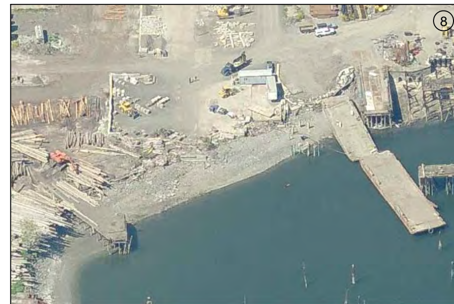
PHOTO 8: PIER 4 AND PIER 5
