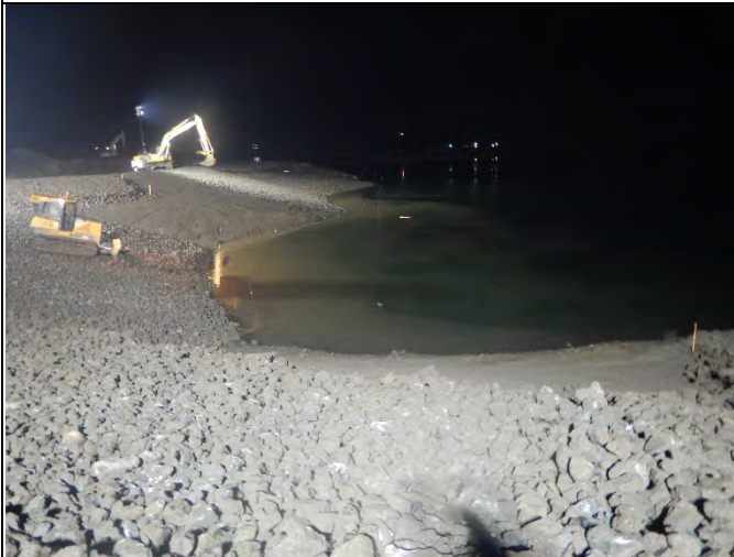
Comment: Pier 4 capping area
