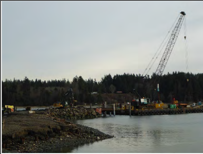
Comment: Removing decking and crane mats from transload
