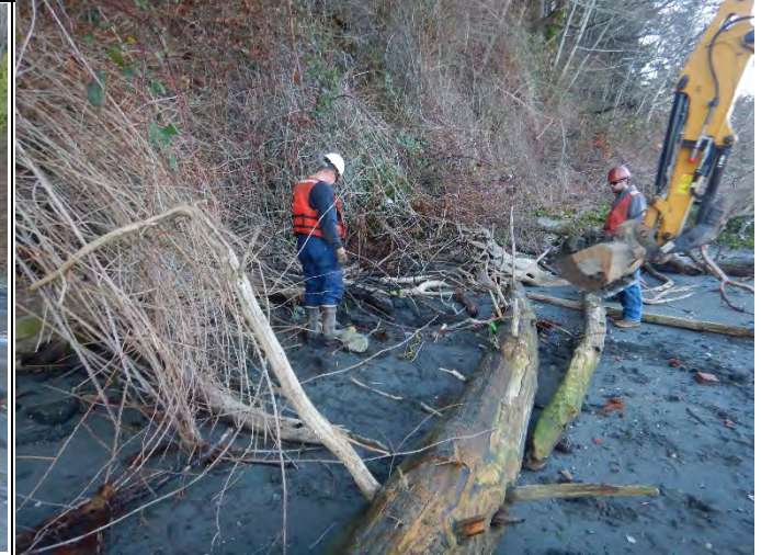
Comment: Removal of asphalt debris in Area 1
