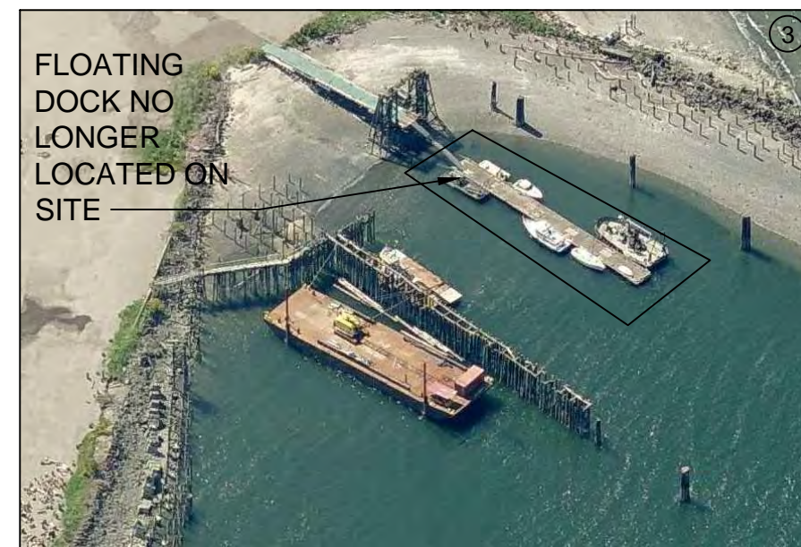
PHOTO 3: CONVEYOR/PIER (FROM BING MAPS IMAGERY)
