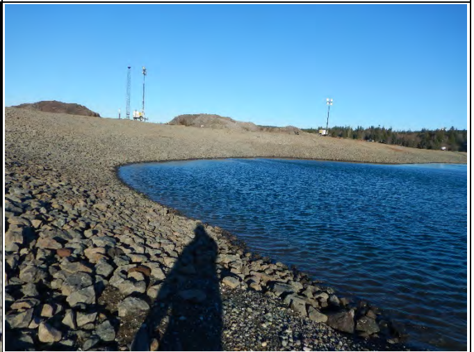
Comment: Completed Pier 4 cap area
