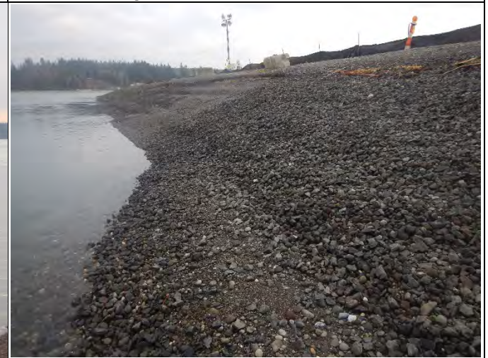
Comment: SMA-1 intertidal cap slope
