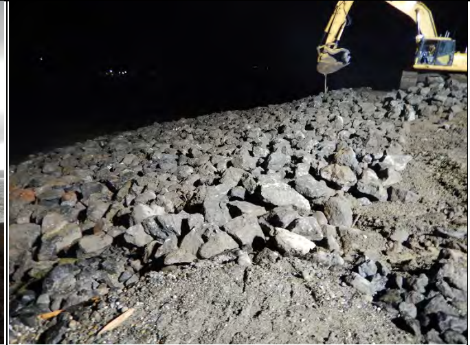
Comment: Placing armor rock in erosion area 1 (pocket beach)
