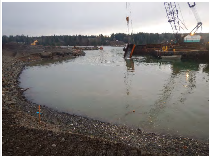
Comment: Placing 3" minus backfill in SMA-2
