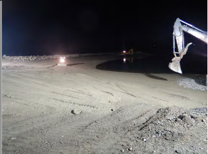
Comment: Placing habitat substrate in final section of SMA-1 intertidal cap
