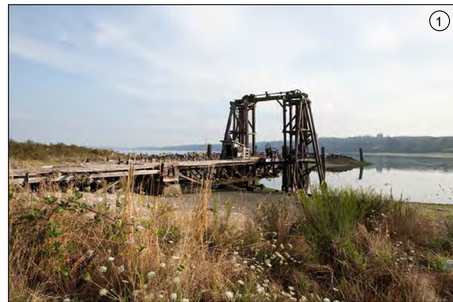
PHOTO 1: LOG TRANSFER DOCK
