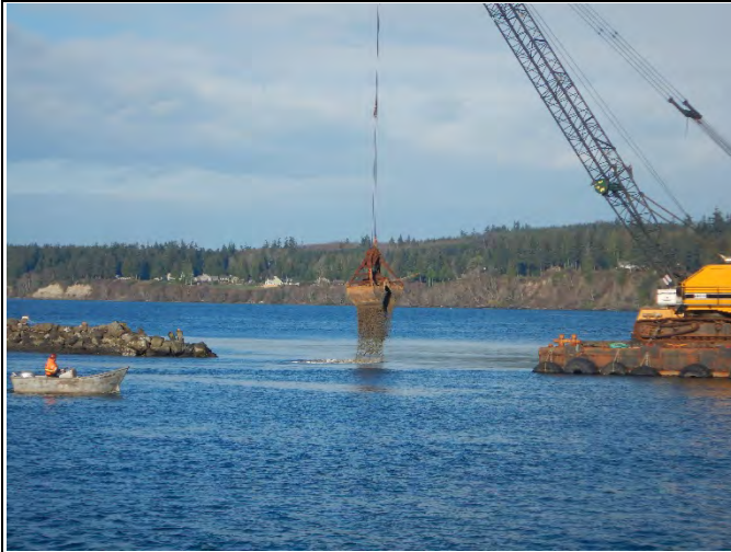
Comment: Placing EMNR material in SMA-1
