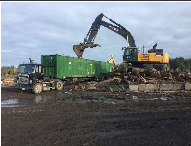
Comment: Processing creosote pilings for off-site disposal
