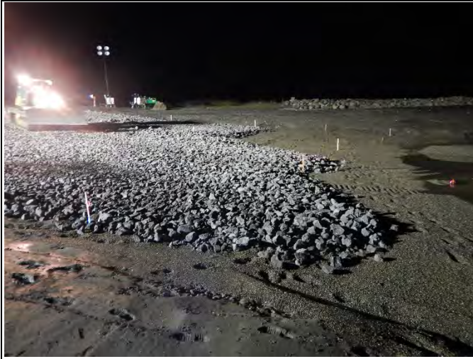
Comment: Placing armor in final section of SMA-1 intertidal cap
