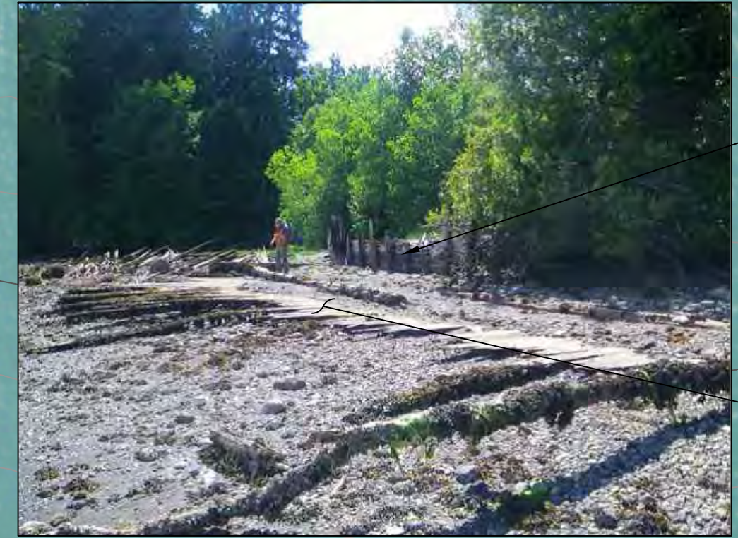
PHOTO 11: LANDFILL 4A AND 4B SURFICIAL BEACH DEBRIS
