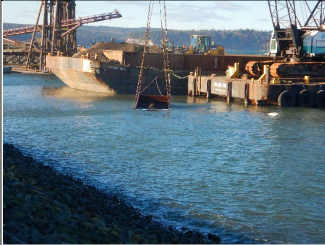
Comment: Placing 3" minus backfill in SMA-1
