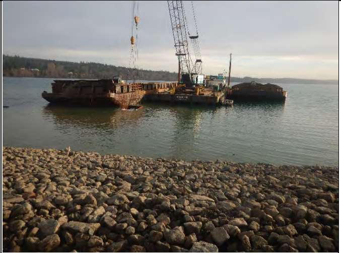
Comment: Placing 3" minus backfill in SMA-2
