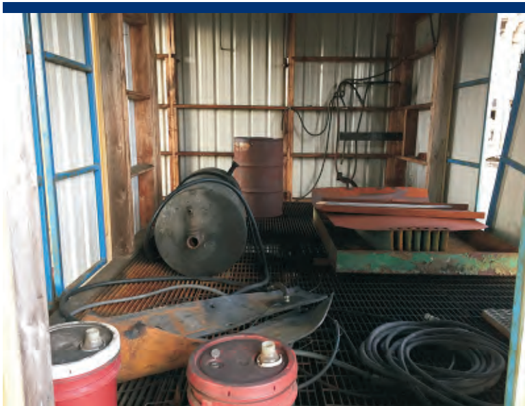
Photo 39 Interior of Oil Storage at east side of Main Shipping Shed.
