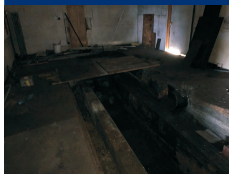
Photo 18 Interior of what appears to have been spray mixing area.
