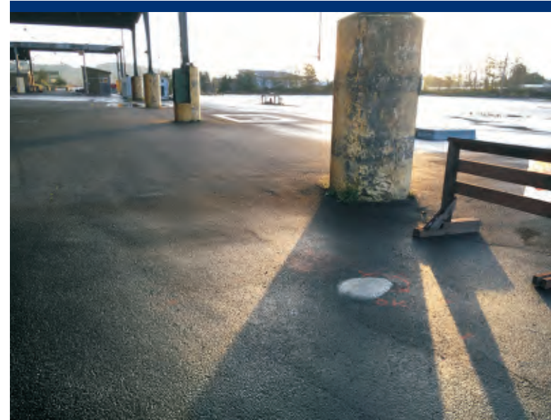
Photo 38 Boring location NA01, patched.
