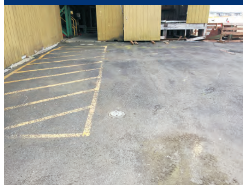
Photo 6 Monitoring well near northeast corner of Planer Building.
