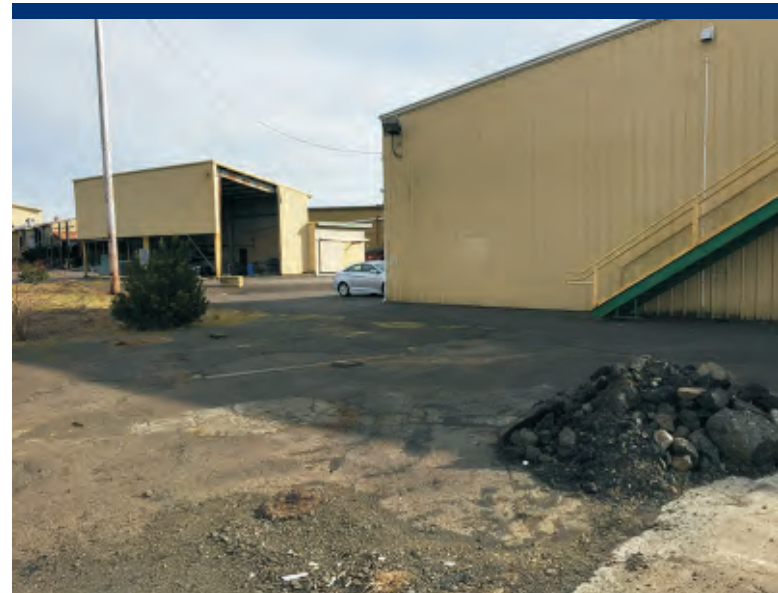
Photo 4 Maintenance shop and fuel/chemical storage building.
