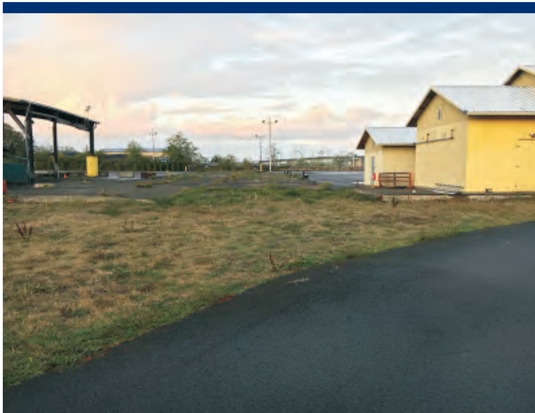
Photo 39 Area north of inner harbor line. Reported to have been location where 5000-gallon (approx.) USTs removed in 1987.
