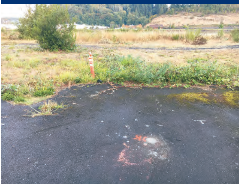
Photo 1 Boring location MS01, patched.
