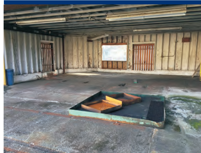
Photo 22 Southern interior of Stacking area of Planer Building.
