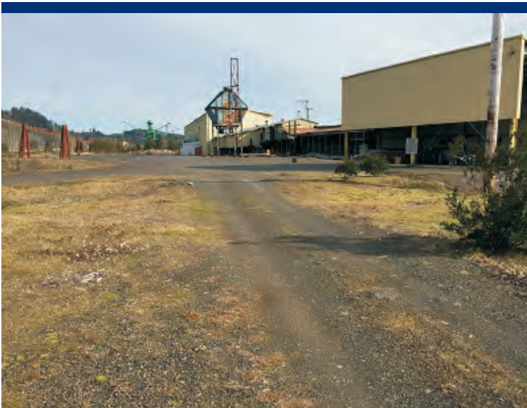
Photo 3 View of small log mill and fuel/chemical storage building from north of maintenance shop.
