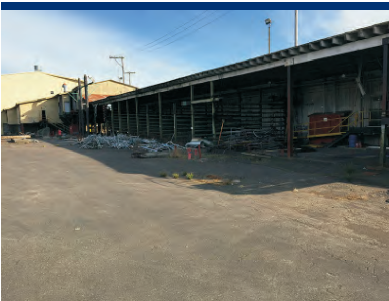
Photo 31 North side of shipping shed.
