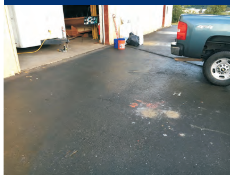
Photo 2 Boring location MS02, patched.
