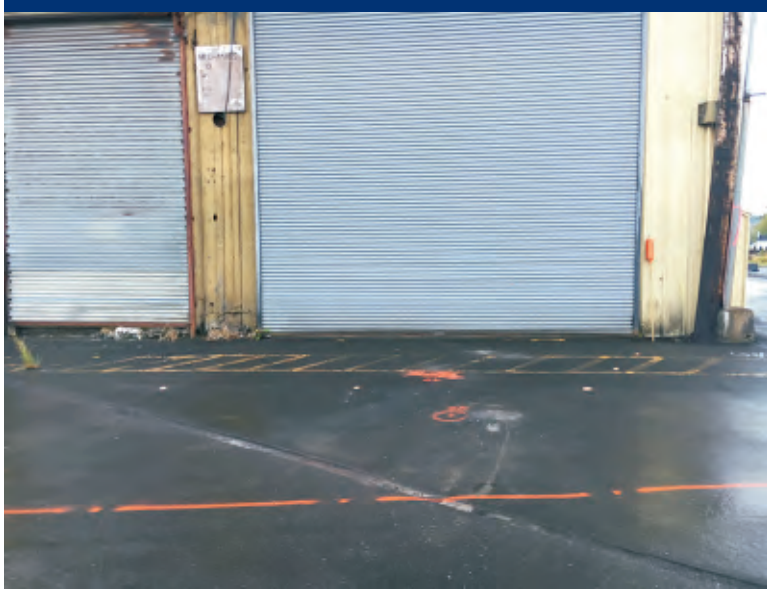
Photo 37 Boring location VM01, patched.
