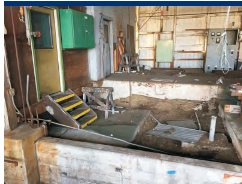
Photo 16 West interior of Planer Building.
