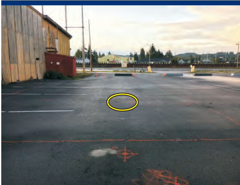
Photo 33 Boring locations OC01 (background) and OC02 (foreground), patched.
