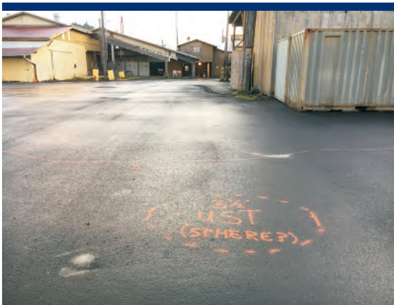
Photo 35 Boring location OC03 (patched) and UST/sphere identified by geophysical contractor.
