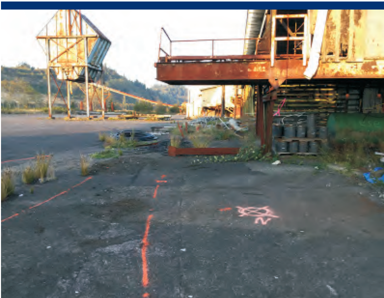
Photo 15 Located lines by geophysical contractor and location FC03 before drilling.
