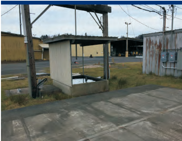
Photo 43 Containment interpreted as location of backup generator diesel AST. Former transformer pad in front.
