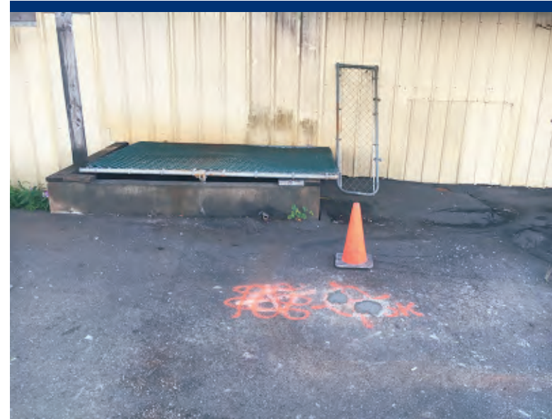
Photo 22 Boring location PB02, patched. Adjacent to suspected hydraulic oil containment vault.
