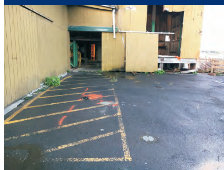
Photo 30 Boring location PB06, patched, with well D-04e in foreground.
