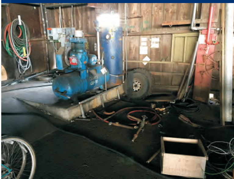
Photo 41 Compressor and discolored concrete at northwest corner of shipping shed near vehicle maintenance area.
