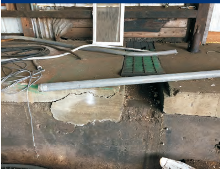
Photo 17 Trench drain type feature on west side of Planer Building.
