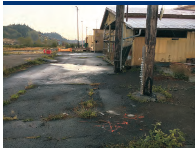
Photo 20 Boring locations PB01 (background) and PB09 (foreground) on north side of planer building.
