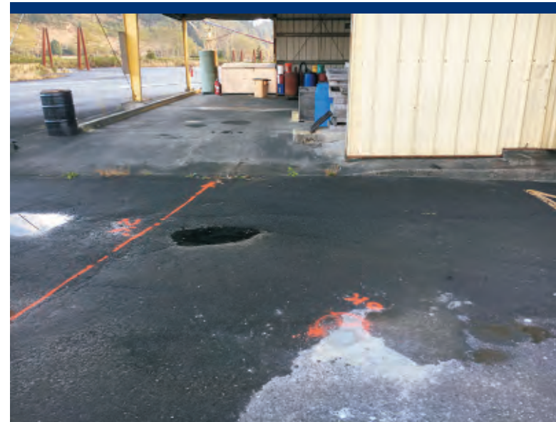
Photo 12 Boring location FC02, patched.
