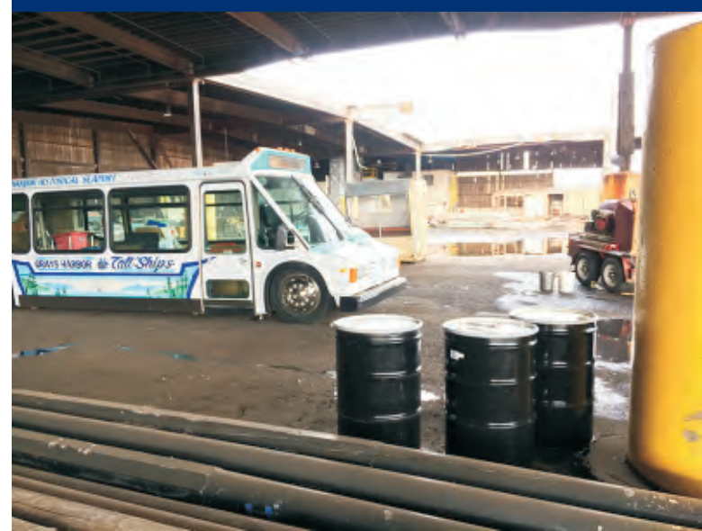
Photo 42 Labeled IDW drums, stored under cover.
