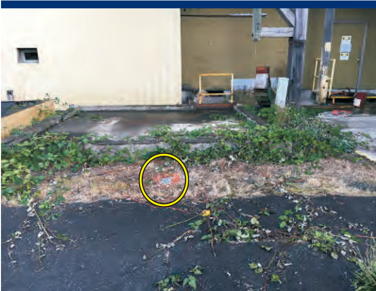
Photo 25 Boring location PB03 and adjacent containment curb/vault, interpreted as past transformer location.
