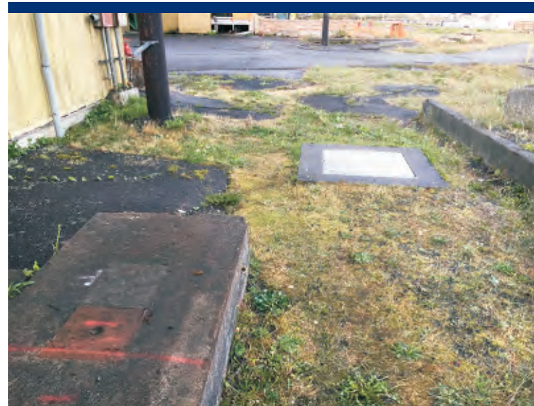
Photo 8 Location where power appears to enter maintenance shop from transformer vault.
