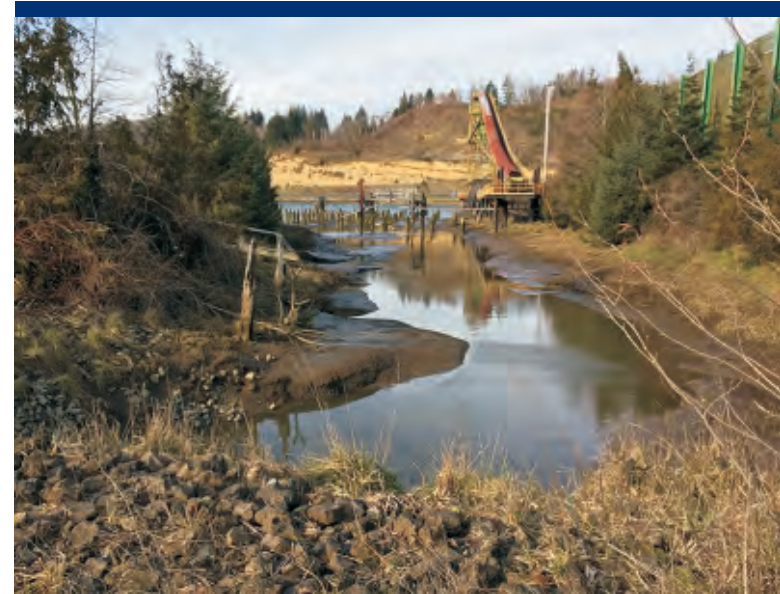
Photo 34 Northern end of slough and chip area blower building on east side of site.
