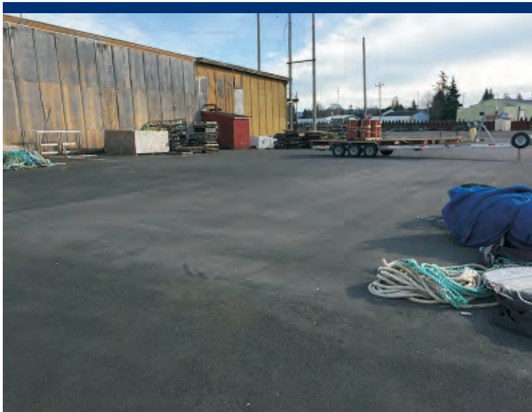
Photo 19 Southwest corner of storage building. Former oil tank and chemical storage shed at near side of building.
