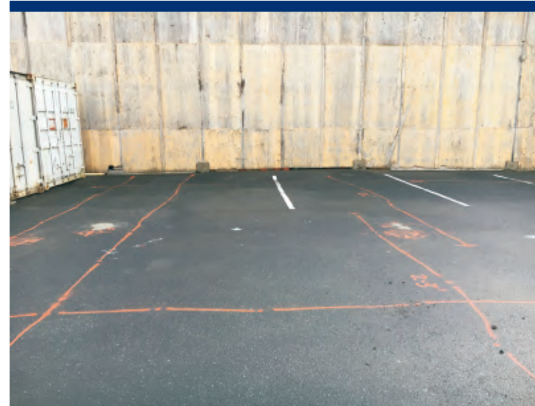
Photo 34 Boring locations OC01 (right) and OC02 (left), patched.
