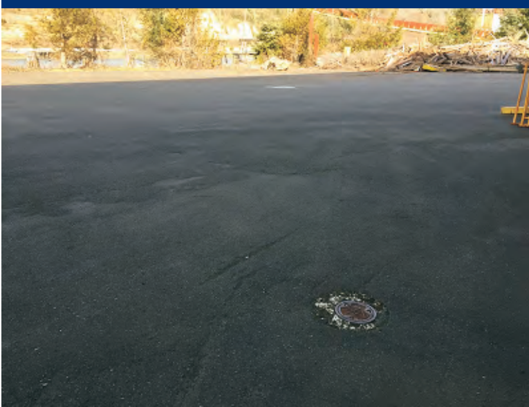
Photo 33 Monitoring well on north side of small log mill.
