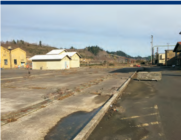
Photo 15 View along foundation for former Green Chain building.
