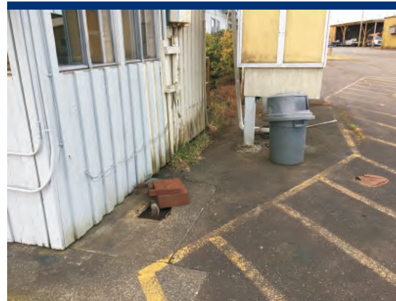
Photo 44 Interpreted UST fill line remaining on north side of guard shack.
