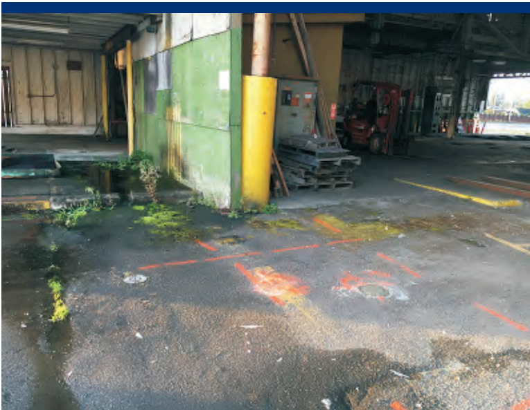
Photo 31 Boring location PW01 (right) and monitoring well D-02 (left).
