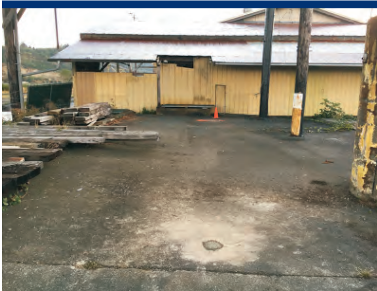
Photo 21 Boring locations PB10 (foreground) and PB02 (cone, background), patched.
