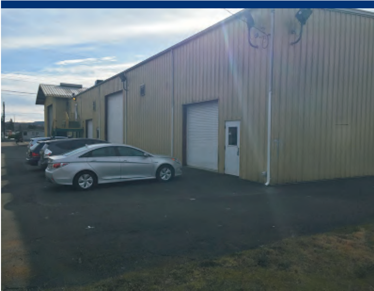
Photo 1 Northeast corner of maintenance shop, near previous boring location.
