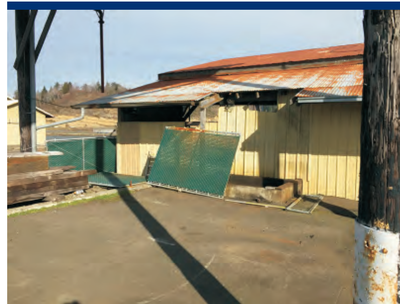
Photo 12 Additional containment curbed area on west side of Planer Building.
