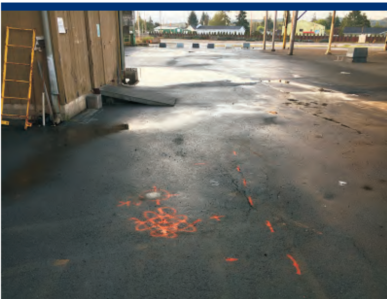
Photo 27 Boring location PB05, patched.
