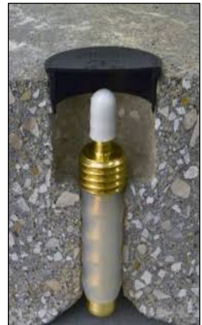
Photo 2. Vapor Pin in Concrete Slab
