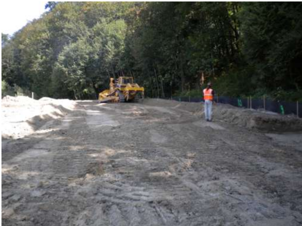
Photograph 4: Removing clean overburden on east half of Site, August 19, 2010.
