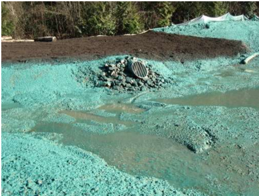
Photograph 21: Hydroseed on north portion of Site by detention pond and wetland buffer, February 2, 2011.
