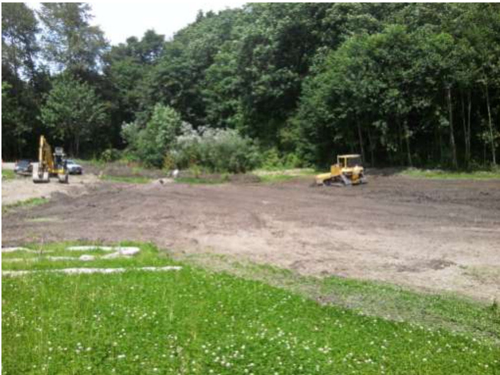
Photograph 24: Final grading at north end of Site, June 30, 2011.
