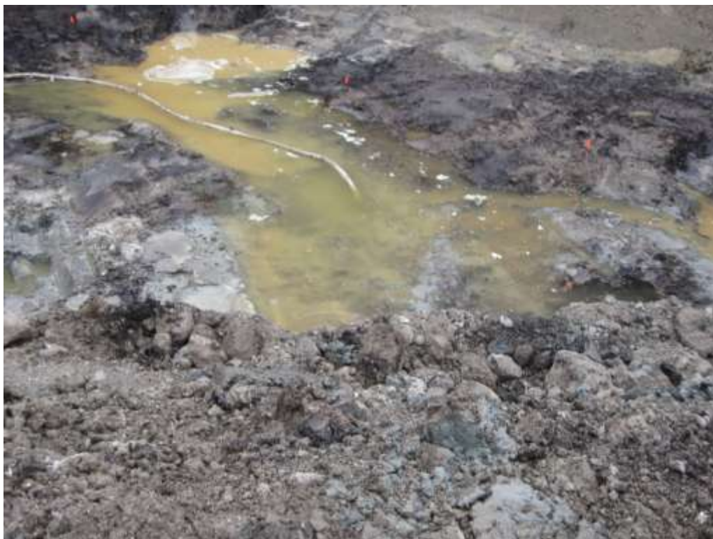
Photograph 12: Dewater low spot in center of excavation, September 18, 2010.
