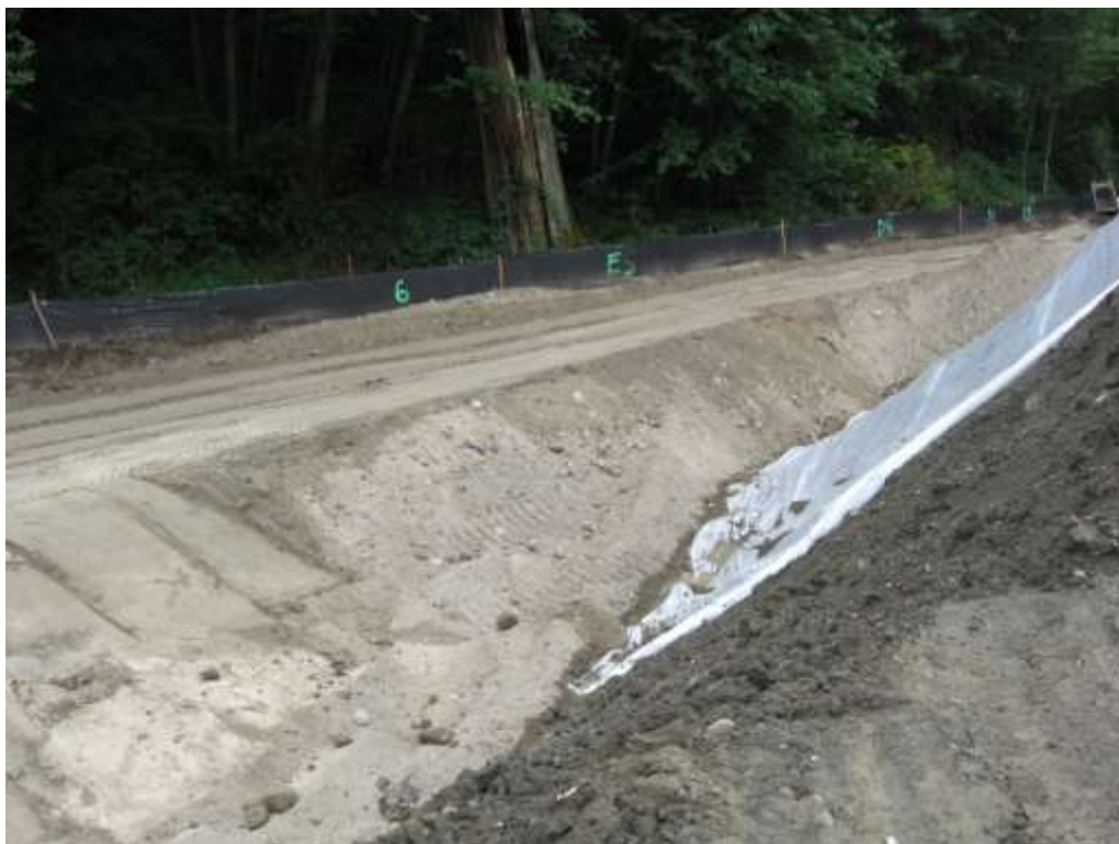
Photograph 10: Clean backfill on east portion of Site, September 9, 2010.
