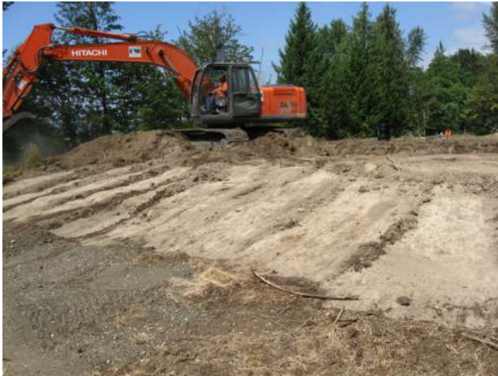
Photograph 3: Removing topsoil at center of Site, August 18, 2010
