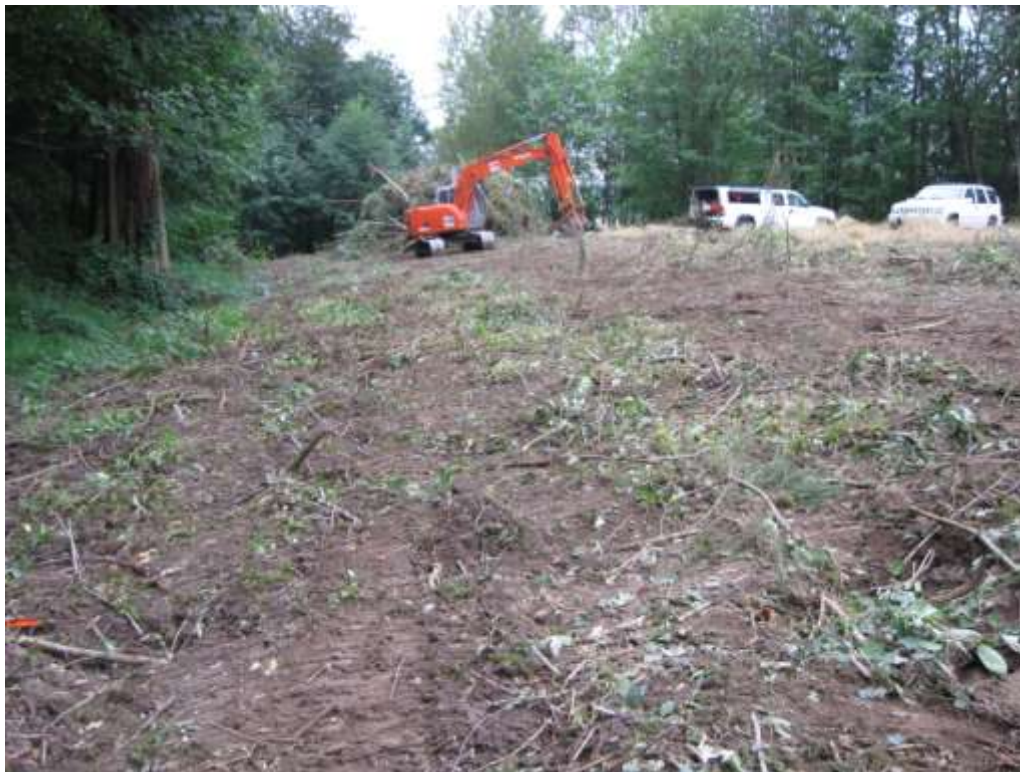
Photograph 1: Removing vegetation on east half of Site, August 9, 2010.
