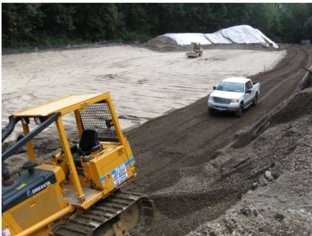
Photograph 14: Compacting clean backfill on east half of Site, October 8, 2010.
