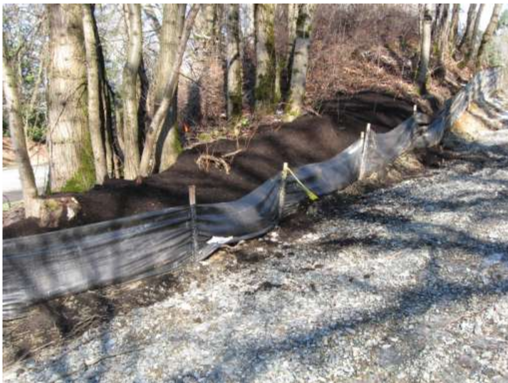
Photograph 22: Completed wetland M restoration near southwest Site entrance, February 25, 2011.
