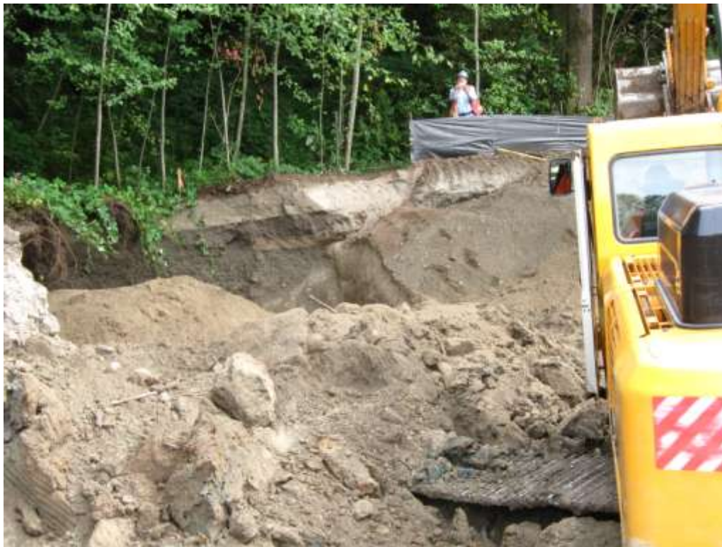
Photograph 11: Slot-cut at northeast side of Site, September 16, 2010.
