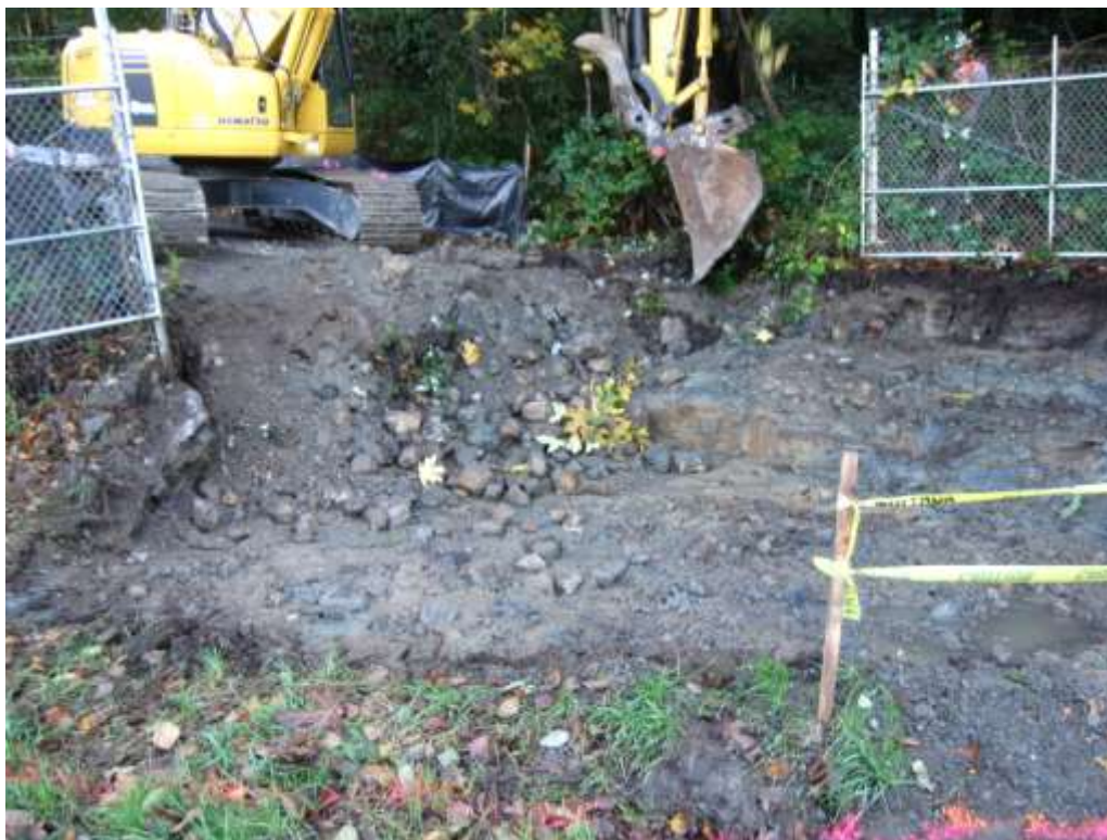
Photograph 17: Removing slag from between gates at southwest entrance to Site, October 25, 2010.
