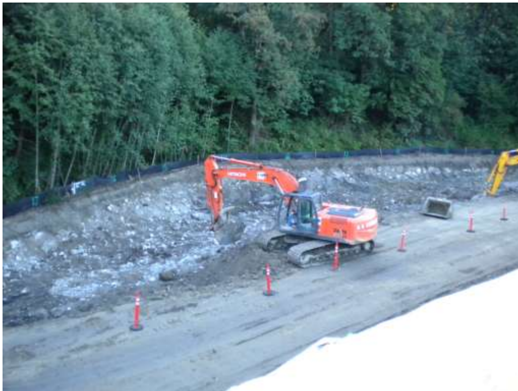
Photograph 7: Removing slag on east portion of Site, September 1, 2010
