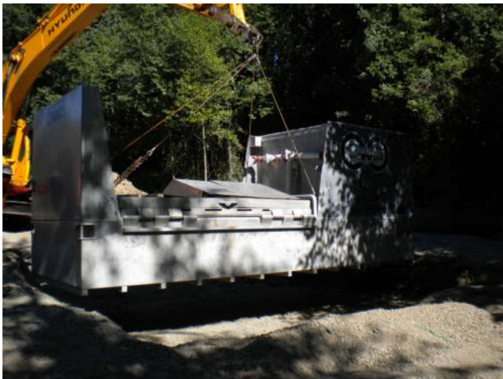
Photograph 6: Installing wheel wash on south portion of Site, August 22, 2010.
