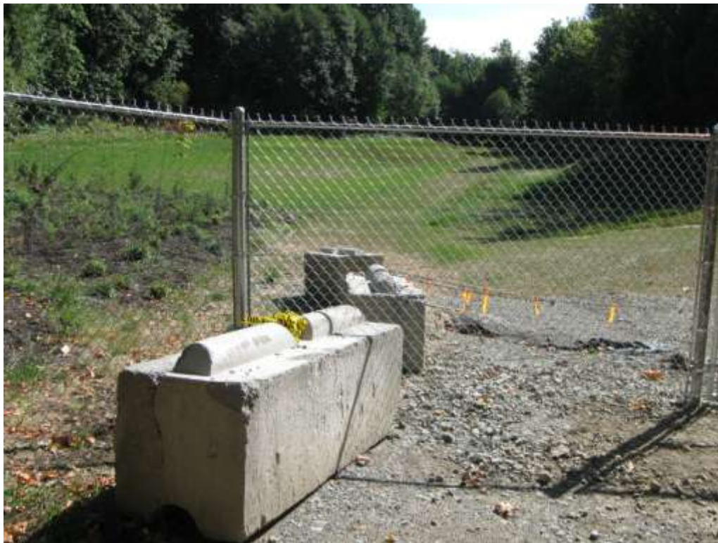
Photograph 25: Restoration of re-graded areas, September 2, 2011.
