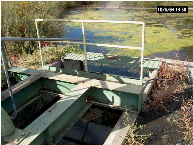
The river water intake gate was constructed of concrete and metal. The intake received water from the intake channel to the north. Excess water overflowed to the east at the spillway and into the overflow channel at right, beyond the view of the photograph.
