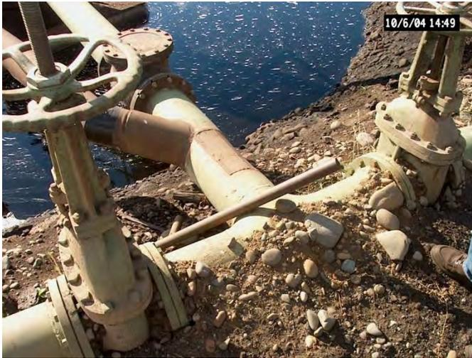
Water supply from the pumps could be directed to sprinkler connections to the south and the north main line sections.
