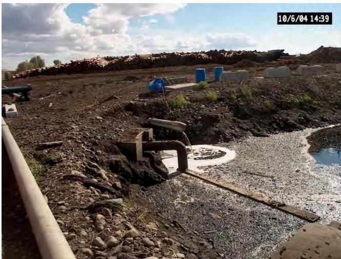
Sodium hypochlorite being added to the recycle pond. Return flow from the sprinkler water return ditch is present at the center of the photograph. The return flow is visibly discharging from a white polyvinyl chloride pipe visible near the center of the photograph,
