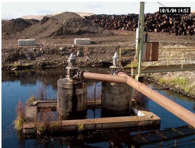
The recycle pond was equipped with two electric motors that pumped water from the pond into the log deck sprinkler system.
