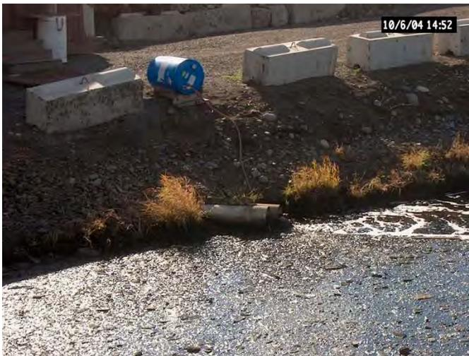
Sodium hypochlorite solution being added to the settling pond.
