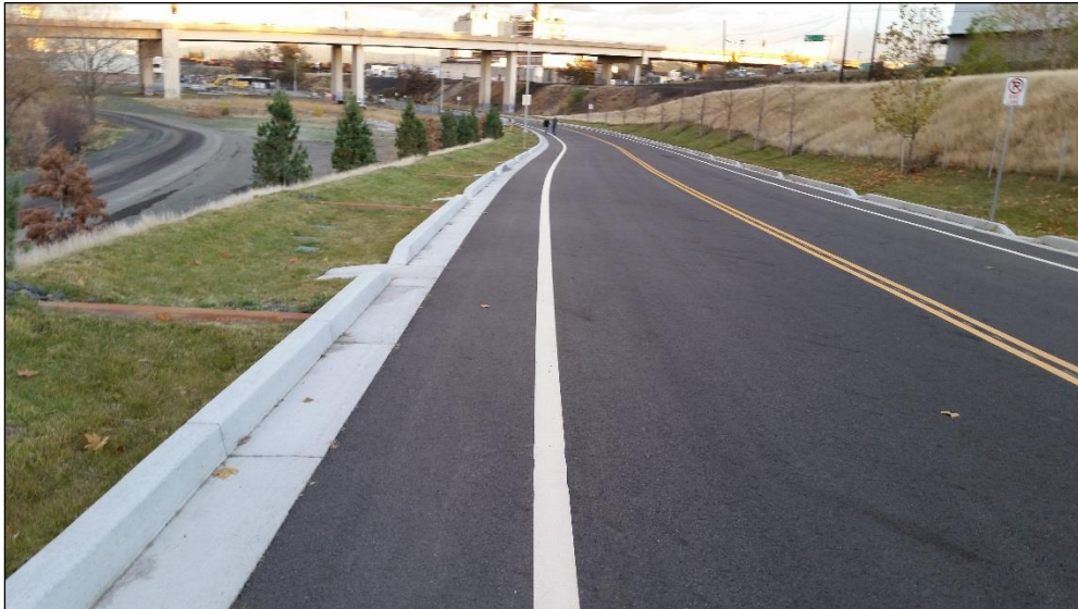
1. View of new MLK Jr Way on Hamilton Street Bridge Site (looking east from west site boundary). New Ben Burr Trail is to the left.
