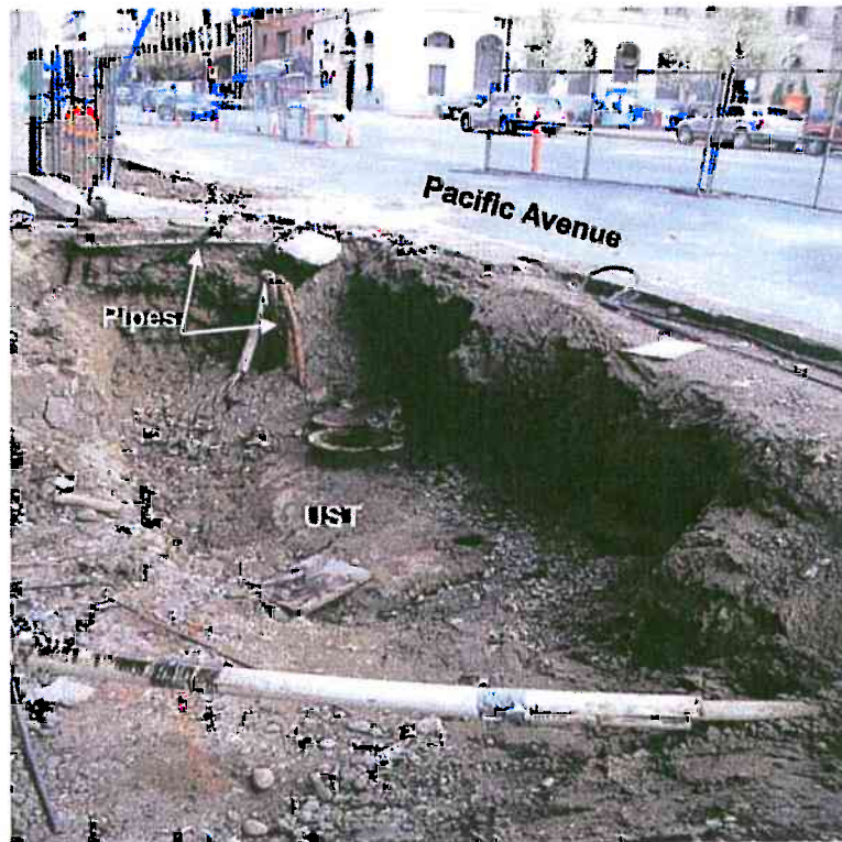
Top of UST exposed looking north. (April 10, 2008)
