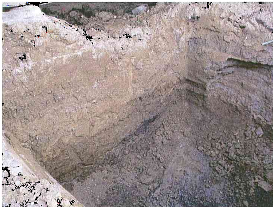
Final extent of excavation on west and northwest wall. (April 14, 2008)
