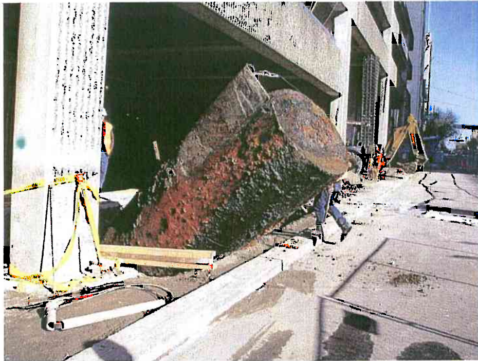
Underground storage tank during removal looking northwest. (April 11, 2008)
