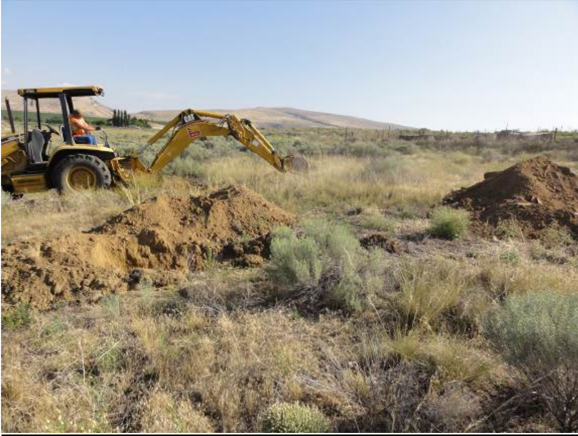
Backhoe digging TP29.
