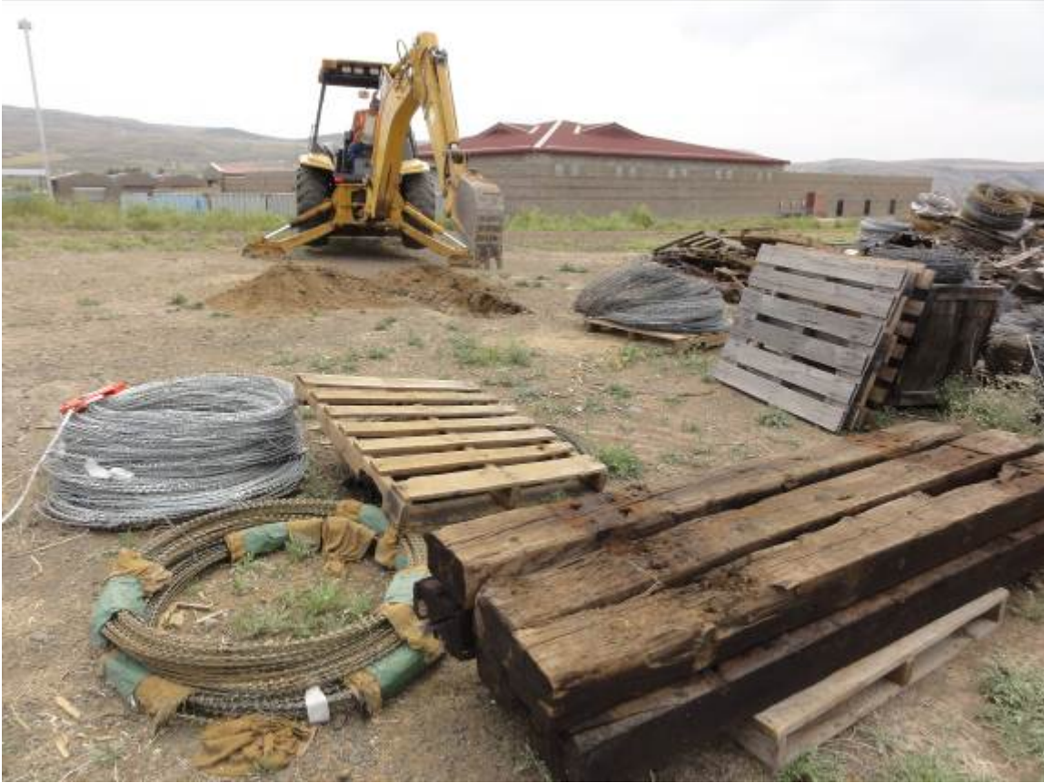
Backhoe digging TP 18. No garbage in TP18.
