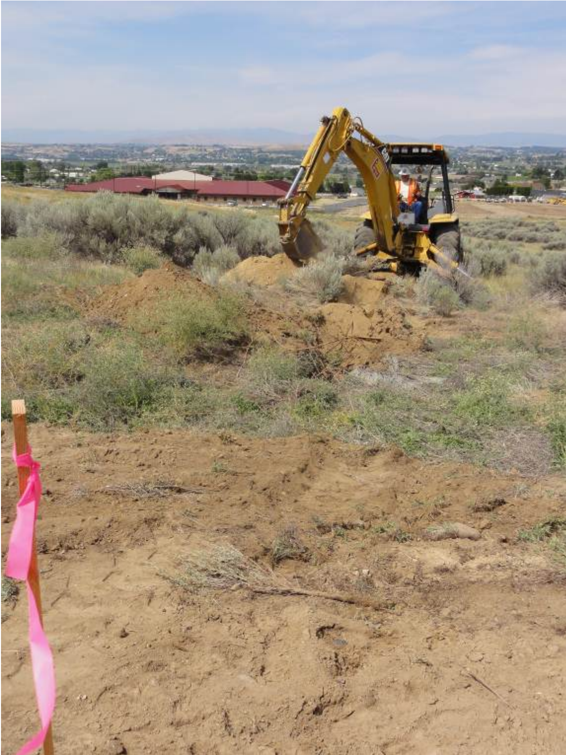
Backhoe digging TP10. No garbage in TP10.
