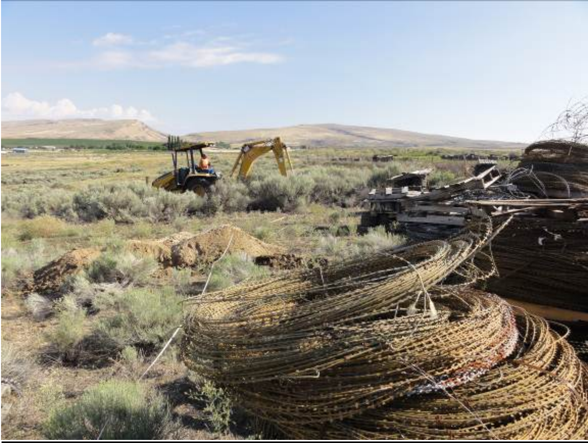
Backhoe digging TP31. No garbage in TP31.
