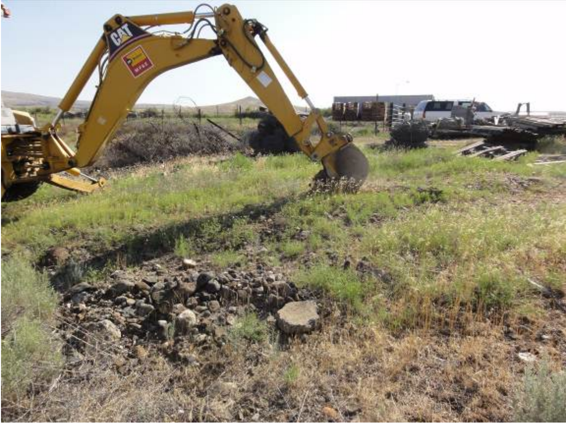
Backhoe digging TP32.
