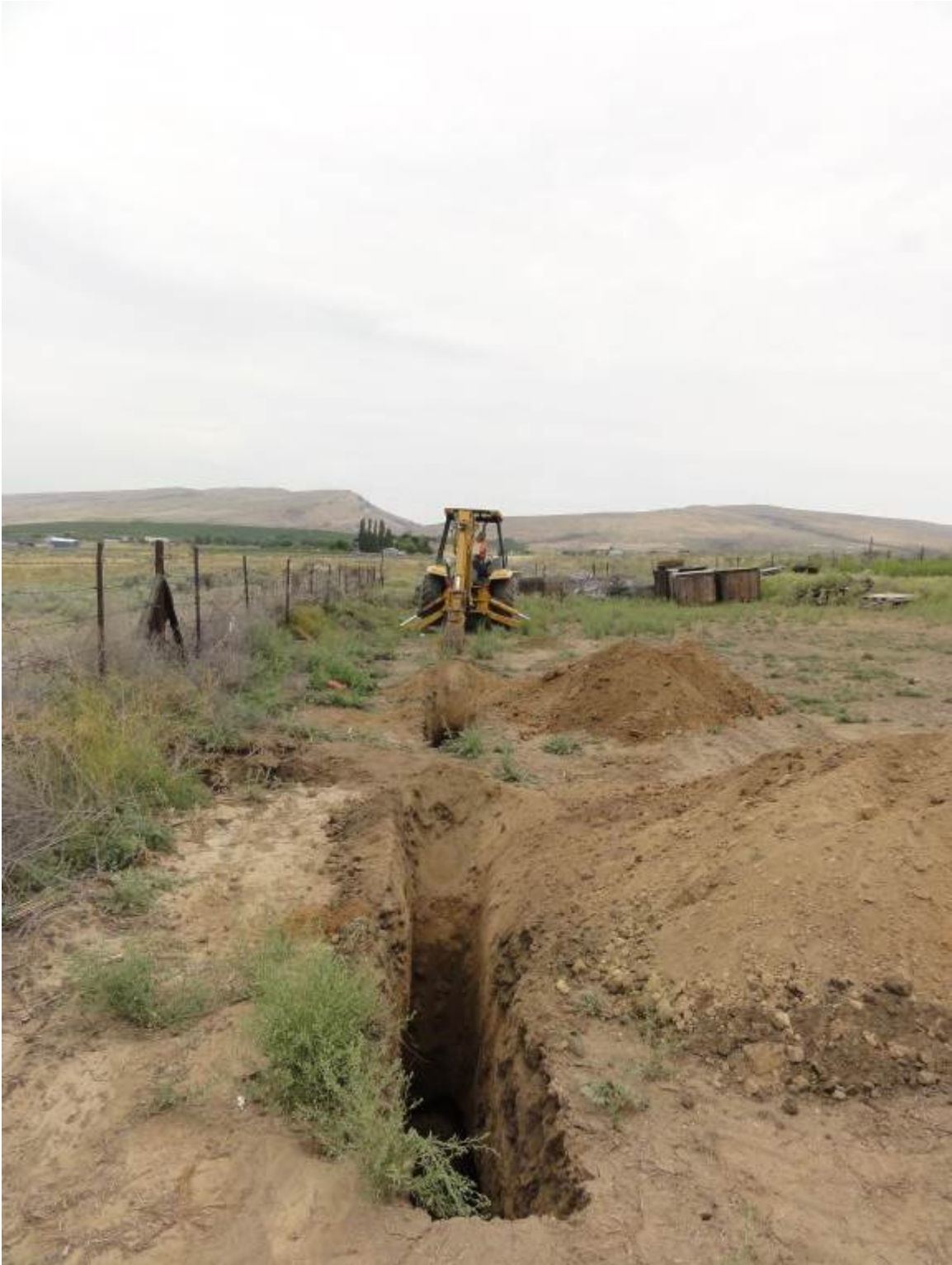
Backhoe digging TP24.
