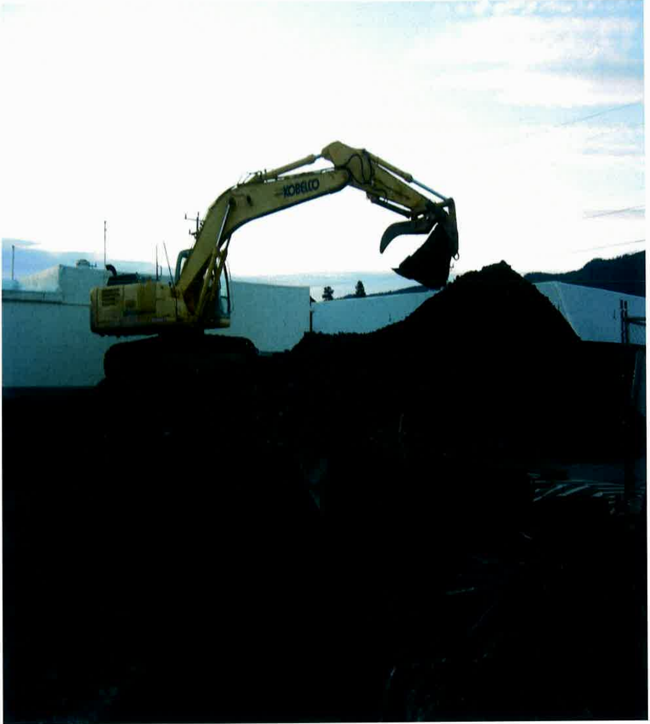
Ready for final "load-out" of contaminated soils on the next morning.
