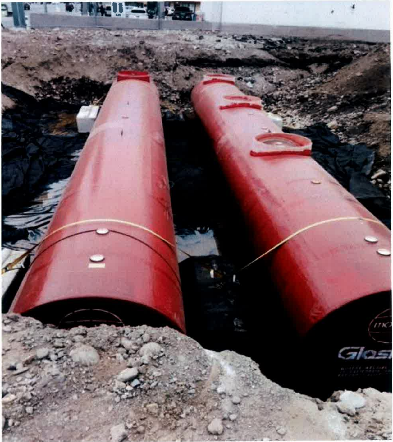
The two new USTs installed in the new Tank Pit.
