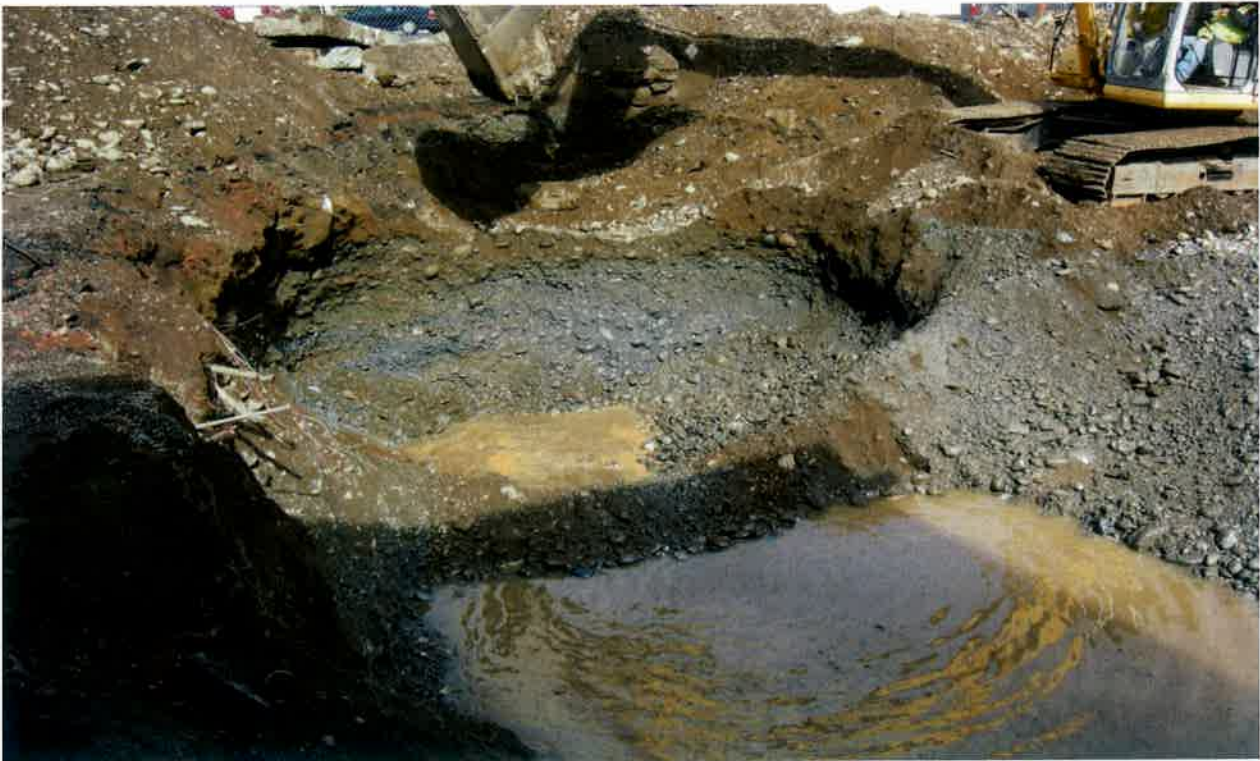
These photos are showing the Northwest end of the Pit, near and beyond where the location of the large "G1" Gasoline tank was located. Note that in the lower picture, the top of the contamination is four feet above the groundwater table, which may indicate that the groundwater table level has widely varied over the years.
