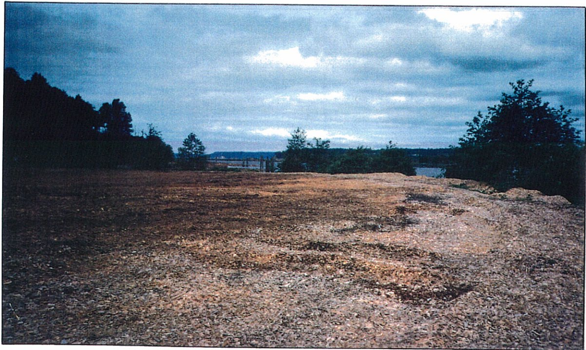
NO. 50 - CHIP PILE FILL, AREA 14
