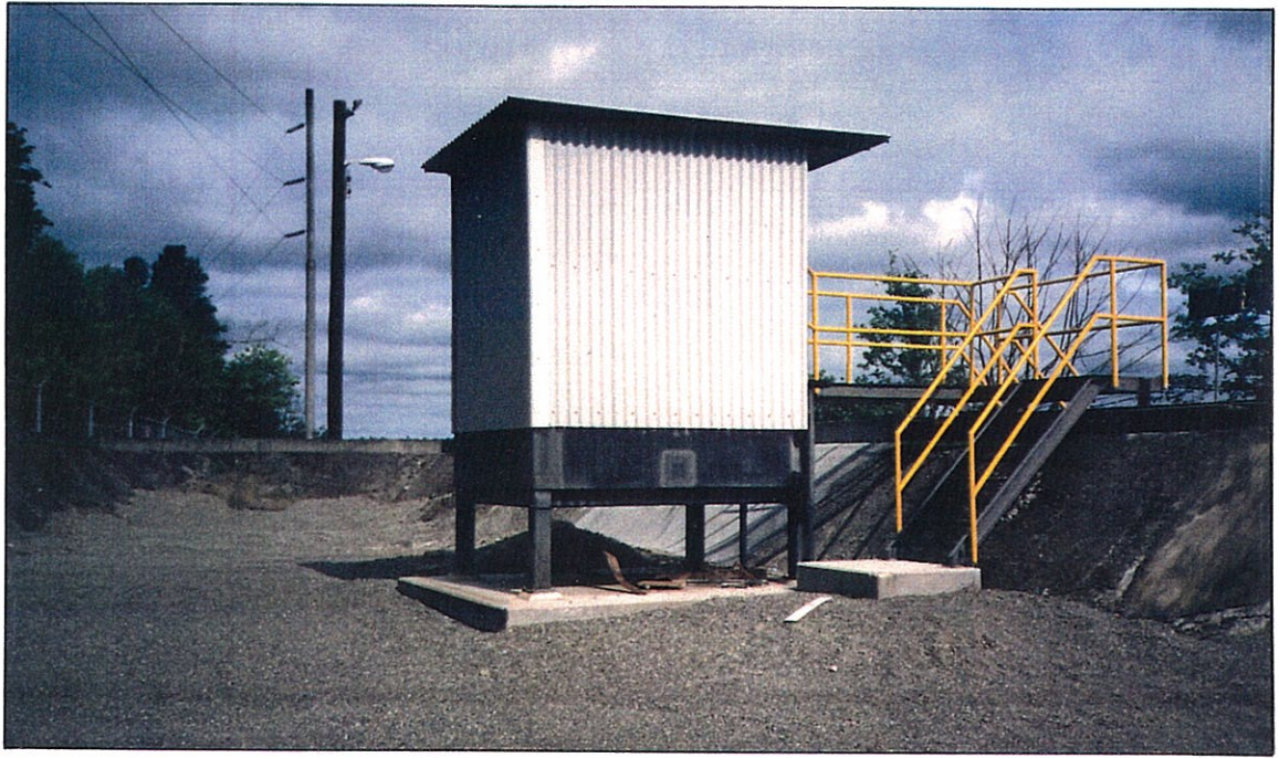
NO. 60 - DIESEL DISPENSER, AREA 15
