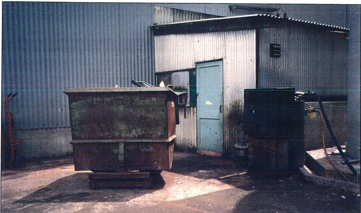
NO. 66 - OIL SHACK, AREA 16
