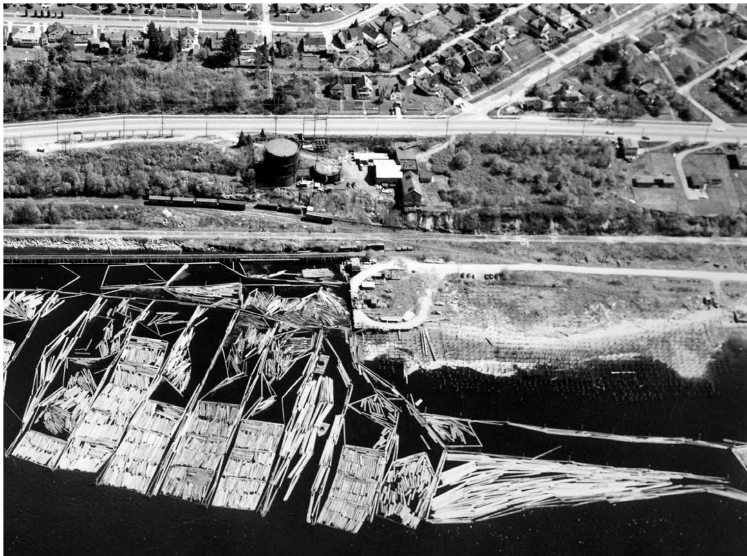
South State Street Manufactured Gas Plant Bellingham, Washington
