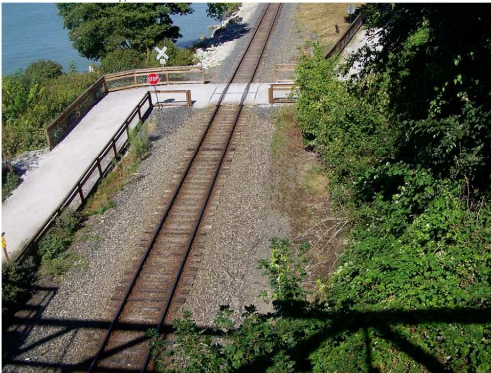
Railroad bed looking west.
