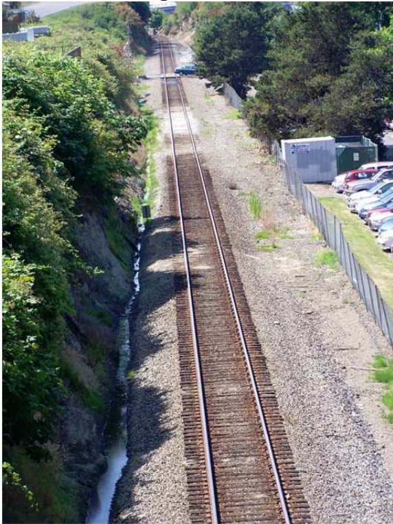
Railroad bed looking east.
