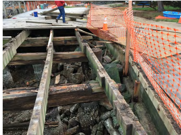
Hand removal of wharf wood
