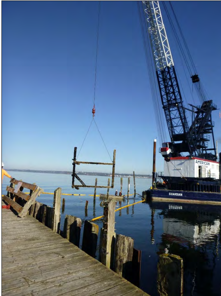
1. Removal of 12"x12" steel H-beams from superstructure.
