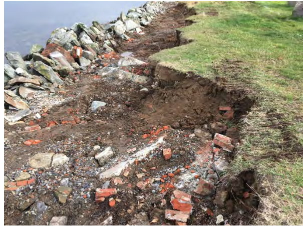
Supgrade before fabric was placed
