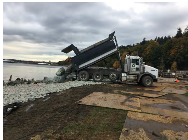
Drift sill tie in location before quarry spall placement.
