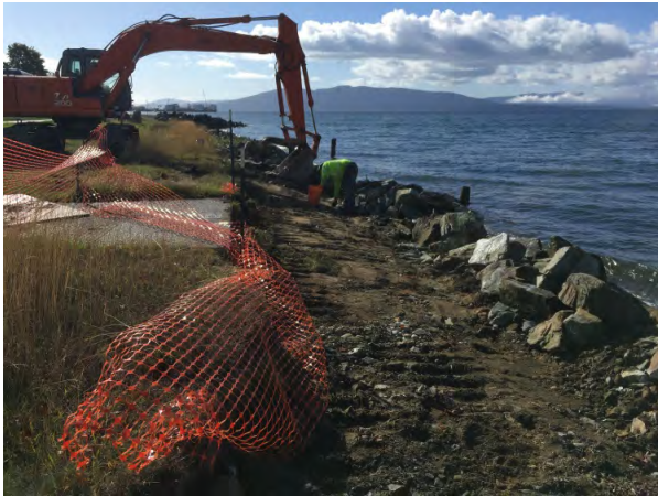
Subgrade prep near the concrete bench pad
