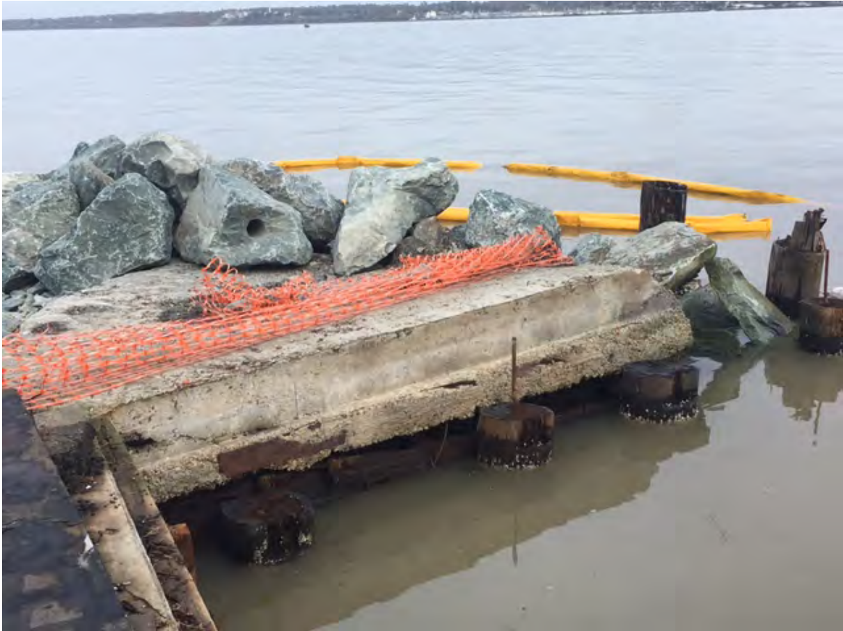
Figure 2. Ground photo of concrete apron taken today, 10/23/2017.
