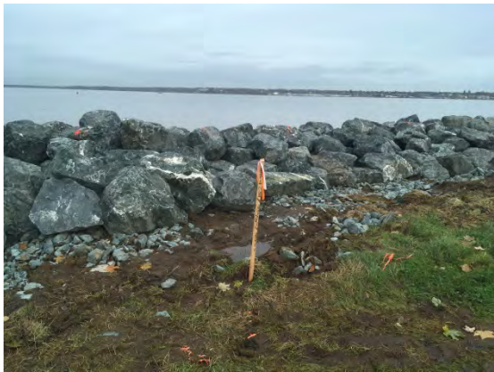
Orange dots showing exact 13.5' crest elevation to the right of this stake, and 14' to the left and grade line.
