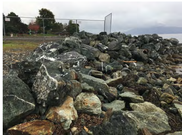
Drift sill tie in location before quarry spall placement.
