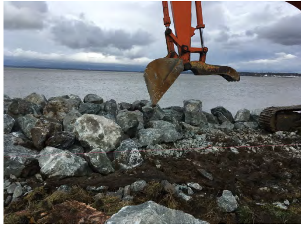
Directing armor stone placement
