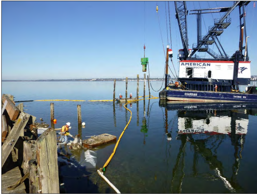
5. Looking north at creosote piles being loosened for extraction.
