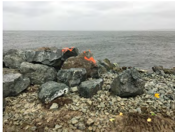
Orange marked rock to show placement going north.
