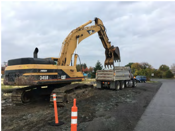
Armor stone from stockpile
