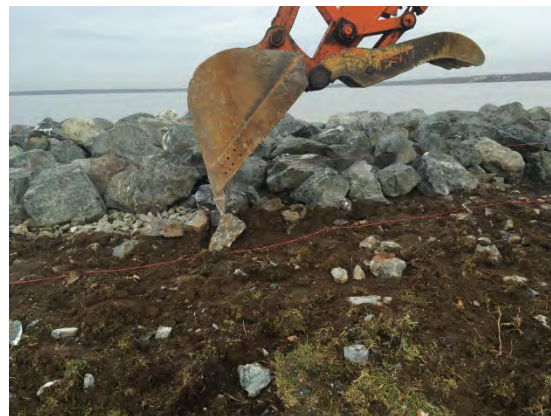
Armor stone direction (directed to move a rock to touch adjacent stones). Rick states this type of direction will be available for final walkthrough on entire armor stone berm.
