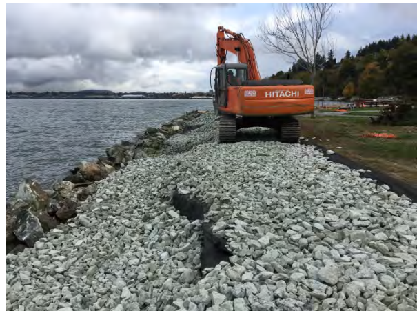
Fabric placement and quarry spall before grading
