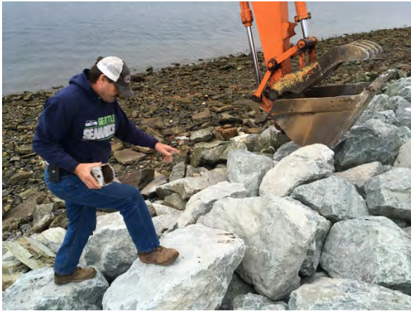
Quarry spall used as haul road.
