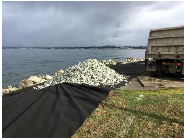
Fabric placement and quarry spall before grading
