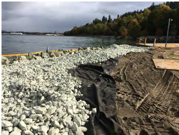
Subgrade before fabric was placed
