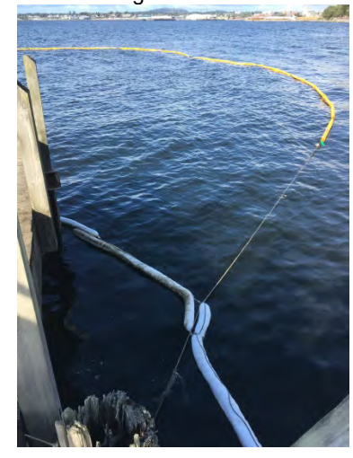
Boom connection to shore, east of wharf.
