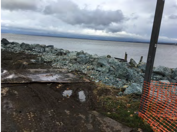
Location of profile H where 13.5 ' MLLW elevation crest width will be re-evaluated once contractor placing rock until Profile H
