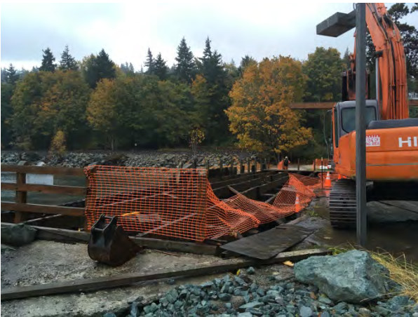
Equipment removal of wharf
