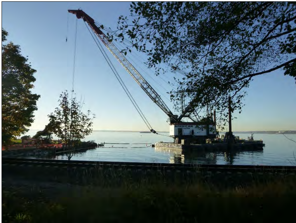
10. Piles removed and buoys in place for sand drop locations.
