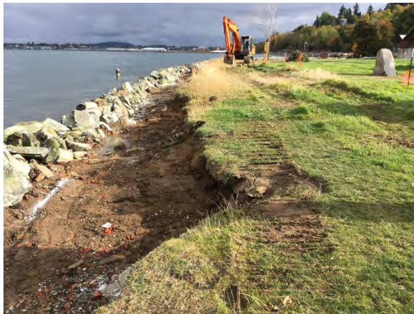
Subgrade before fabric was placed
