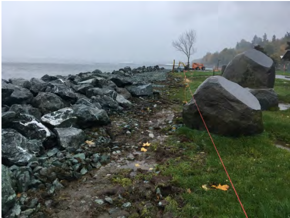
Grade line and Syper quarry rock
