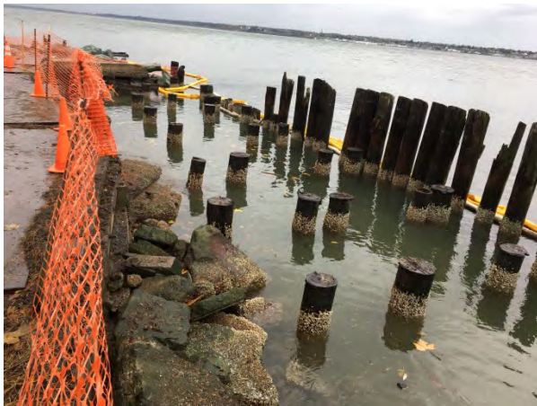
Removed wharf and shoreline condition
