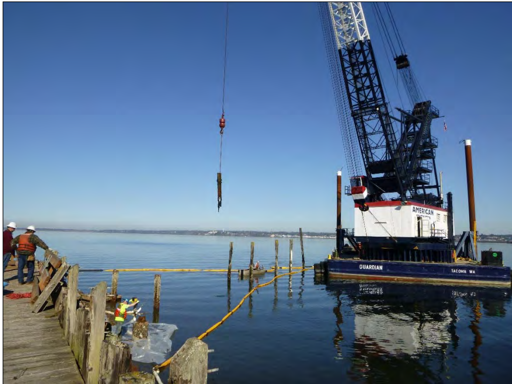
3. Looking north at first H-pile removal.
