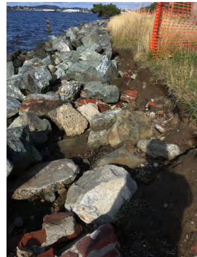
Shore conditions looking north
