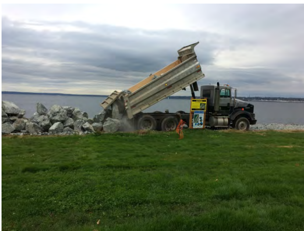
Rock delivery using quarry spall as haul road
