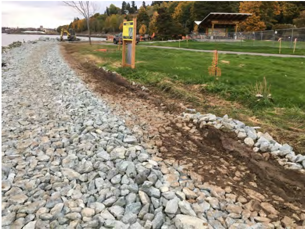
Quarry spall used as haul road.
