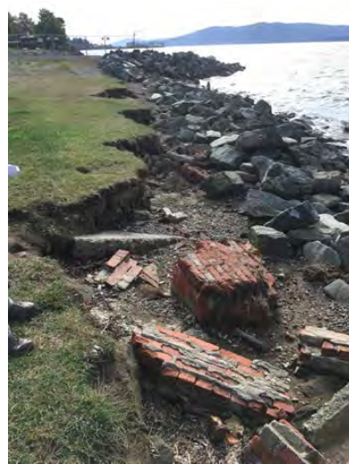
Shore conditions near drift sill of pocket beach
