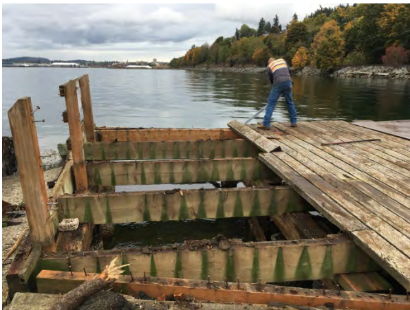
Hand demolition of wharf
