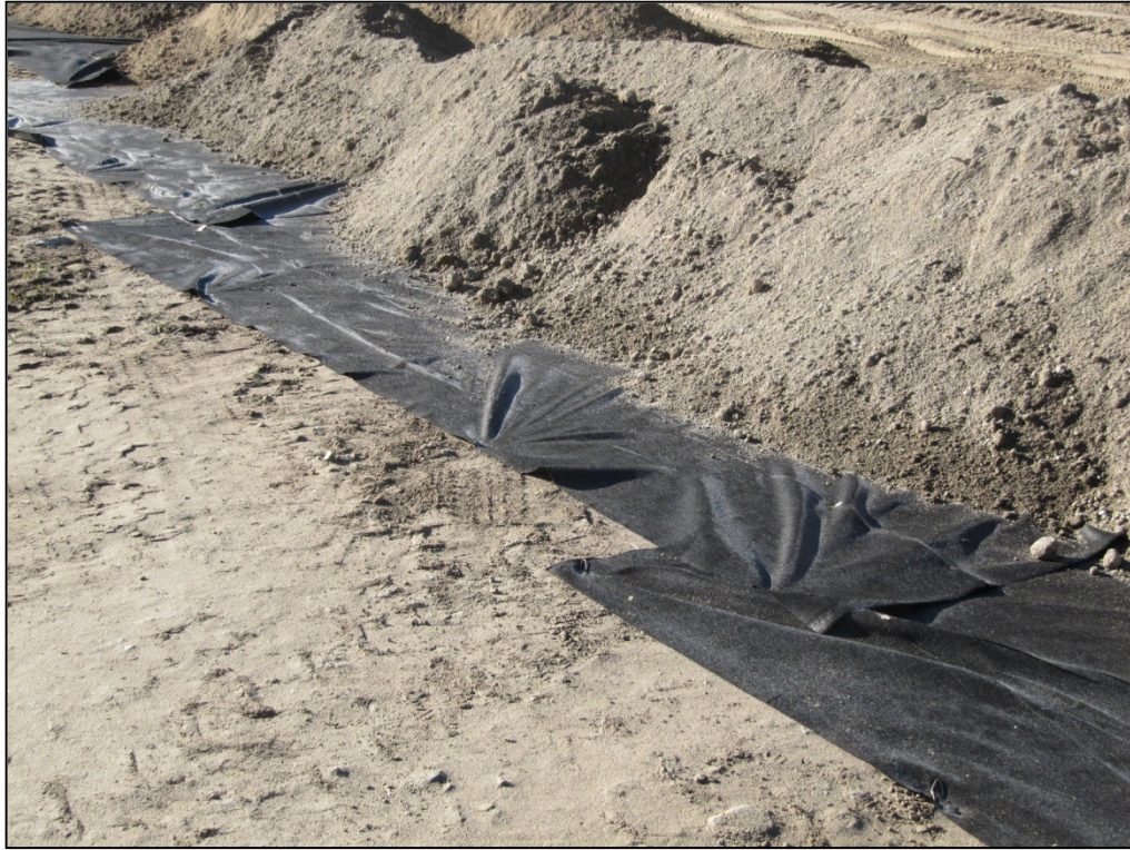
3. Overlapping geotextile fabric.
