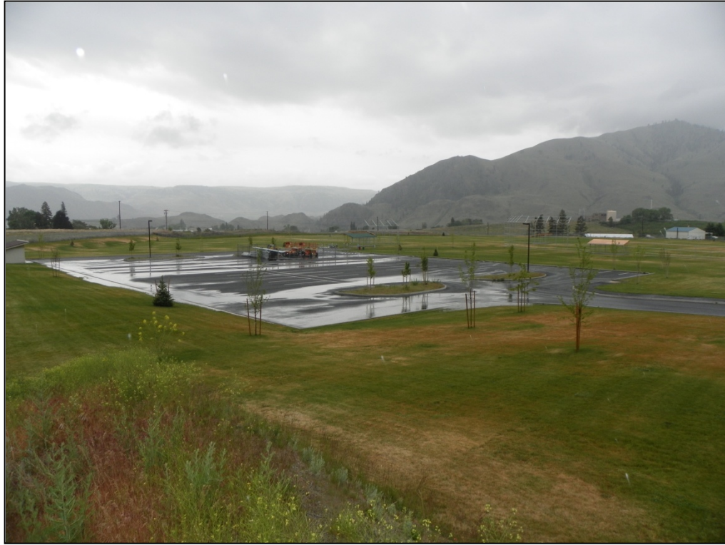
5. Completed remediation and site improvements in the South Fields area.
