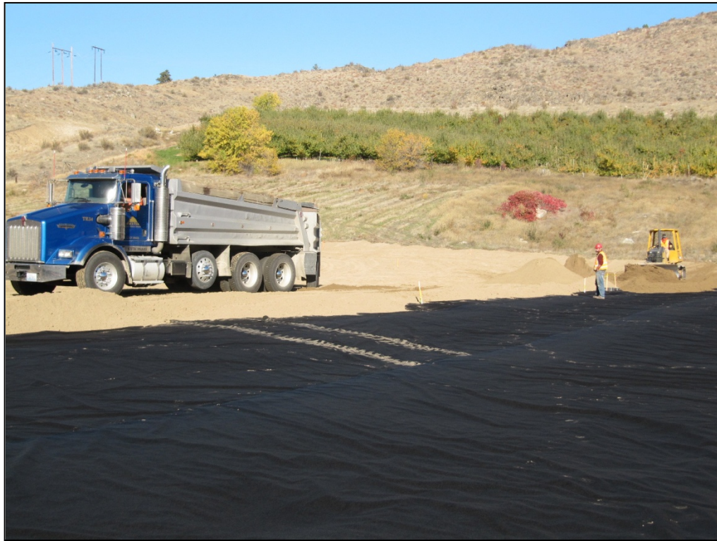
4. Placing clean fill material on the North Fields area.
