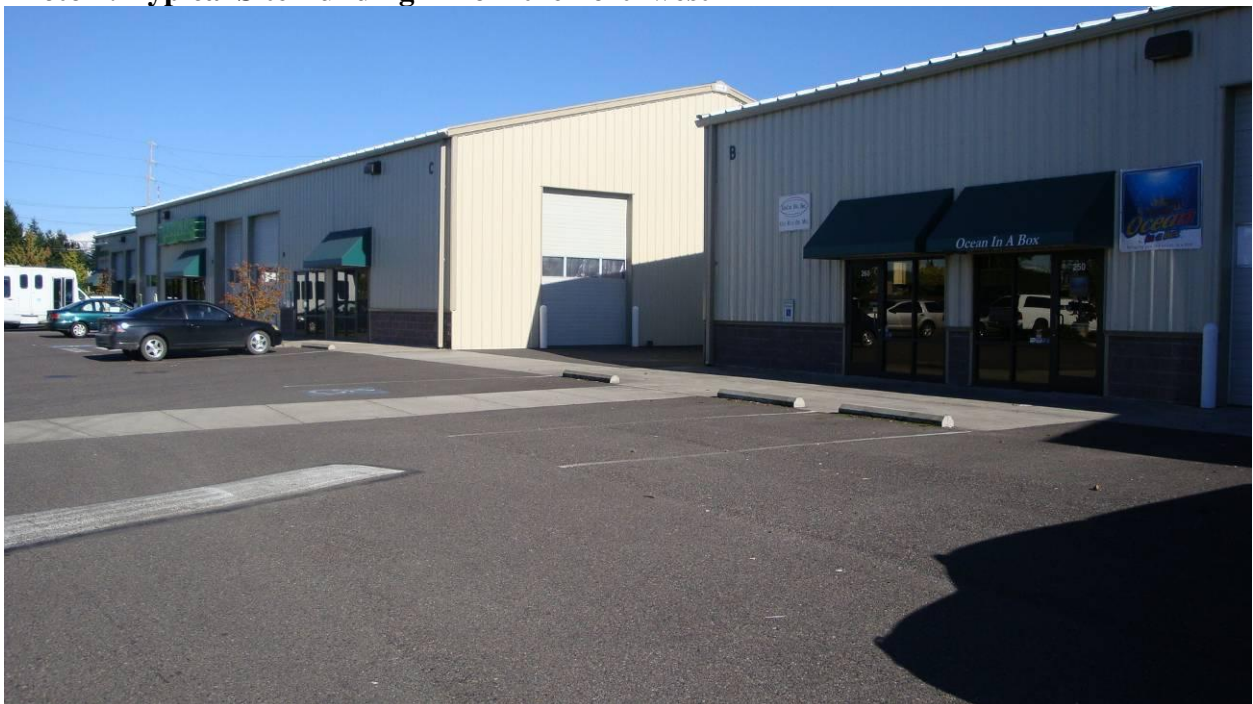
Photo 2: Typical Site Building – from the northwest
