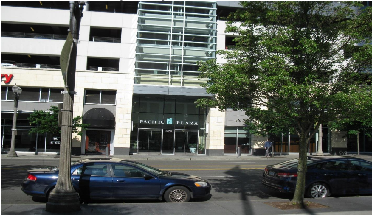
Photo 1: Pacific Plaza Garage Building – from the North
