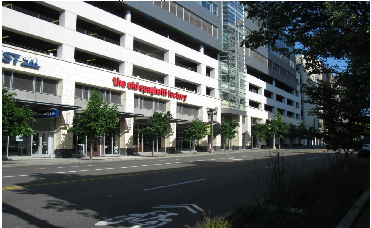
Photo 2: Pacific Plaza Garage Building– from the Southwest
