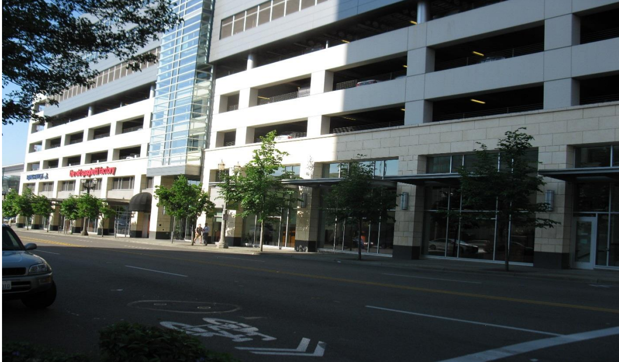
Photo 3: Pacific Plaza Garage Building – from the Northeast
