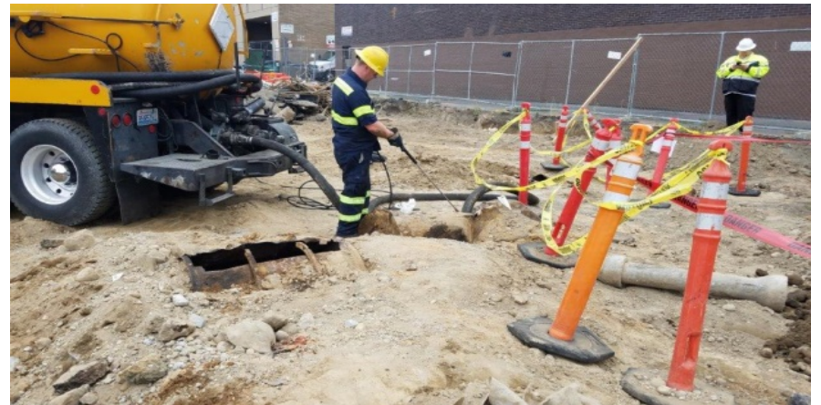
Photo 4: Triple Rinsing USTs
