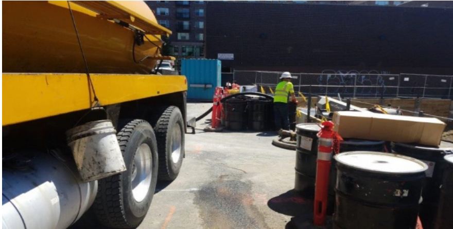
Photo 5: Drumming Product and Wash Water
