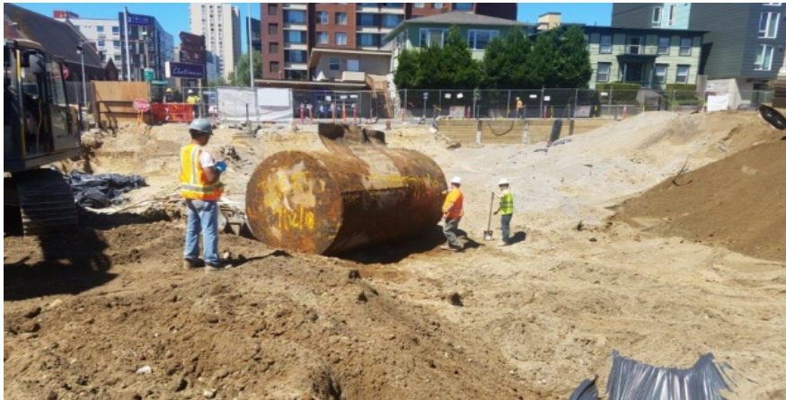
Photo 7: Labeling UST 7 Prior to Transport
