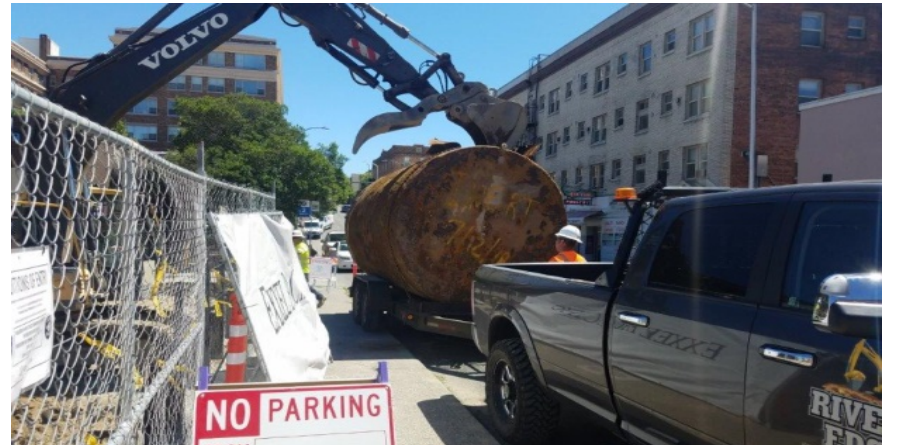
Photo 8: Loading UST 7 for Transport
