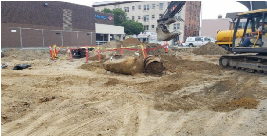
Photo 5: USTs 2 and 3 Removed
