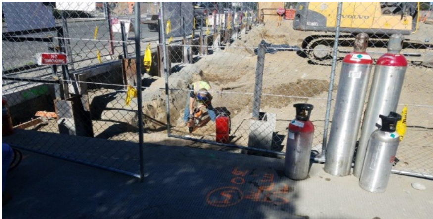
Photo 3: Cutting UST 8 for Cleaning
