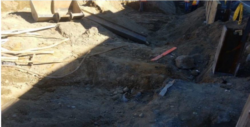
Photo 1: Top of UST 7
