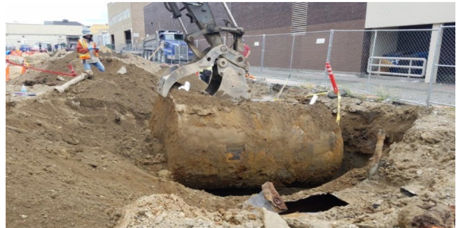
Photo 8: Removal of UST 4
