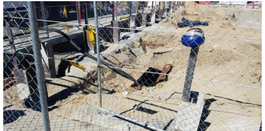
Photo 4: Pumping Residual Product from UST 8
