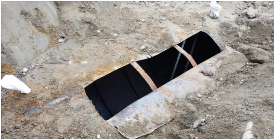
Photo 3: Top of UST 4
