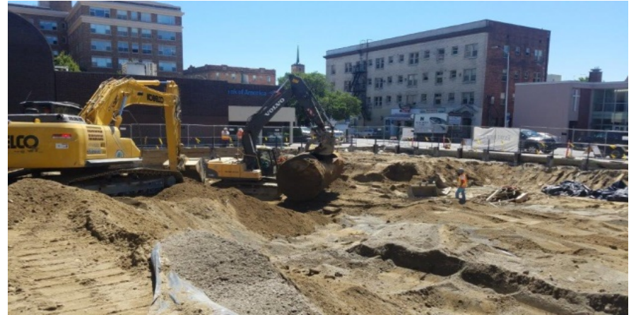
Photo 6: Removal of UST 7
