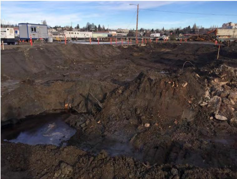
Photograph 4. Overburden removed, contaminated material encountered.
