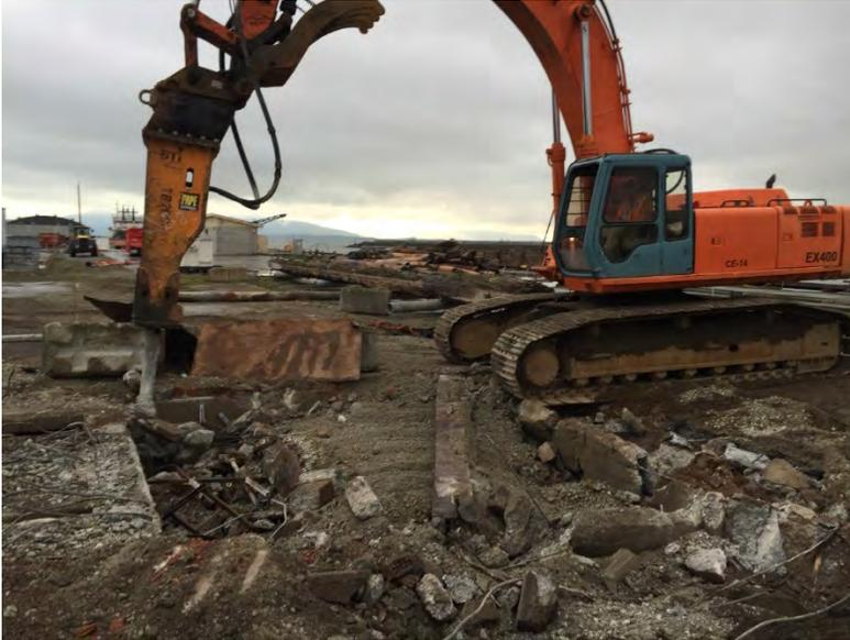
Photograph 1. Removal of surface slab and foundation elements.
