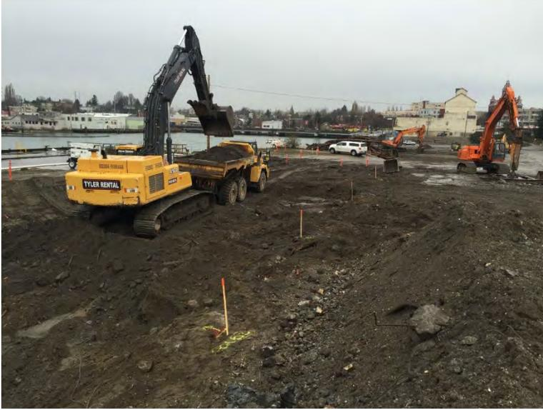
Photograph 3. Loading out of overburden to stockpile area.
