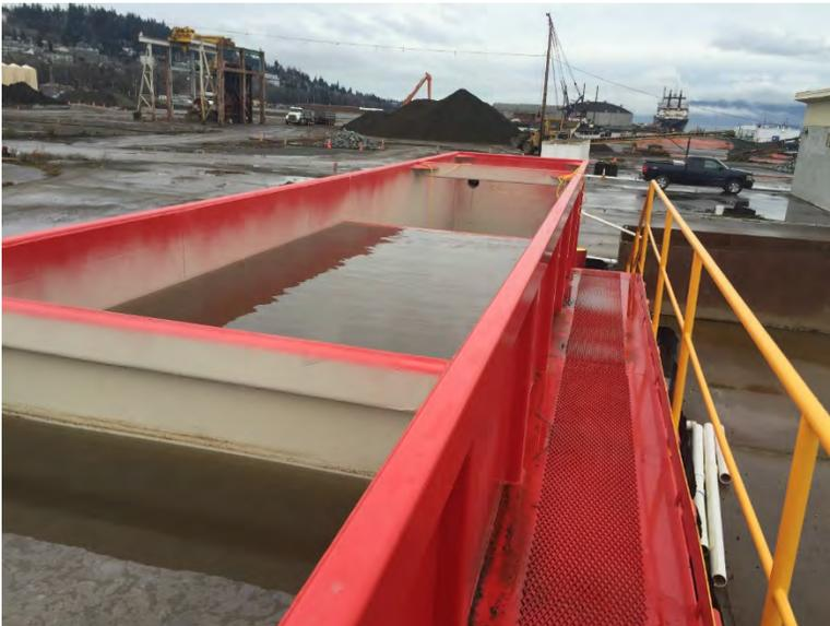
Photograph 6. Weir tank as part of water treatment system.
