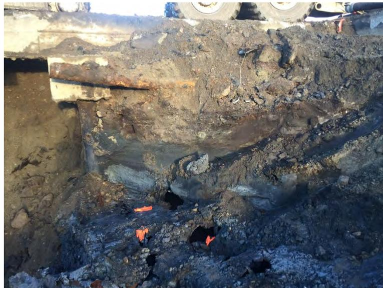
Photograph 10. Excavating contaminated material at bulkhead in NE corner of excavation. Orange flags mark locations of pipes that pierced bulkhead. No evidence of petroleum in pipes. Pipes were cut and capped.
