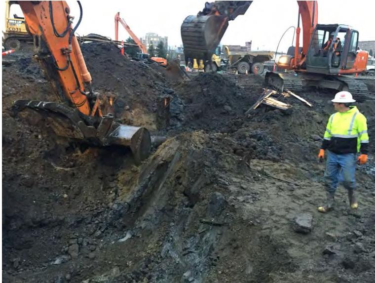
Photograph 7. Excavating contaminated material.
