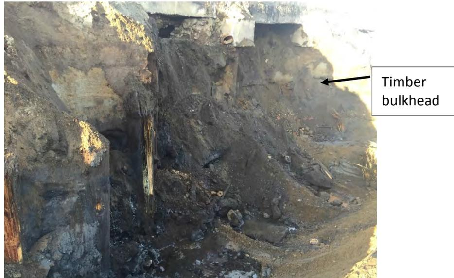
Photograph 9. Excavating contaminated material at bulkhead in NE corner of excavation.
