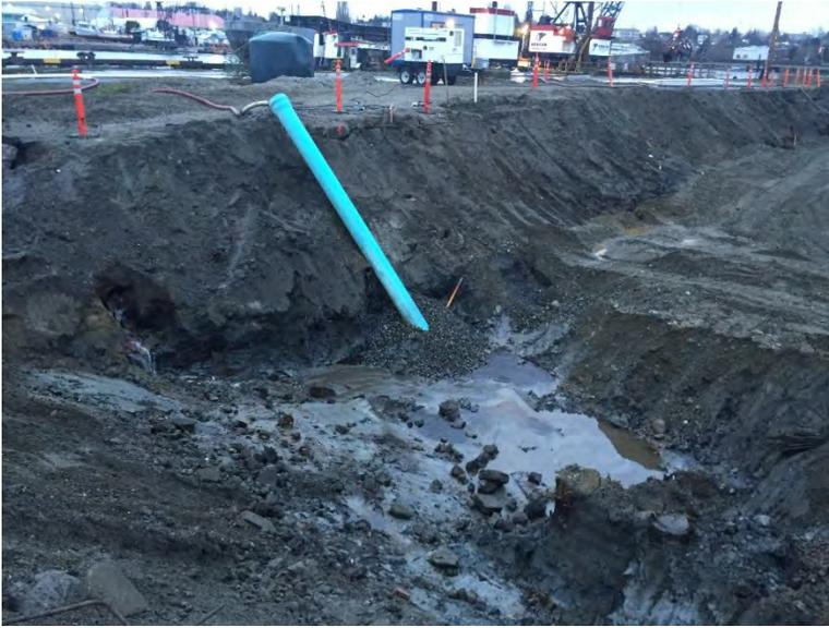
Photograph 5. Dewatering sump in operation.
