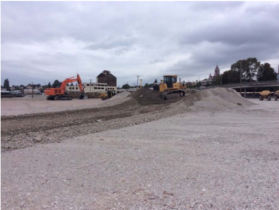
Photo 8. Re-grading Recycled Concrete Aggregate.
