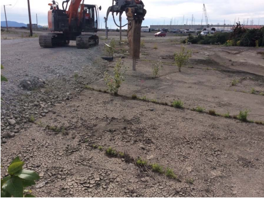
Photo 5. Perforating degraded pavement to facilitate infiltration.
