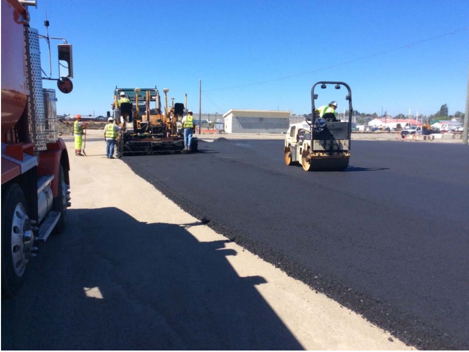
Photo 13. Constructing asphalt pavement hard cap.
