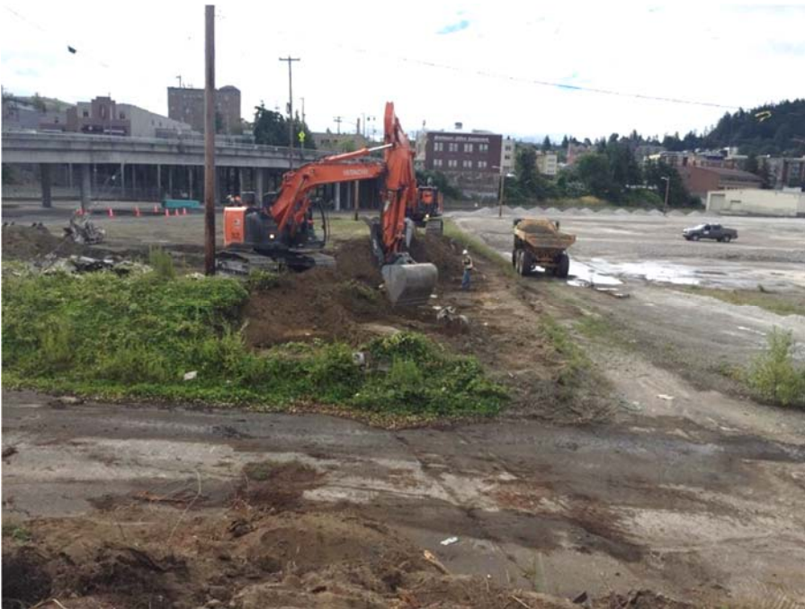
Photo 2. Excavation of knolls.
