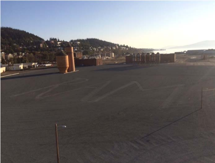
Photo 14. The completed cap, looking mill-west from Chestnut Avenue.
