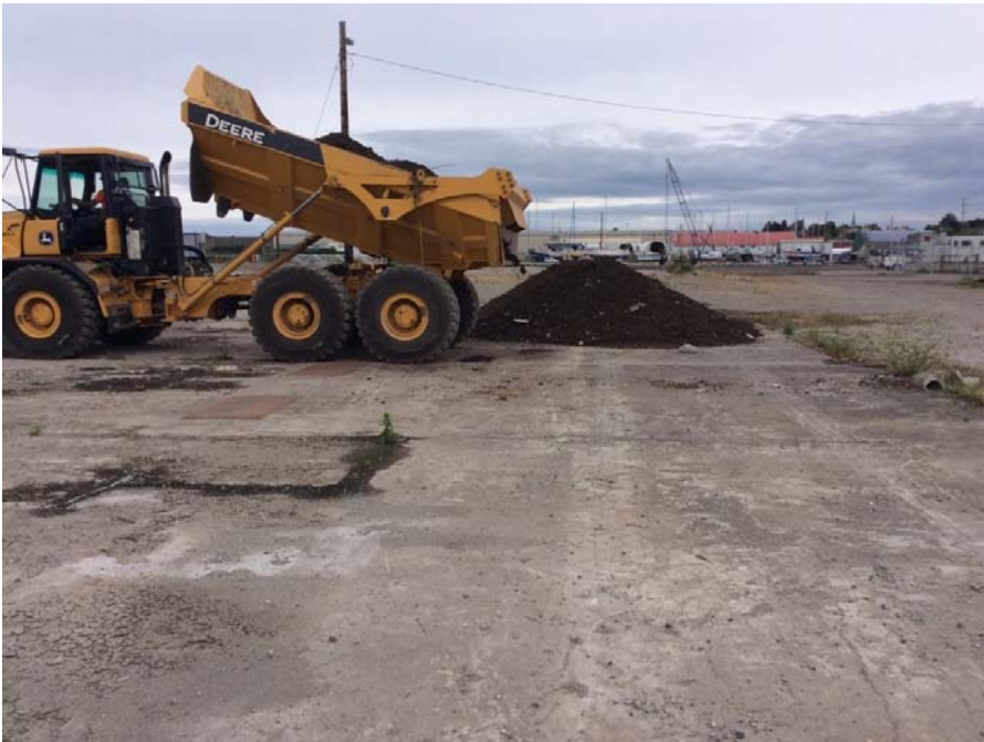
Photo 4. Placing removed veneer in above-grade fill area.
