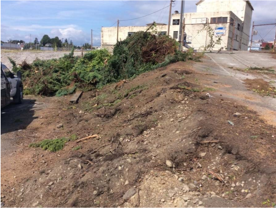
Photo 1. Clearing and grubbing before excavation of knolls.
