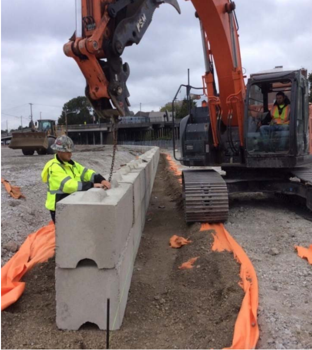
Photo 9. Constructing gravity block wall along southeast edge of above-grade fill area.
