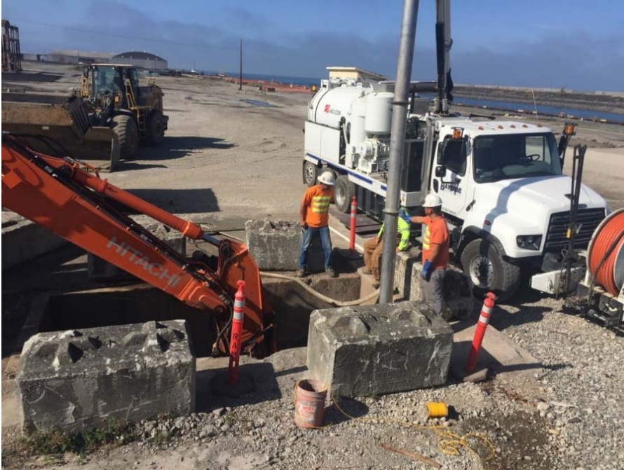
Photo 7. Cleaning out subsurface structures.
