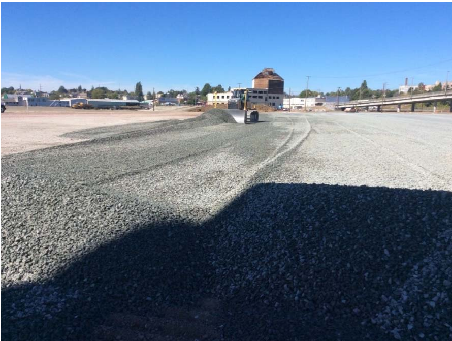
Photo 12. Placing permeable ballast.
