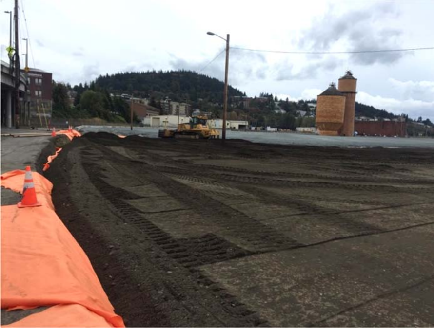
Photo 11. Grading of gravel borrow over separation geotextile.
