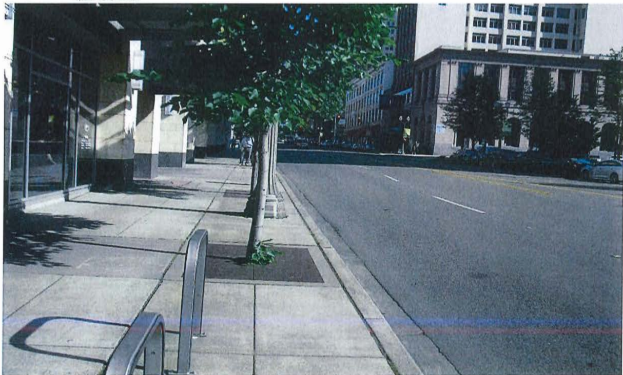
Photo 6: Soil Contamination Left-in-Place below the Sidewalk and Pacific Avenue – from the South
