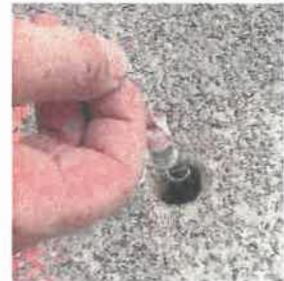
WMS™ Sampler being deployed for sub-slab gas sampling
