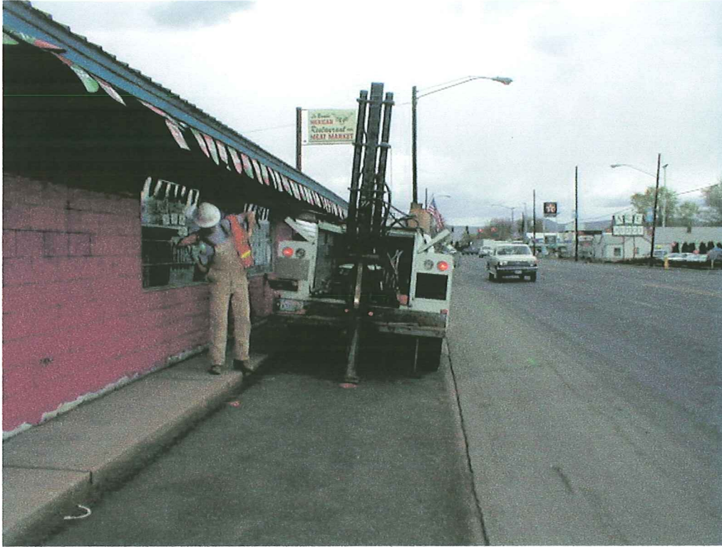
PHOTO 5: BORING #4 NEAR EAST PROPERTY BOUNDARY
