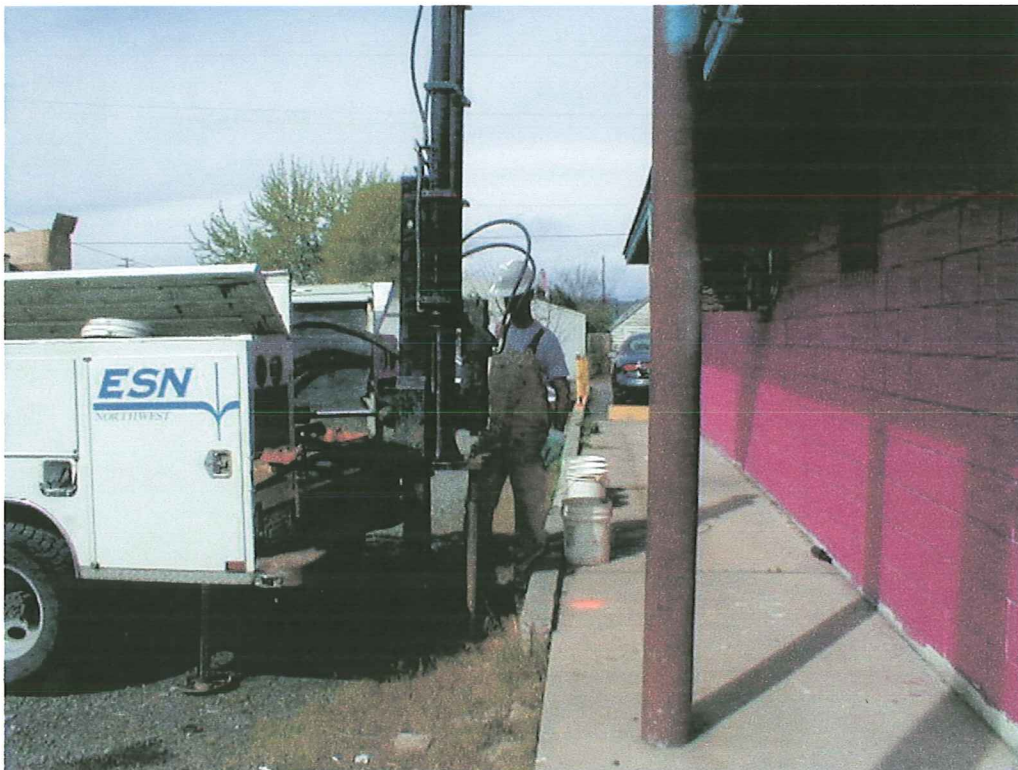
PHOTO 2: LOOKING WEST, BORING #1
