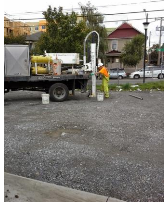
Photo #2: Boring B-6 being advanced. Photo looking east.
