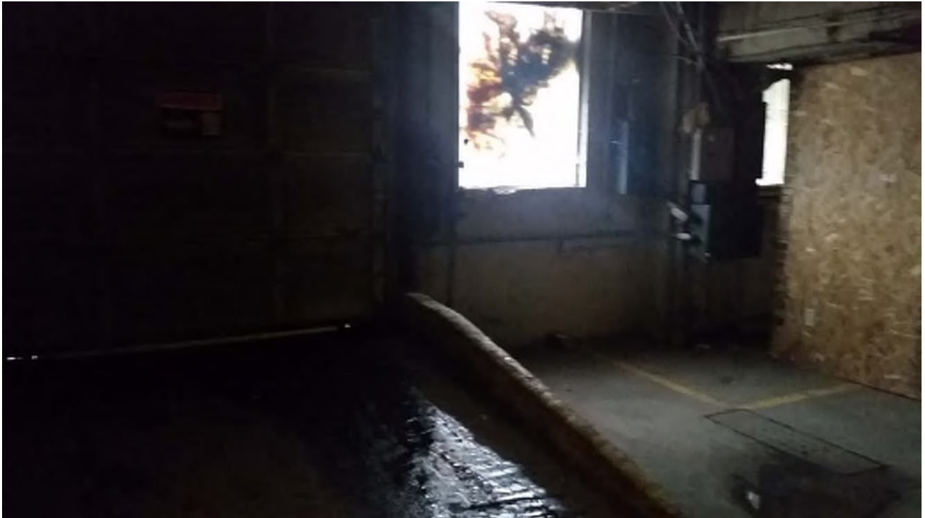
Photograph 5: Bay door with ramp into first floor.
