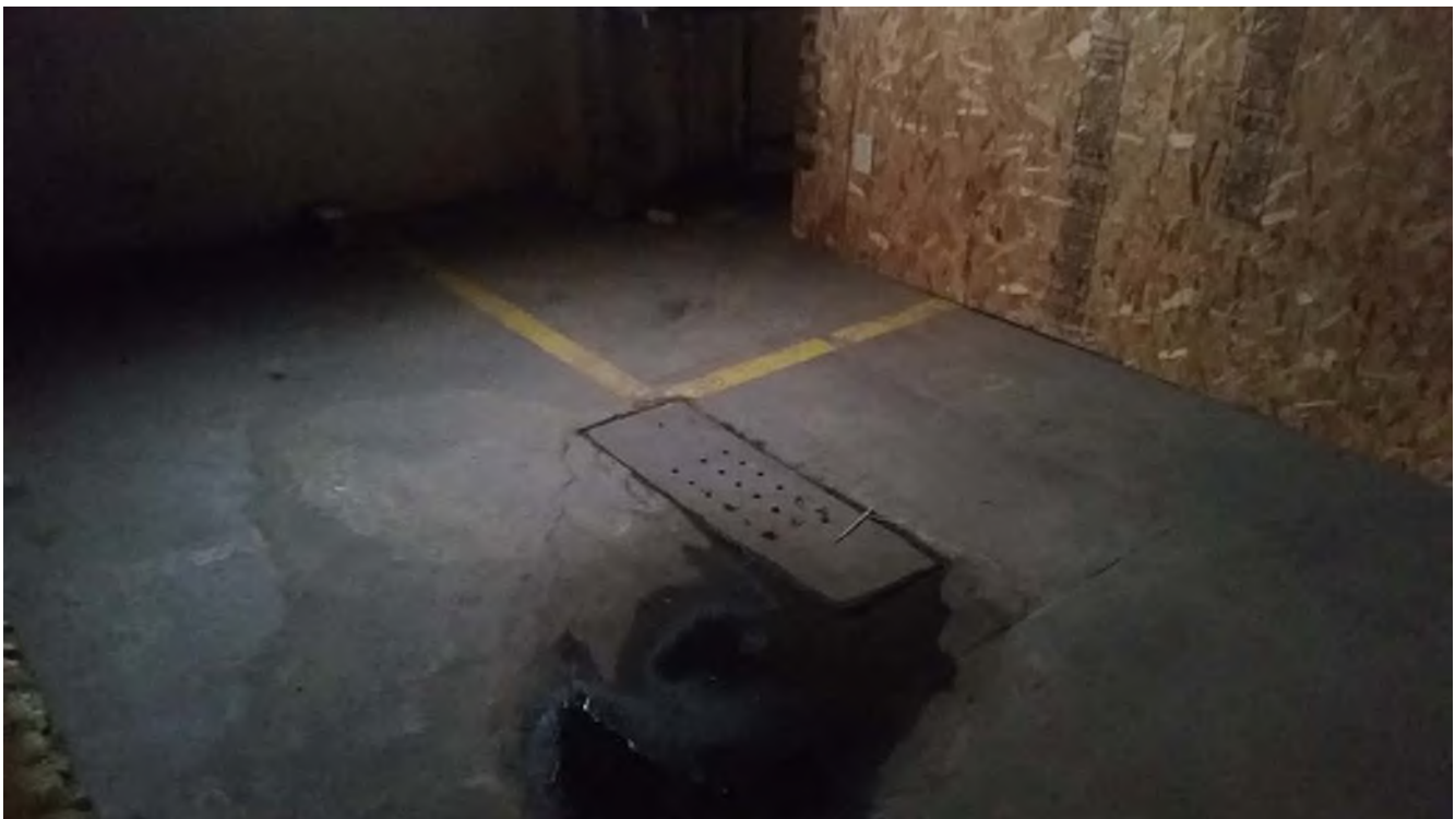
Photograph 4: Drain on first floor.
