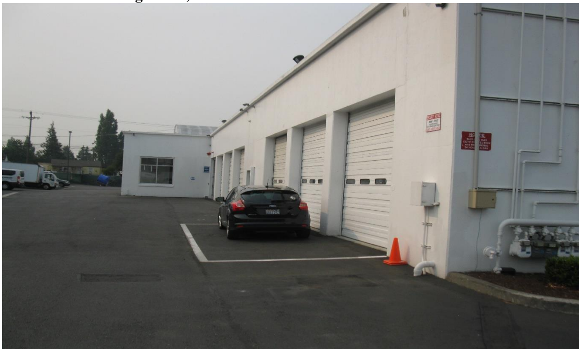
Photo 5: Western Back Side of the Current Self-Storage Building (Former Pierce Transit Maintenance Building): Asphalt Cap on the Contaminated Soil Left-in-place (in Front of the First Three Rolling Doors)—From the Northeast
