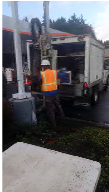
View of Direct Push Rig advancing B3
