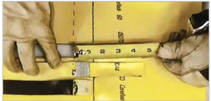
STEP 4. Weld width verification
