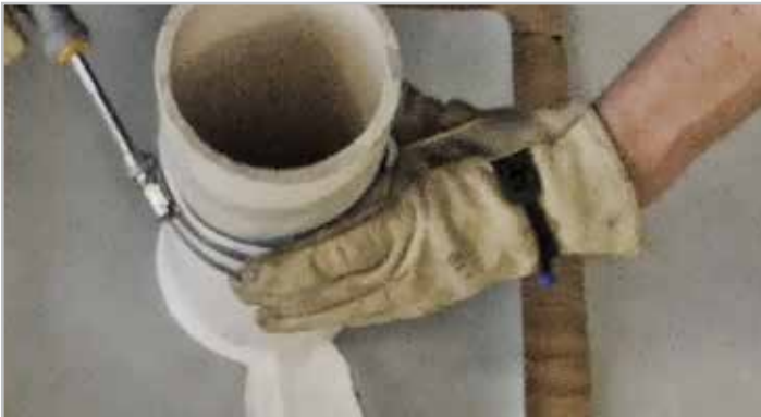
STEP 7. Install second hose clamp
