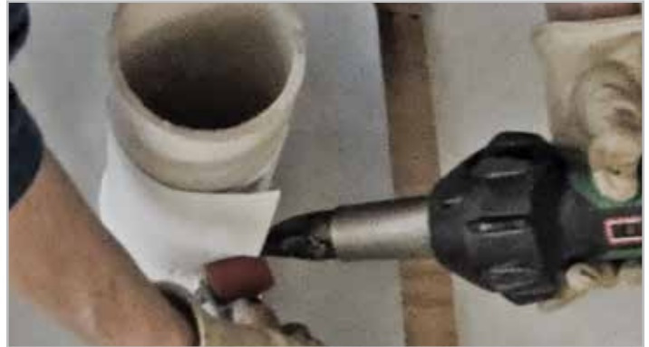
STEP 4. Weld vertical overlap seam up stack
