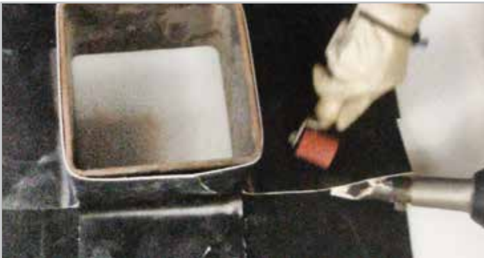
STEP 4. Weld target patch in place
