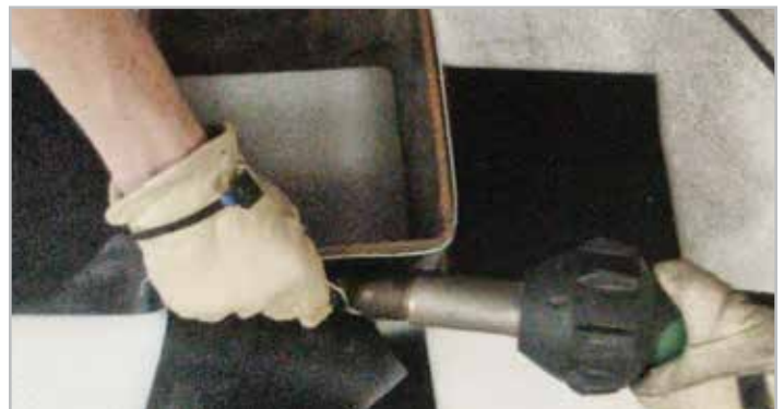
STEP 2. Target flashing tack weld
