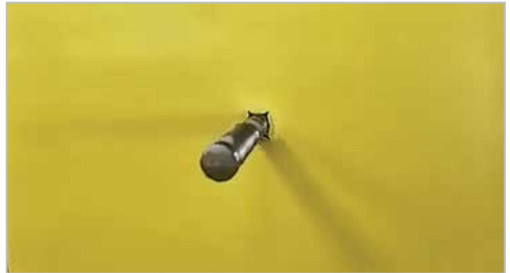
STEP 1. Install COREFLASH target piece
