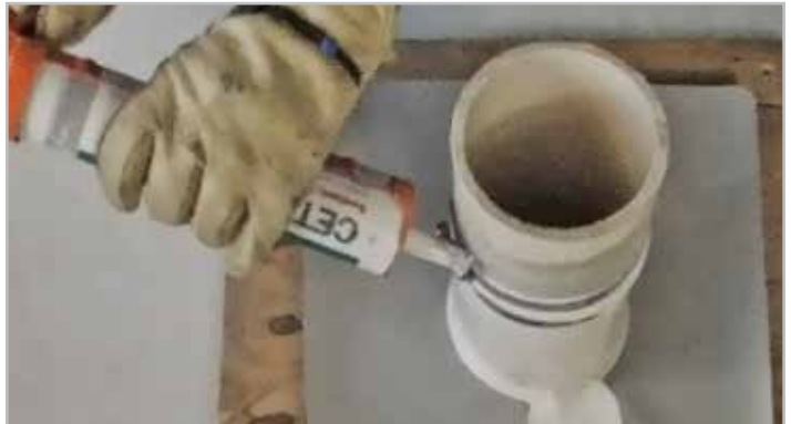
STEP 9. Apply CETSEAL bead at termination
