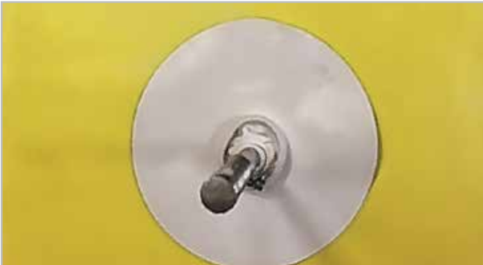
STEP 8. Tightly secure hose clamp
