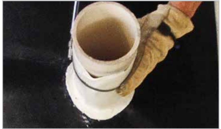
STEP 6. Install lower clamp
