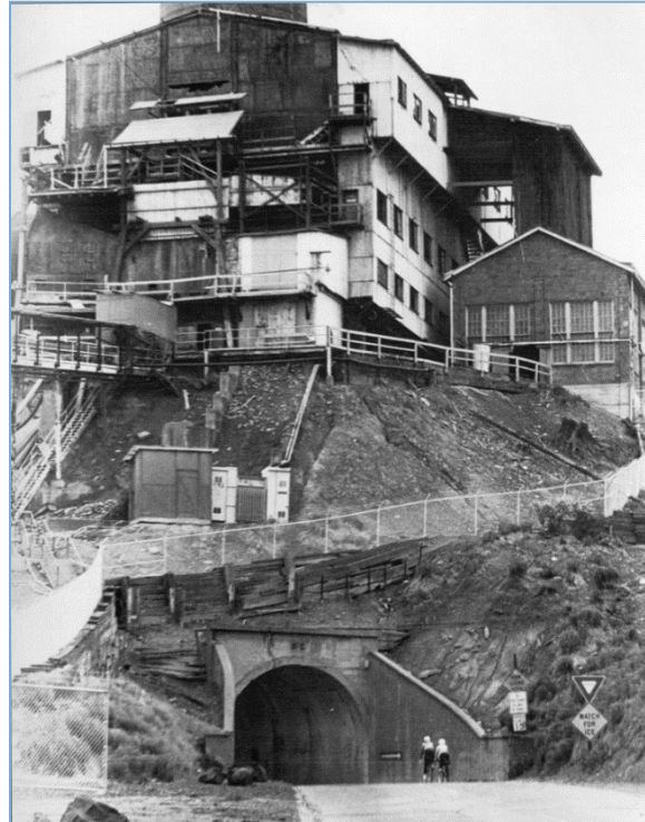
Photo 15:- Ruston Tunnel under the former Asarco plant. Photo courtesy of Sherri Forch.
