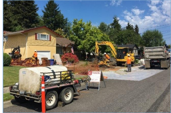
Photo 4: A contractor excavates contaminated soil from a yard in Tacoma
