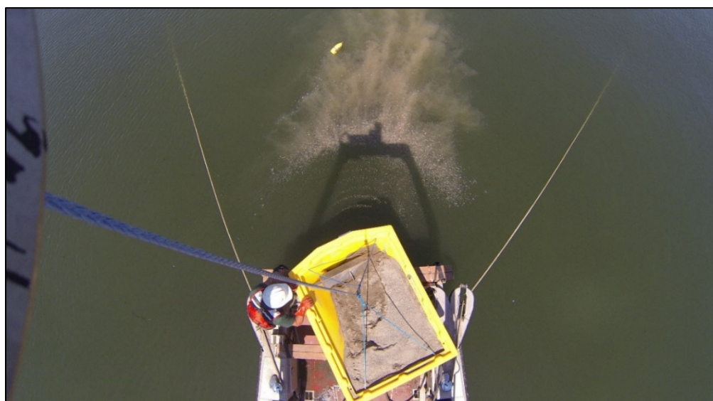
Photograph 1 – Application of capping material
