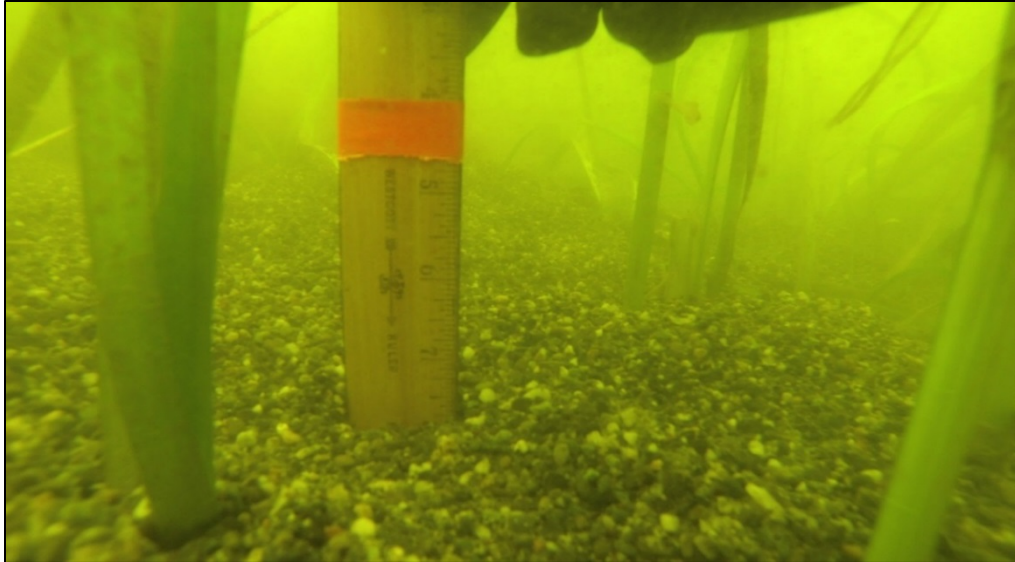
Photograph 2 – Assessment of deployed cap material at 4-inch test plot
