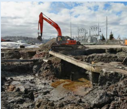
Figure 2 - K-C Site in 2013 during interim cleanup work
