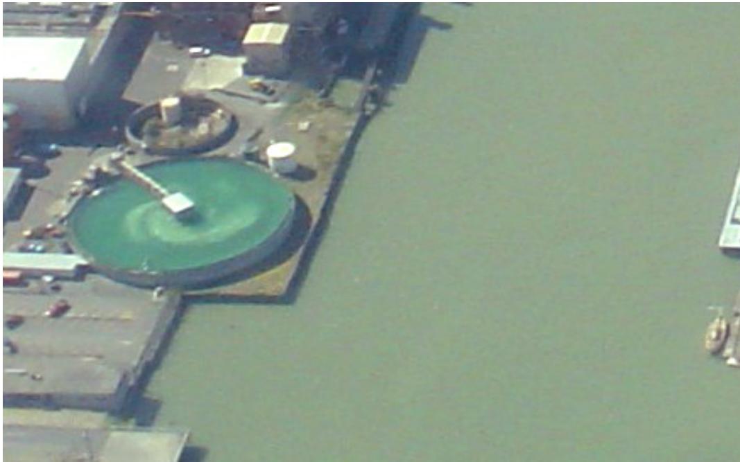
Before Construction: The South Shoreline consisted of a vertical bulkhead and fill area occupied by the abandoned clarifier structure. Numerous creosote-treated timber dolphins and unused structures were present.
