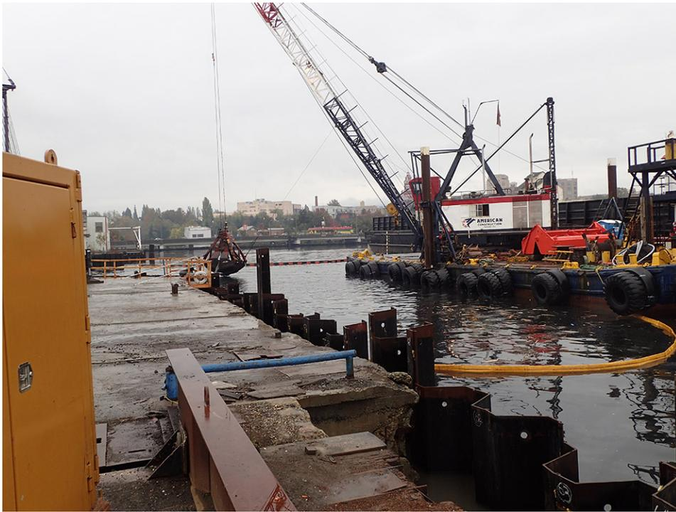
**Photograph 29: Inner Waterway dredging operations; debris booms deployed. Facing east.**
