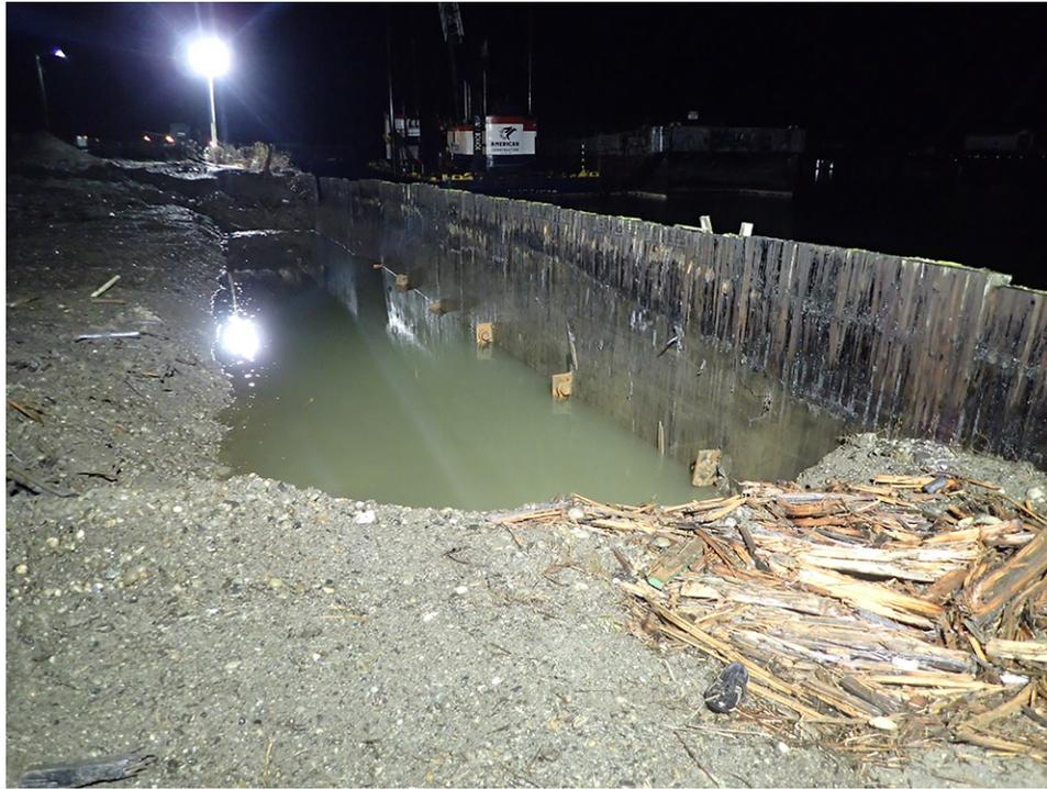
**Photograph 3: South shoreline during removal of the steel sheetpile bulkhead. Facing west.**
