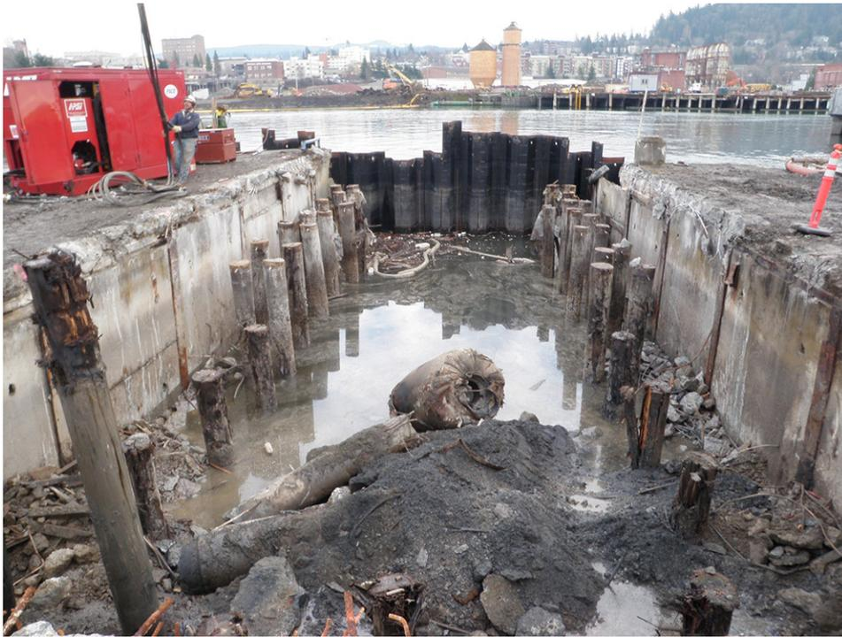
**Photograph 39: Central Waterfront barge ramp demolition at the Maple Street Bulkhead. Facing south.**
