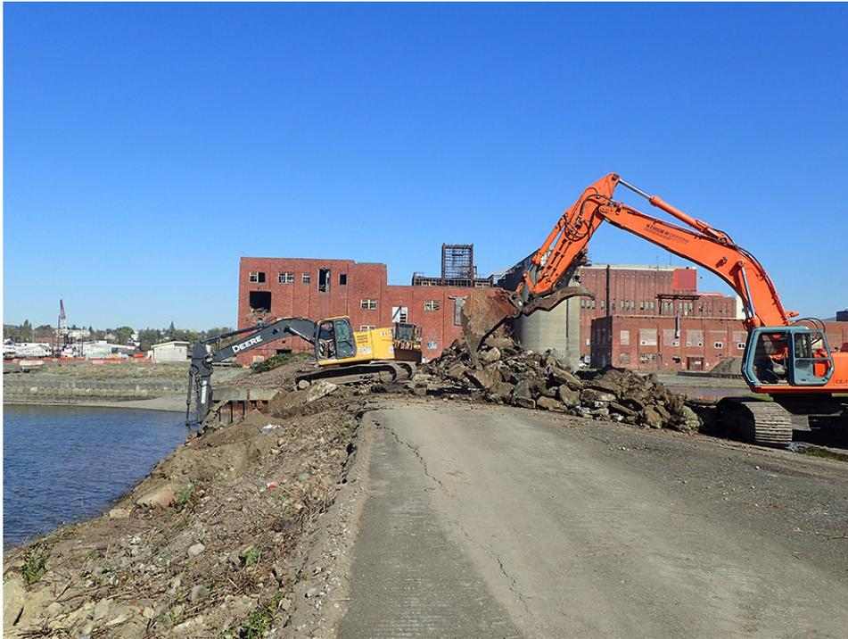
**Photograph 21: Log Pond Area shoreline debris removal.
