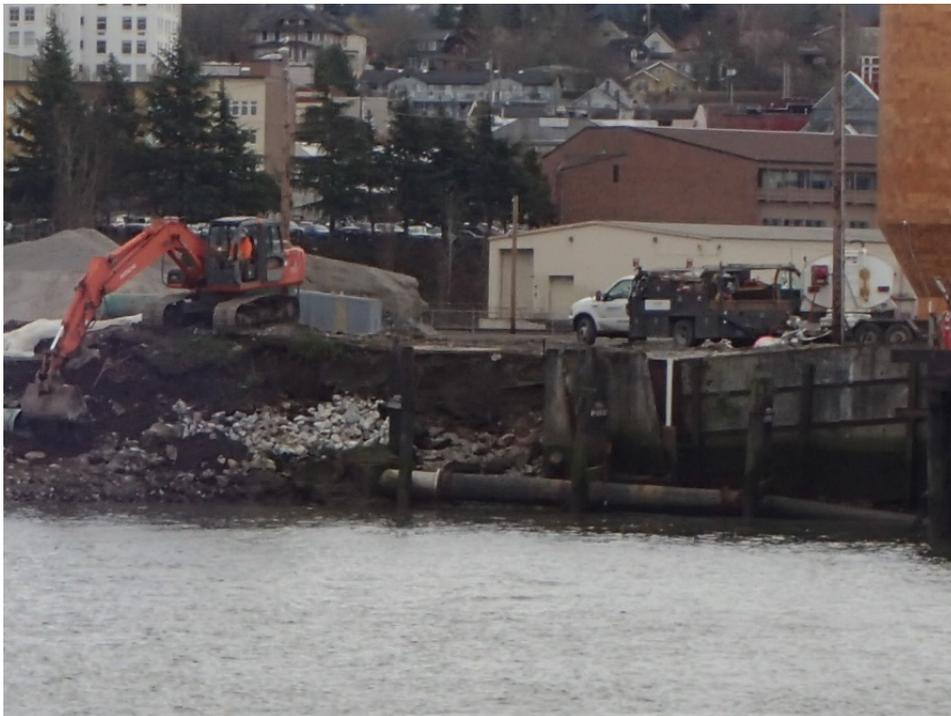
**Photograph 12: Foam tank area stormwater conveyance replacement. Facing east.**
