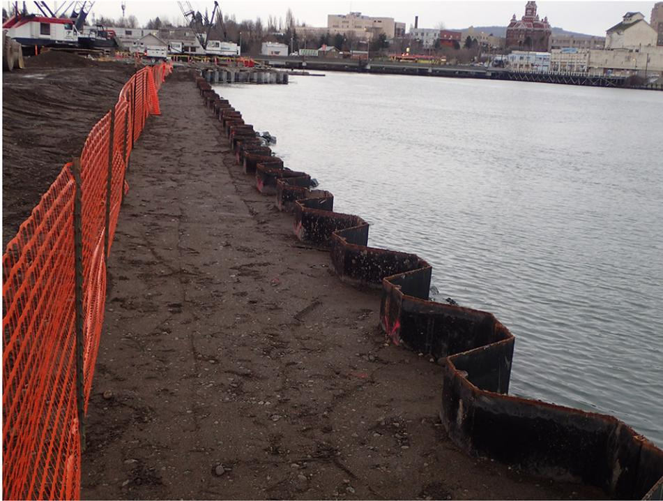
**Photograph 45: Central Waterfront: WCWW backfilled after dredging and capping. Facing east.**
