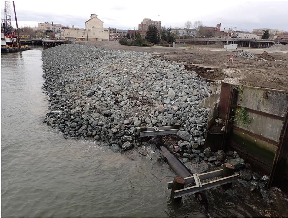
**Photograph 13: Foam tank area during capping.
