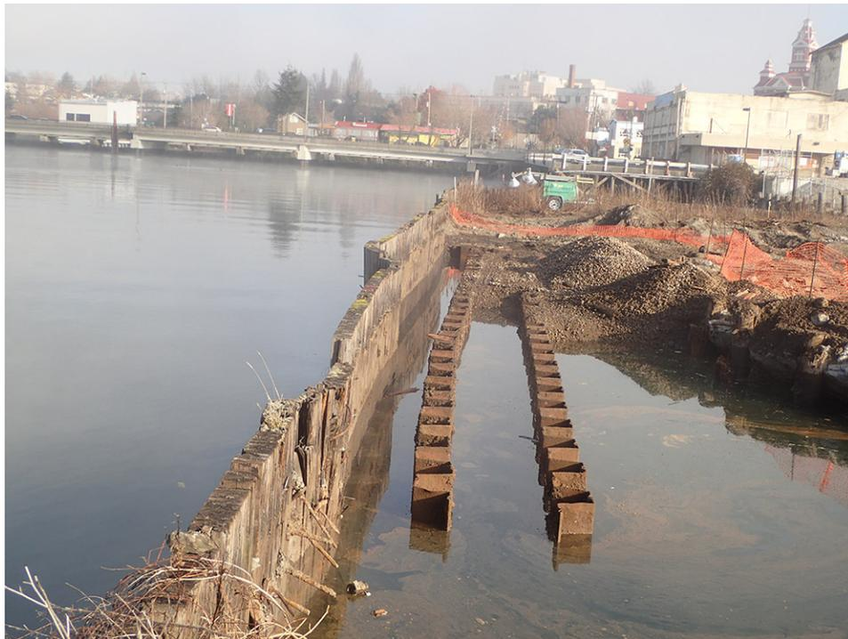
**Photograph 4: South shoreline during removal of the steel sheetpile bulkhead. Facing east.**
