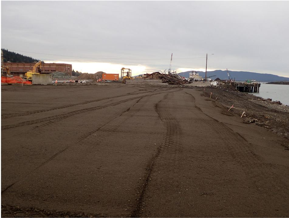
**Photograph 7: South shoreline during capping of former clarifier area.
