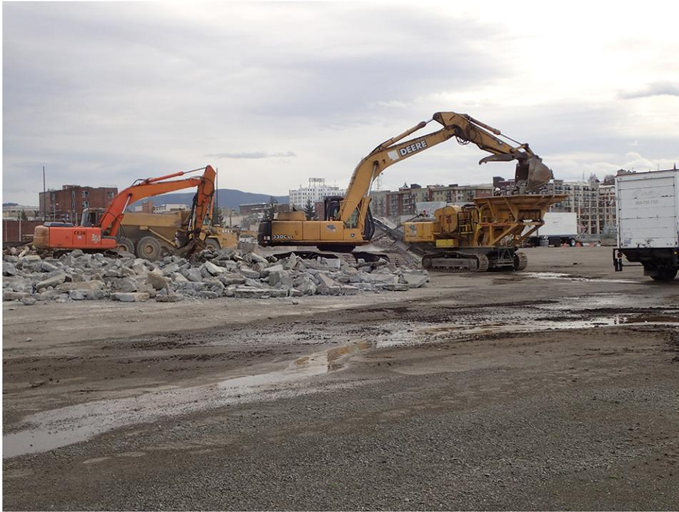
**Photograph 17: Former GP West SSA concrete reduction and sorting.
