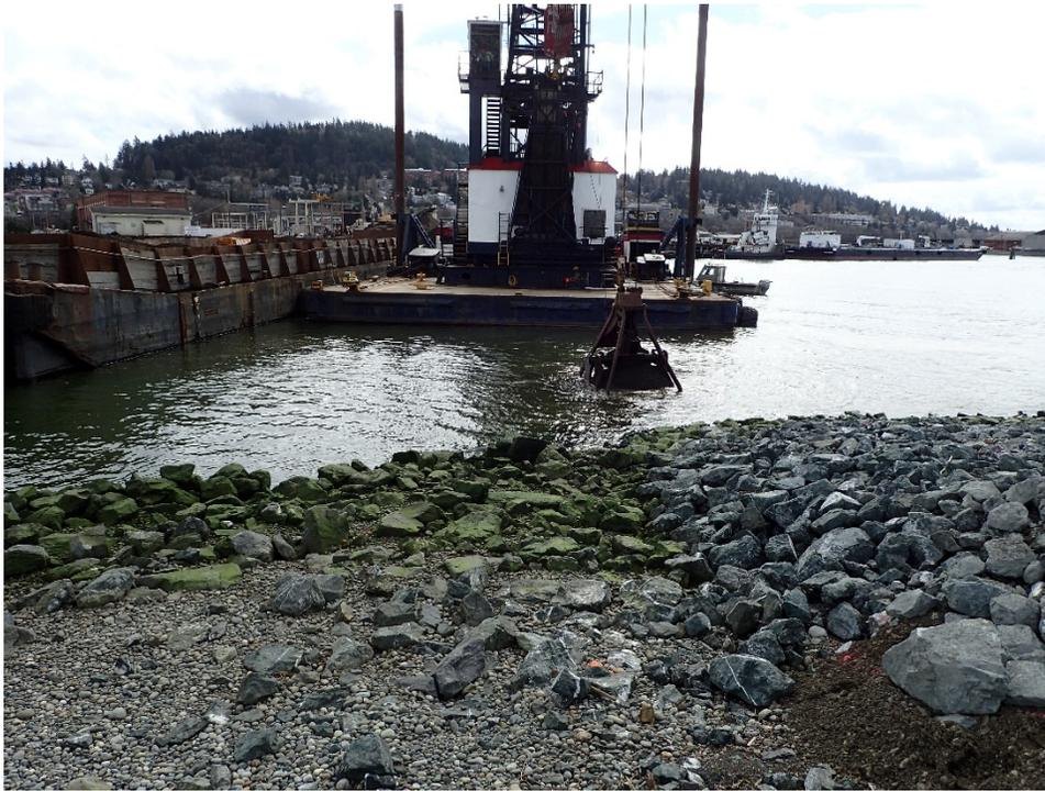
**Photograph 33: Inner Waterway capping operations.
