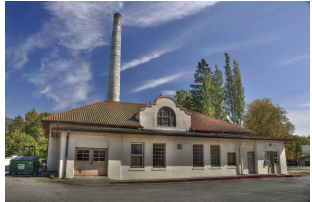
Power House Building, Summer 2017
