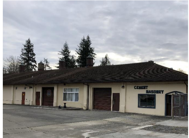
Former Laundry Building, January 2019
