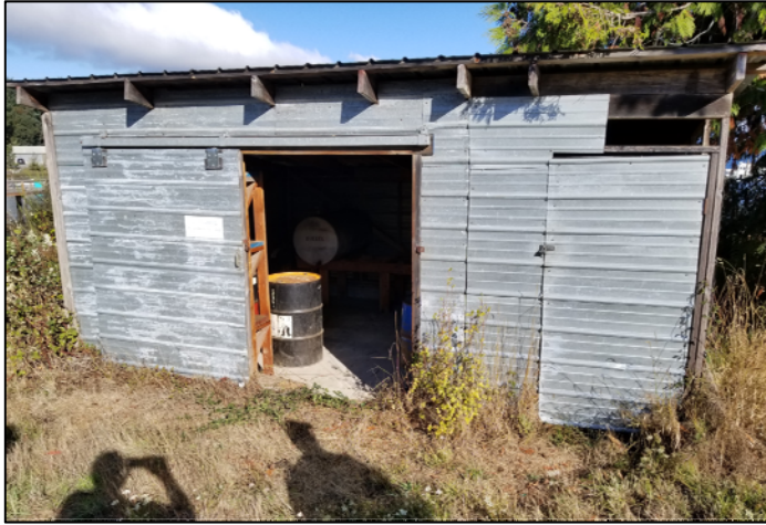
Photo 1. A view looking east at the oil storage building located at the northeast corner of the upland portion of the property.
