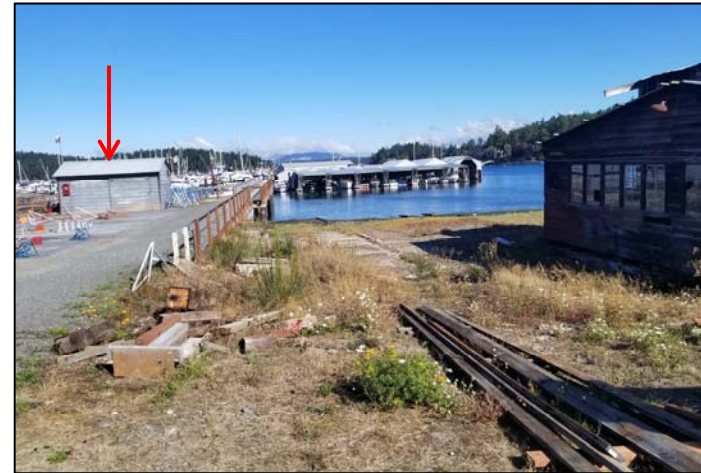
Photo 8. A view looking north along the dock. The wash water treatment building is visible in the distance (indicated by arrow).
