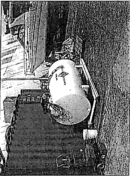
Photograph 17: View of diesel AST, facing northwest.
