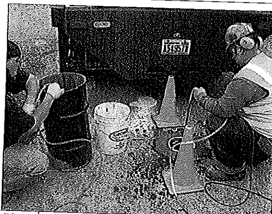
Photo #4: View of well development at AEGMW-3. Wells were purged with a sediment pump until the water became clear and free of sediment.
