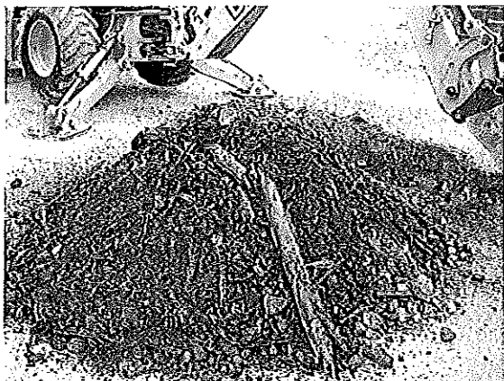
Photo #7: View of the excavation of TP-7. Note the presence of a large amount of wood debris in the fill material found at the Site.
