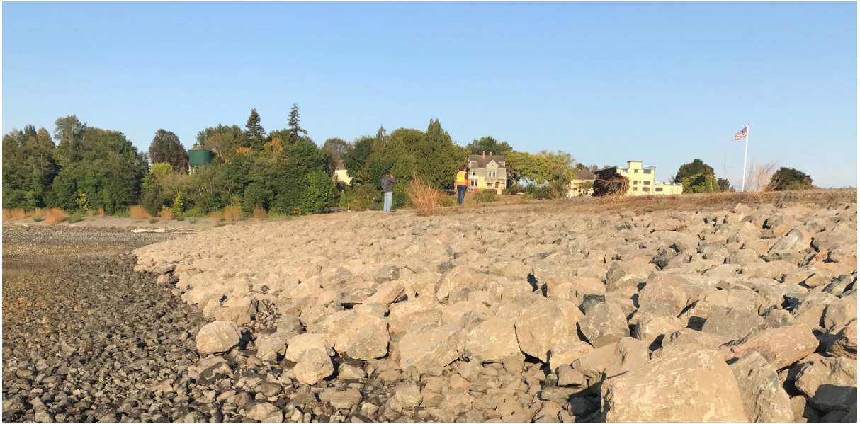
Figure 11 Photograph of Repaired SMA-2 Intertidal Cap Area
