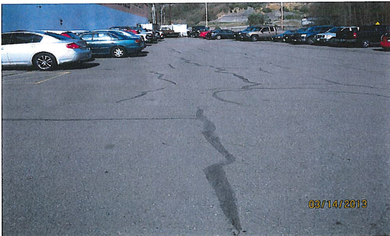
Photo 8: Patched/Repaired Asphalt Cap – From Southeast
