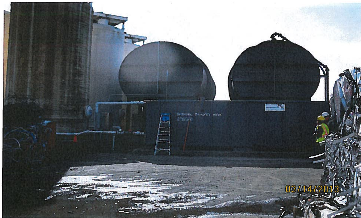
Photo 6: Storm Water Storage and Treatment Systems – Sequential Filtration
