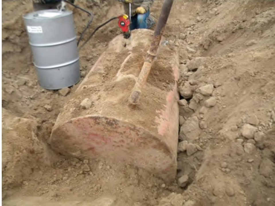
Figure 5: Pumping Fuel from Tank
