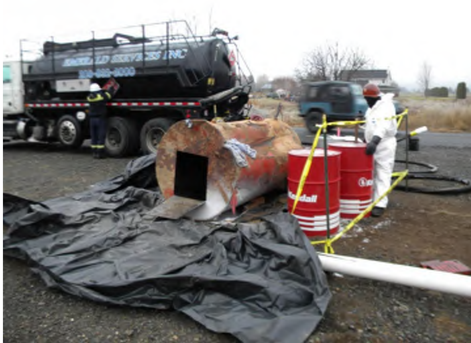
Figure 17: Cleaning out barrels
