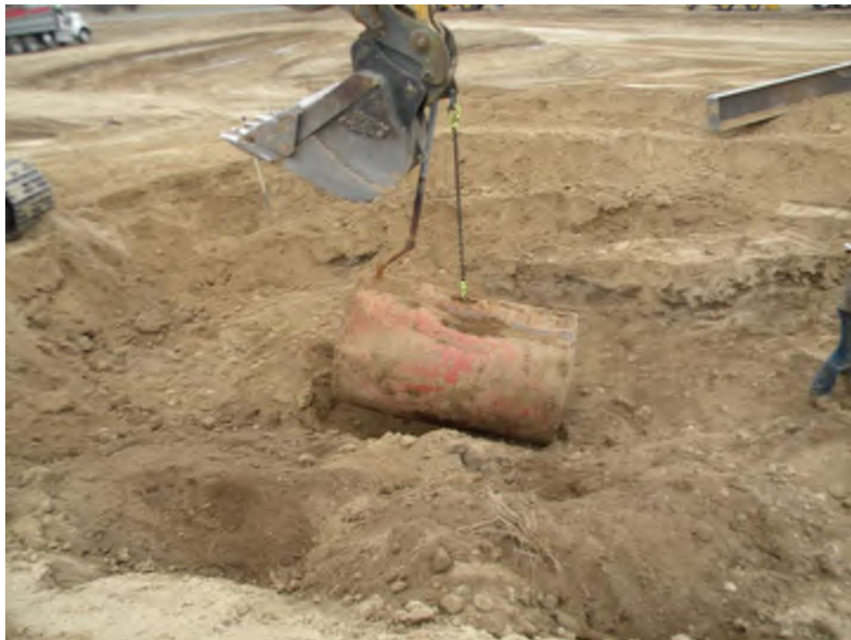
Figure 6: Removing empty tank
