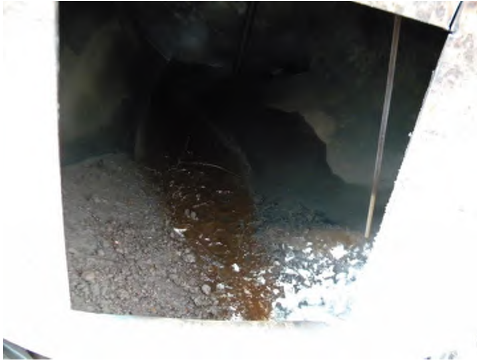
Figure 15: Sediment inside tank
