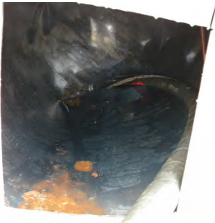
Figure 18: Cleaned tank for disposal
