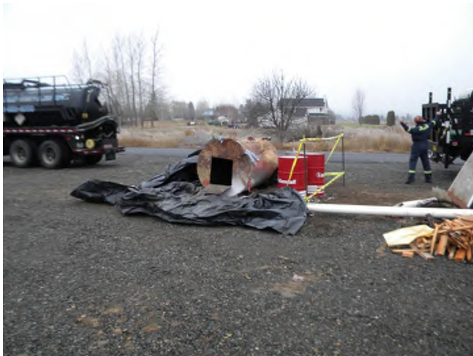
Figure 14: Tank cut for cleanout after inerting with dry ice
