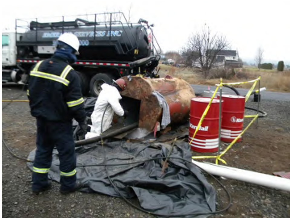
Figure 16: Cleaning out tank
