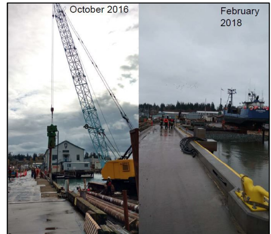
Figure 3: Harris Avenue Pier before and after the 2018 interim action
