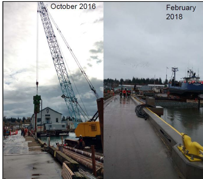
Figure 4: Harris Avenue Pier before/after Interim Action
