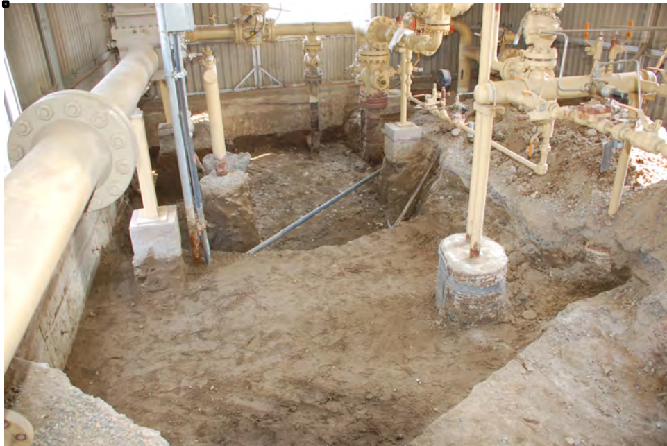
3. Looking at remedial excavation inside meter building.
