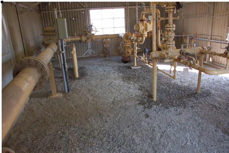
4. Looking at completed restoration inside meter building.
