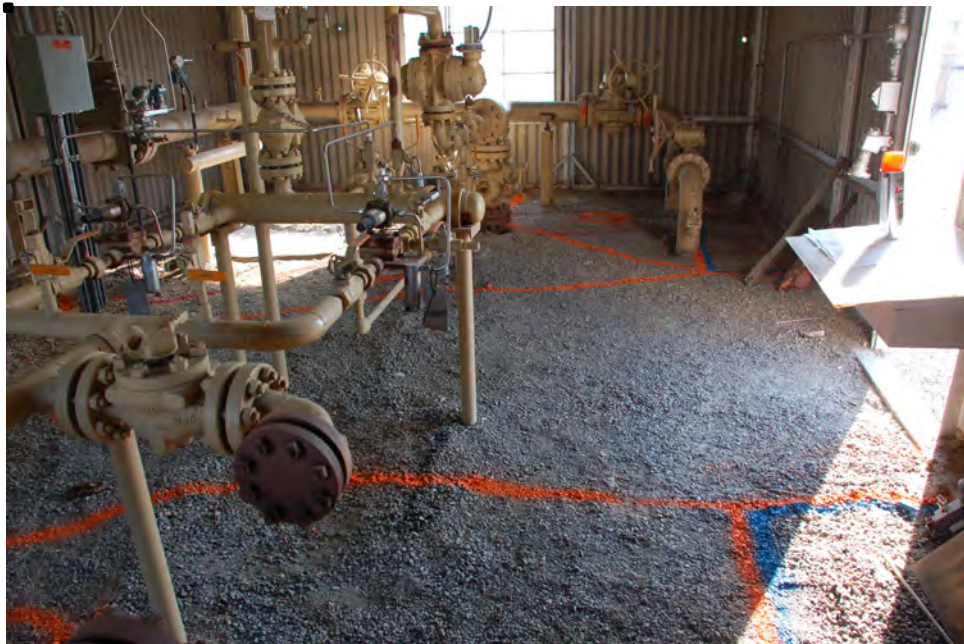
2. Looking at remedial area inside meter building.
