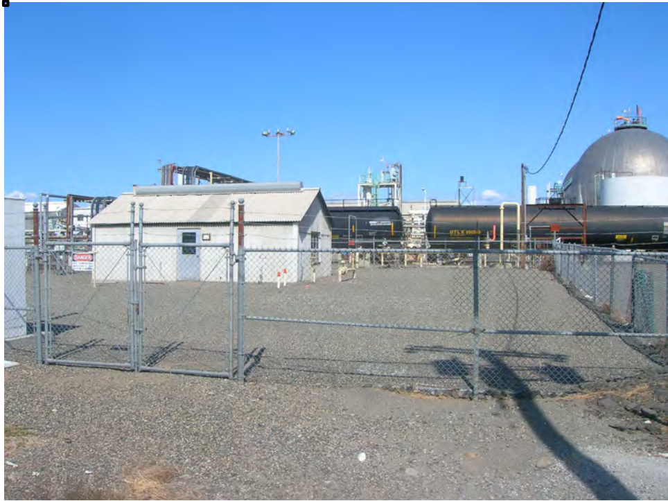
1. Looking at meter building.
