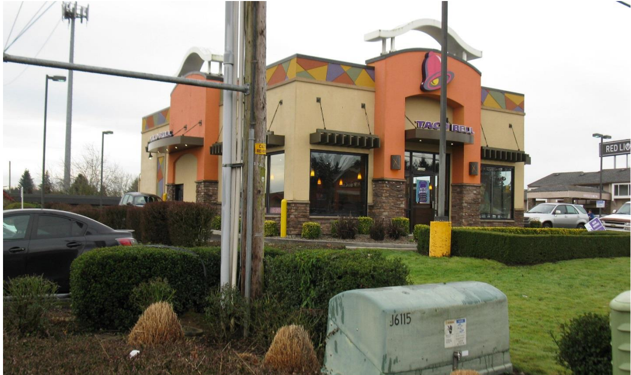
Photo 3: Current Taco Bell Restaurant and Landscape/ Former Exxon Station – from the Southeast
