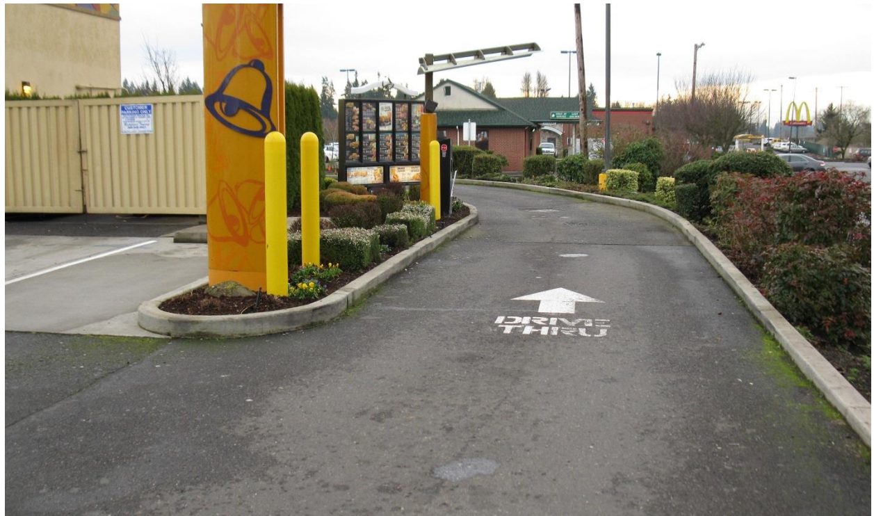
Photo 4: Current Drive-Through / Former Fuel and Waste Oil Storage USTs Location – from the North
