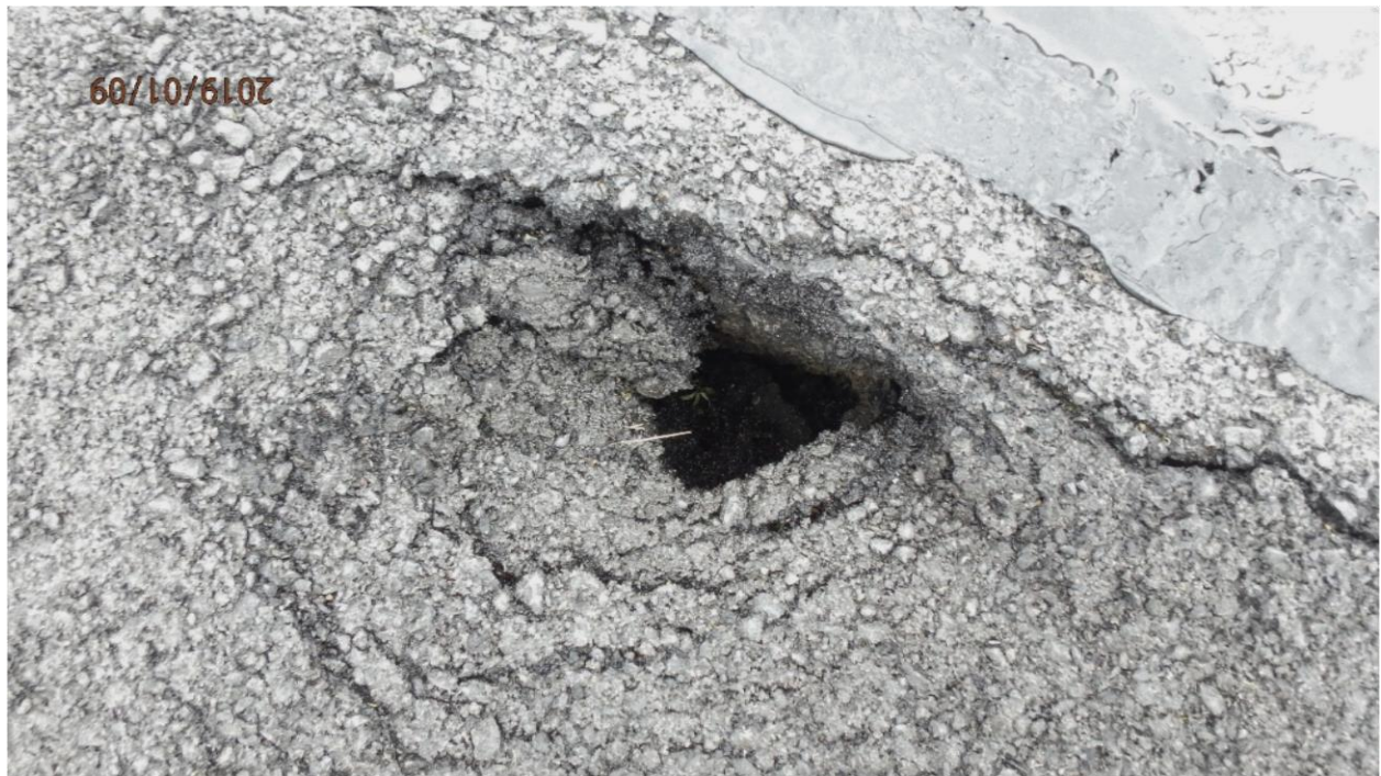
Photo 1. Hole on west side of pavement settlement area: RA-3 (map note 1)
