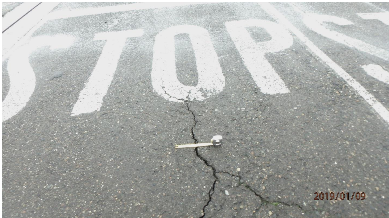
Photo 6. Mound in pavement with cracks as wide as 1 in.: RA-3 (map note 6)
