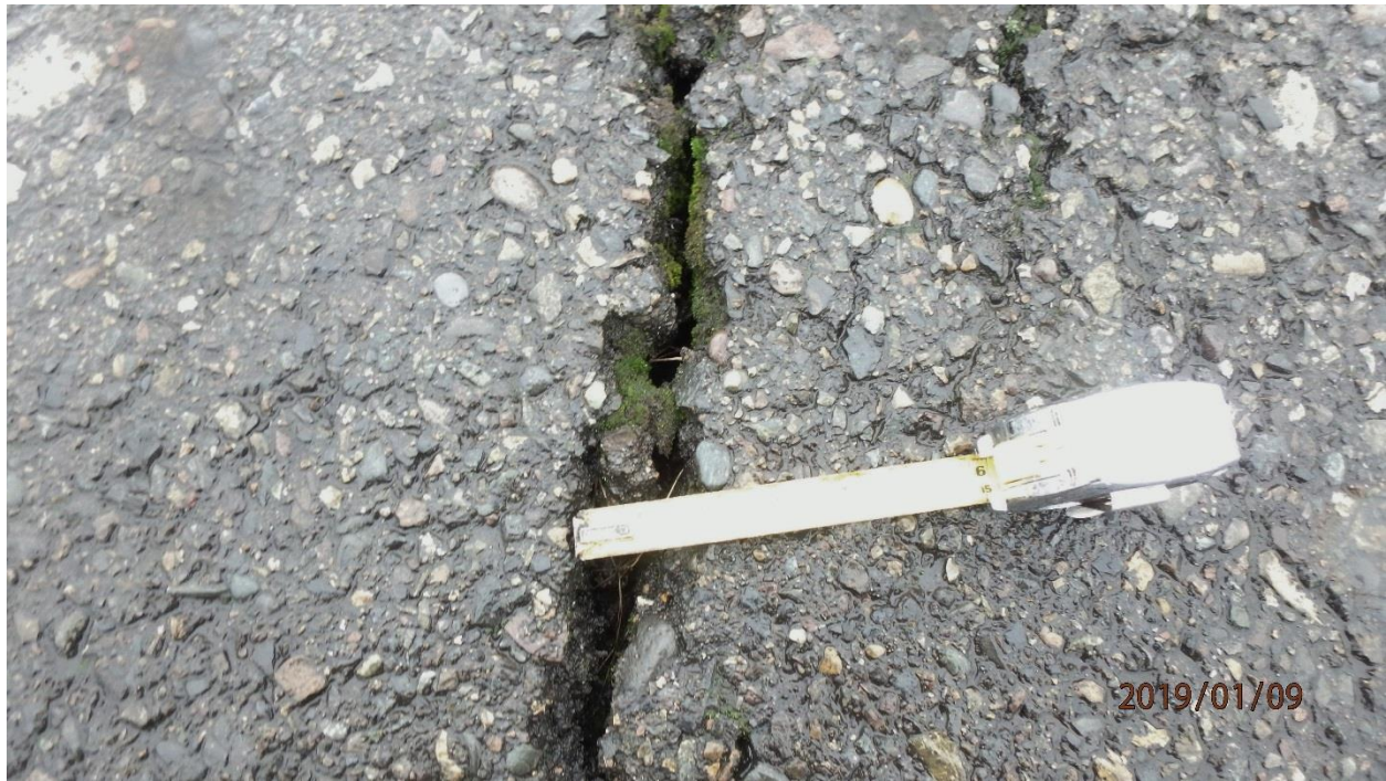
Photo 3. Close-up of mound in pavement with cracks as wide as 2 in.: RA-2 (map note 4)
