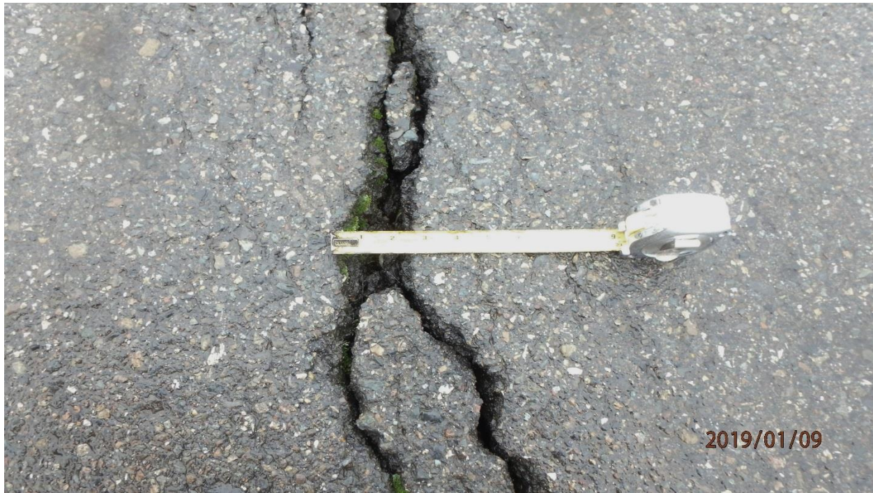
Photo 11. Close-up of mound in pavement with cracks as wide as 3 in.: RA-2 (map note 8)
