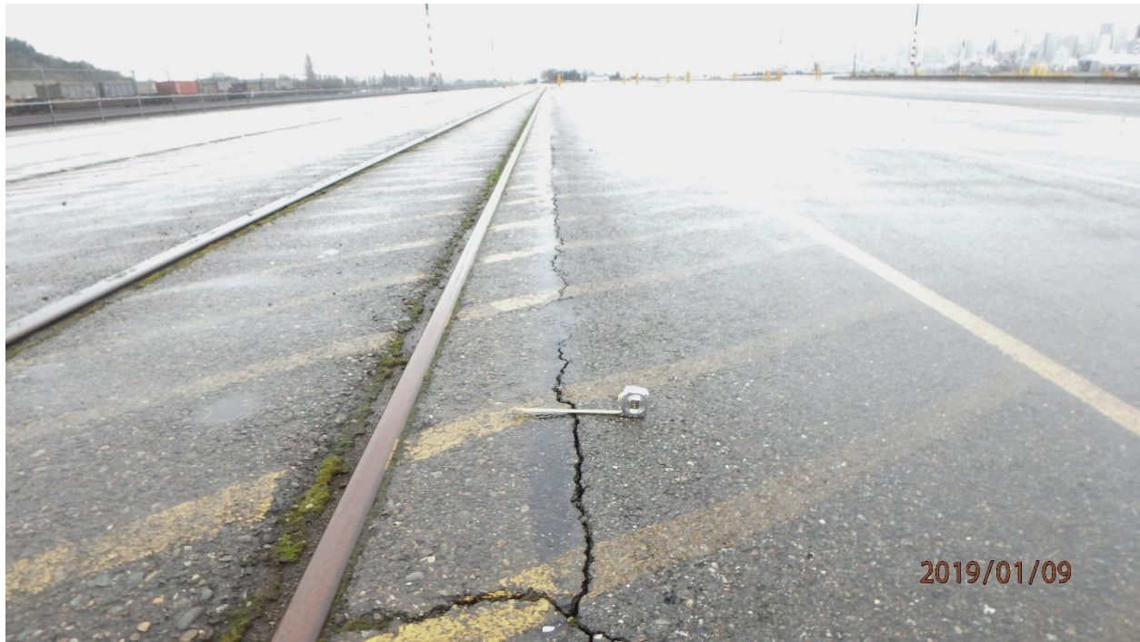
Photo 15. Crack as wide as 1 in.: RA-3 (map note 12)
