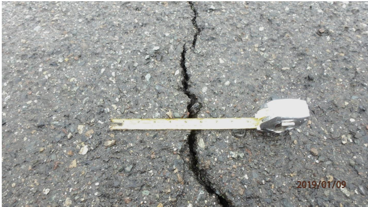
Photo 7. Mound in pavement with cracks as wide as 1 in.: RA-3 (map note 6)
