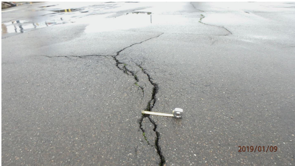
Photo 10. Mound in pavement with cracks as wide as 3 in.: RA-2 (map note 8)
