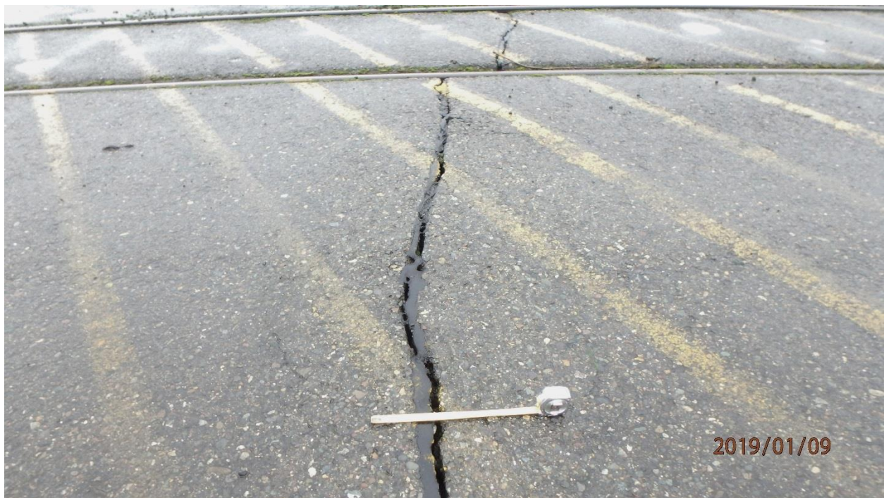
Photo 14. Crack as wide as 2 in.: RA-3 (map note 11)
