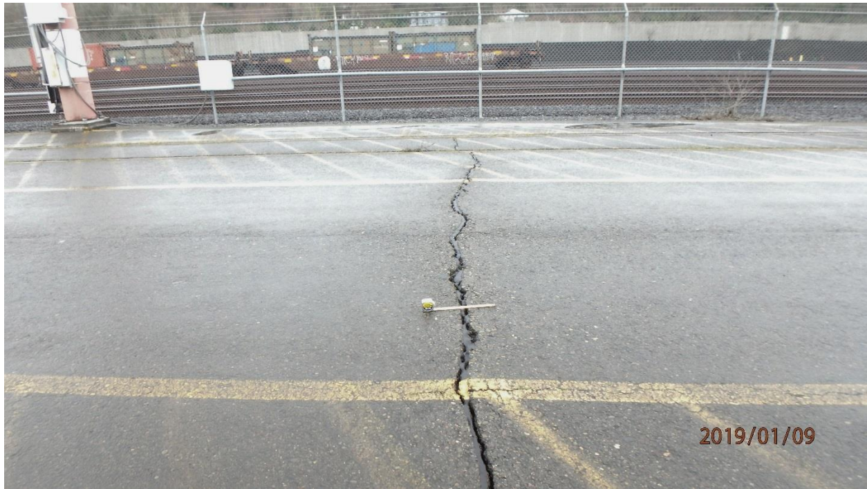
Photo 13. Crack as wide as 1.25 in.: RA-3 (map note 10)
