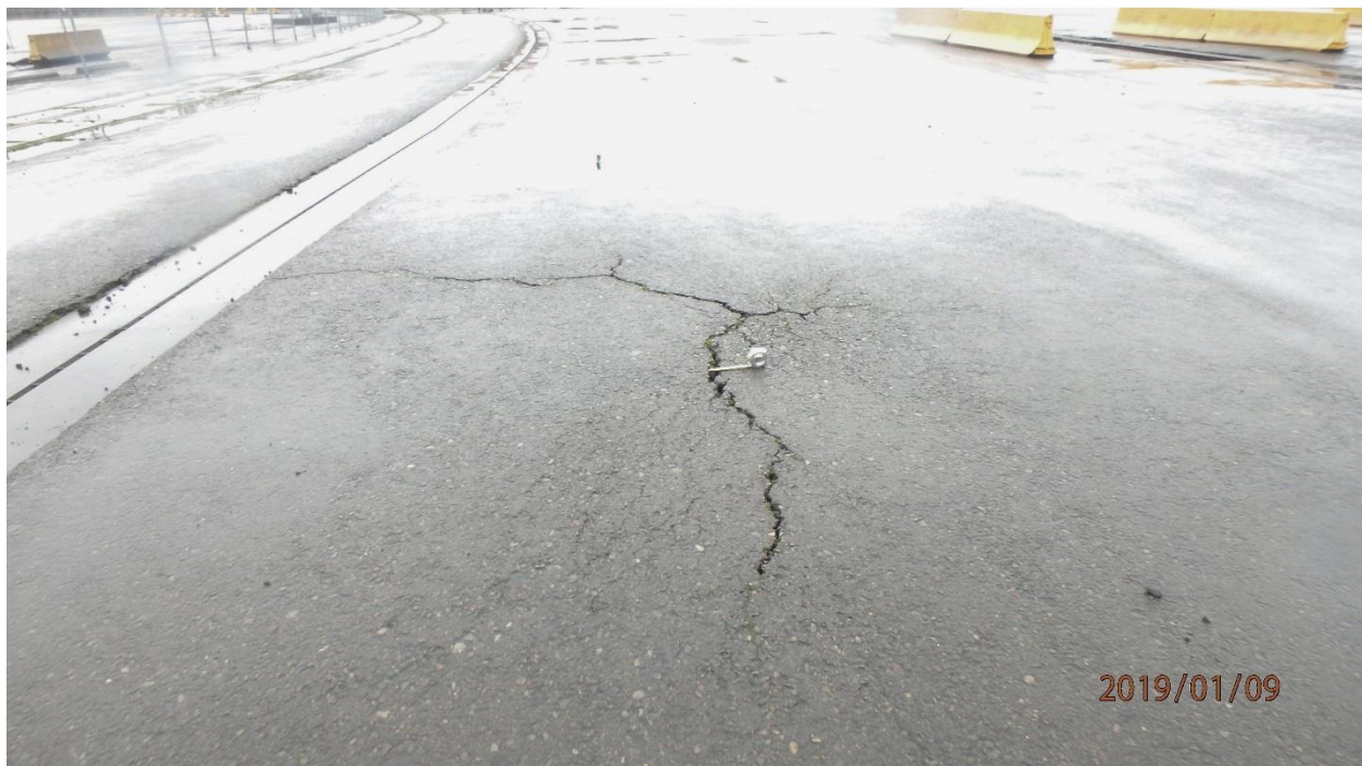
Photo 2. Mound in pavement with cracks as wide as 2 in.: RA-2 (map note 4)
