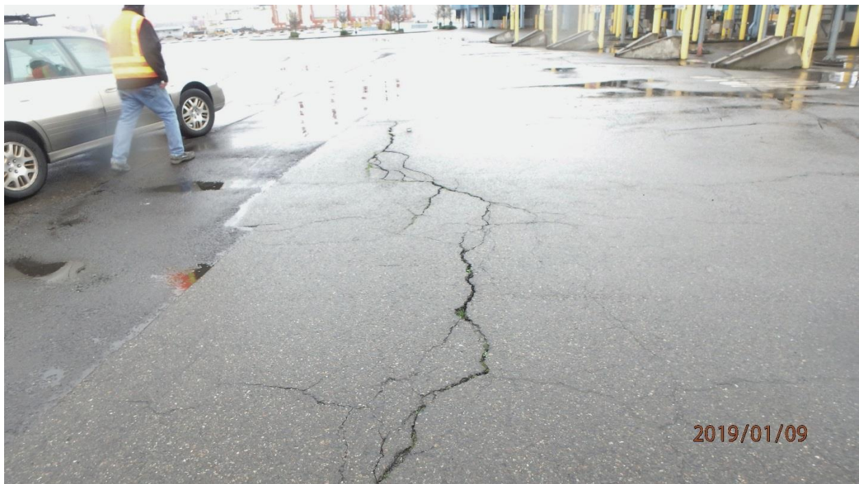
Photo 8. Elongated mound in pavement with cracks as wide as 2 in.: RA-2 (map note 7)
