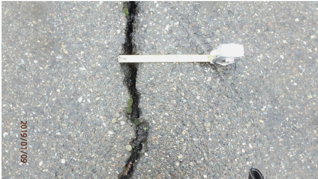
Photo 9. Close up of elongated mound in pavement with cracks as wide as 2 in.: RA-2 (map note 7)
