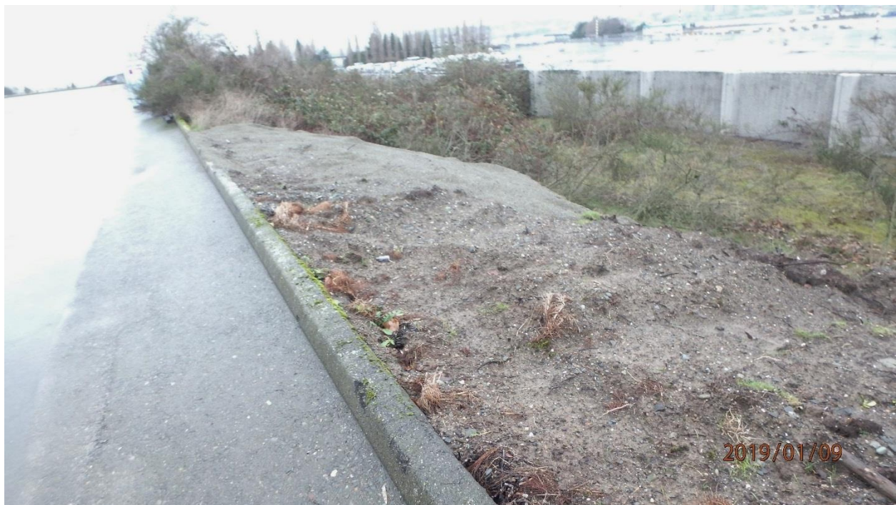
Photo 18. Representative photo of three areas on east landfill slope, cleared of vegetation and covered with loose soil: RA-3 (map notes 17, 18, and 19)
