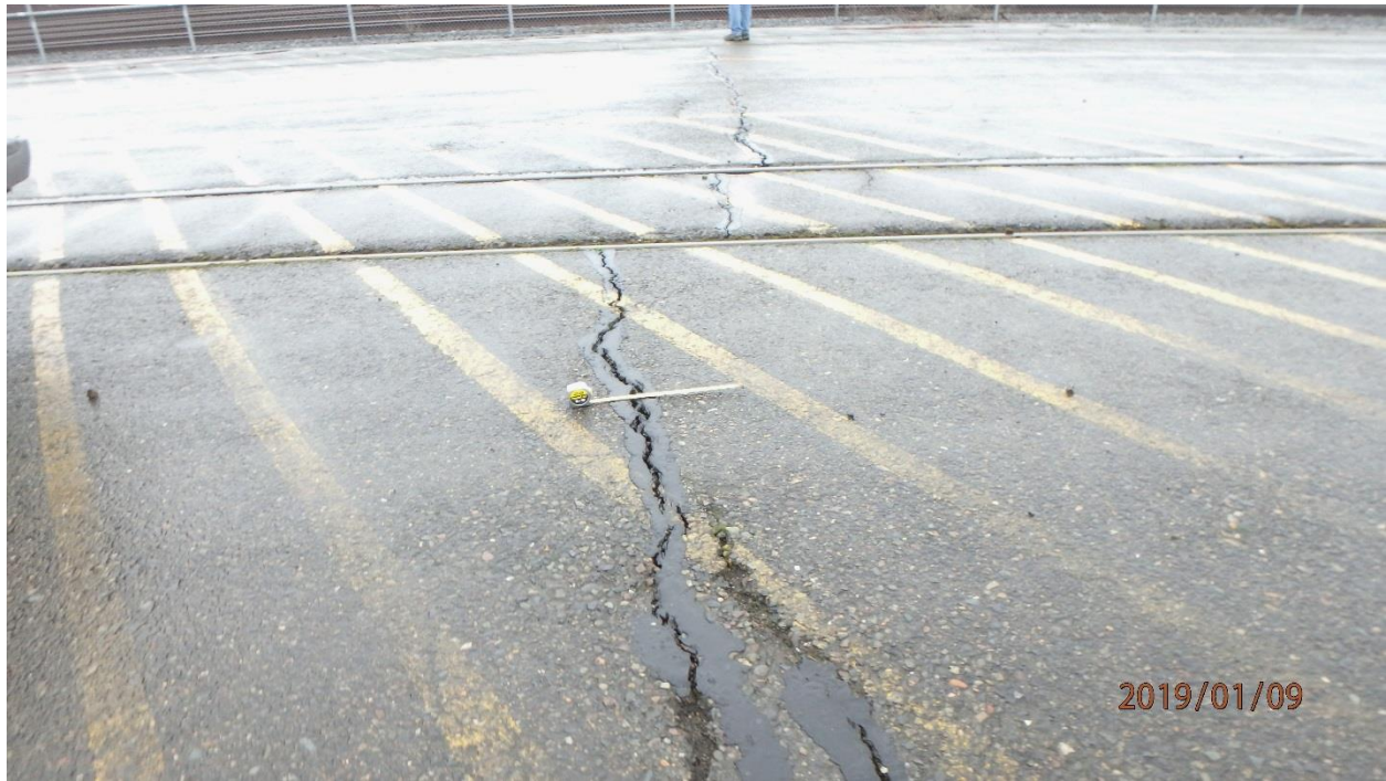
Photo 17. Crack as wide as 2 in.: RA-3 (map note 14)
