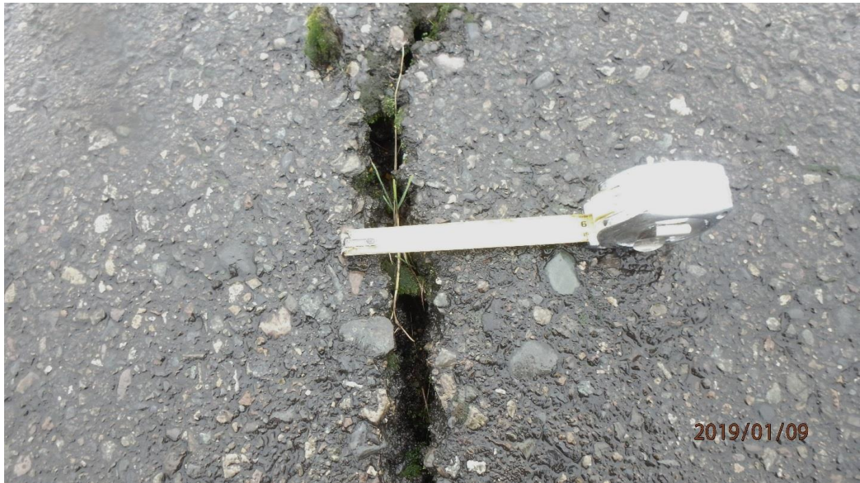
Photo 5. Close-up of mound in pavement with cracks as wide as 2 in.: RA-2 (map note 5)
