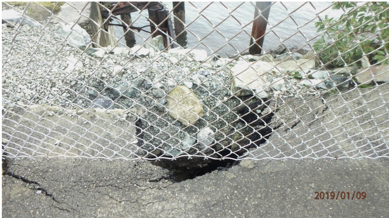
Photo 12. Hole and cracking in pavement near northeast corner of site: RA-5 (map note 9)
