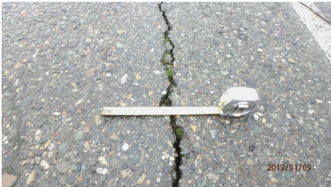
Photo 16. Crack as wide as 1 in.: RA-3 (map note 13)
