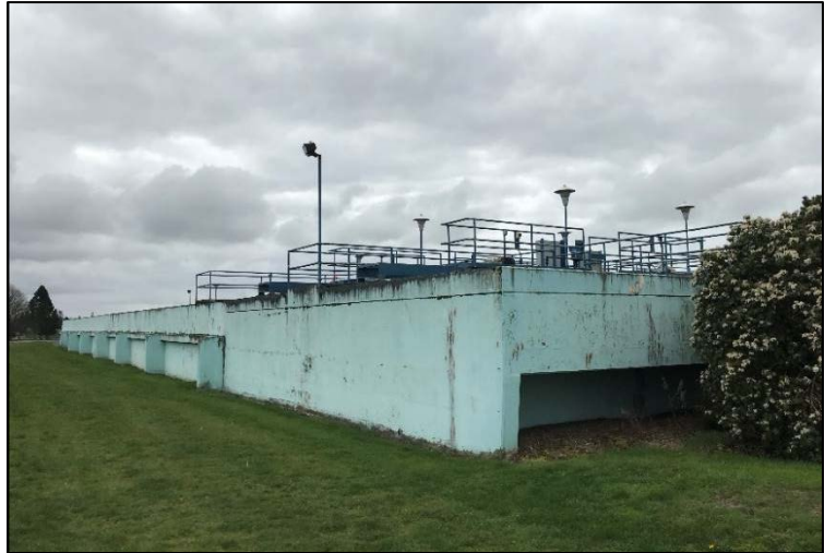
Figure 6: Decommissioned Sedimentation Basin, March 2018
