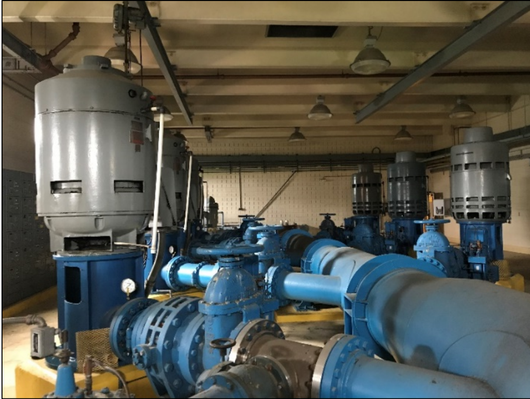
Figure 4: Decommissioned Pump Room below Administration Building, March 2018
