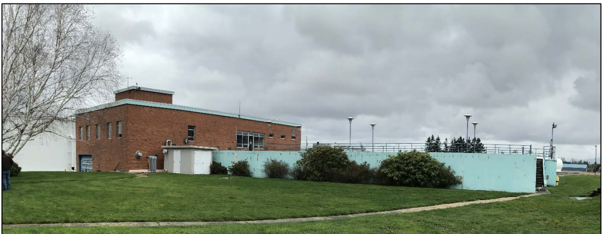
Figure 5: Decommissioned Administration Building and Filtration Basin facing North, March 2018
