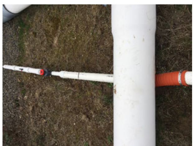
After Well Head Replacement at N-4
