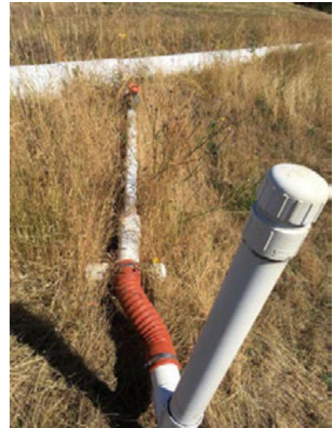
After Repaired 3-in PVC T at E22
