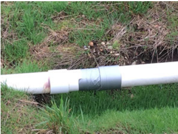
Before 12-in Lateral Installation at E-39
