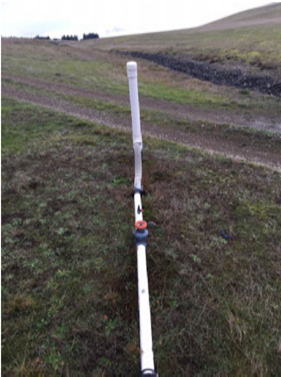
Before Hose Replacement at N-37
