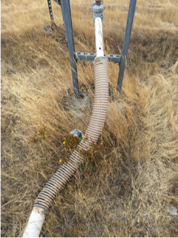
N-12 Before Repairs
