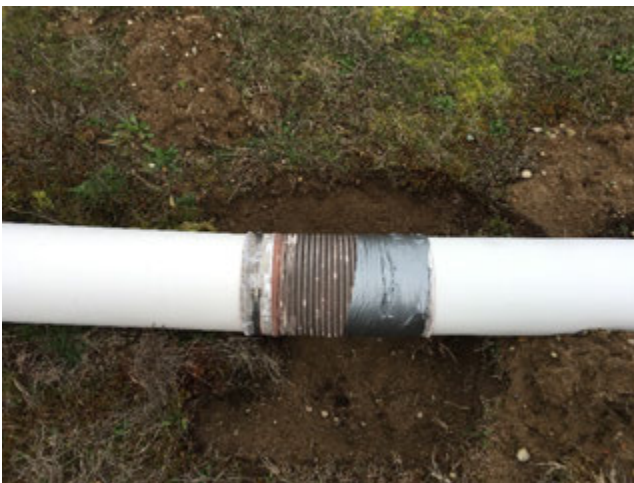
Before Hose Replacement at N-3
