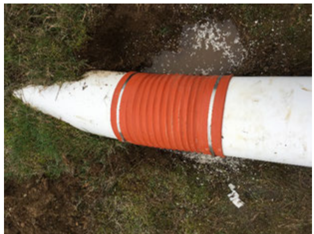
After Hose Replacement at N-4
