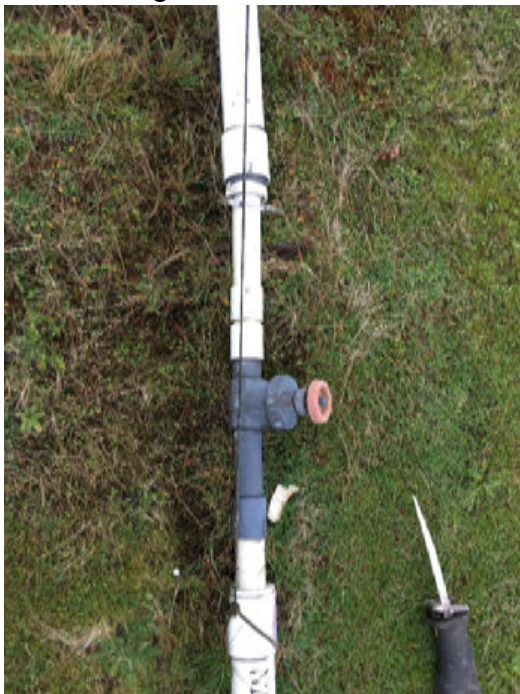
Before Hose and Valve Replacement at N-23
