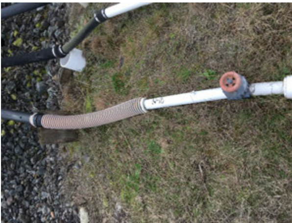
Before Hose and Valve Replacement at N-48
