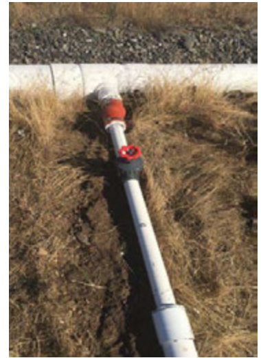
After Well Head at E16 Repair
