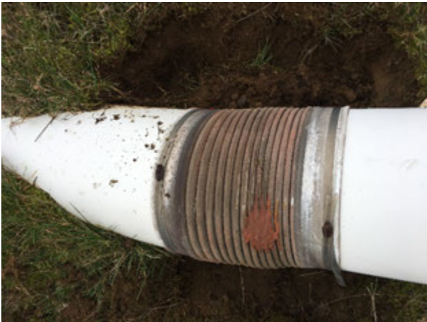
Before Hose Replacement at N-4
