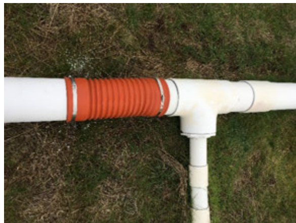
After 6-in Hose Installation at E-7
