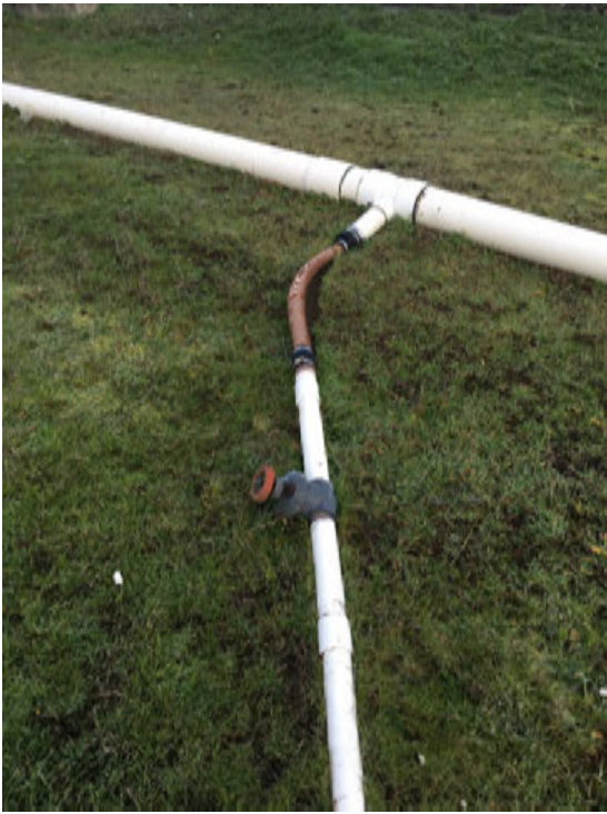
Before Hose and Valve Replacement at N-65
