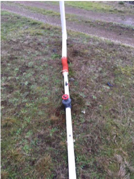
After Hose Replacement at N-37
