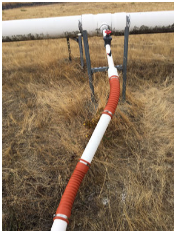
N-12 After Repairs
