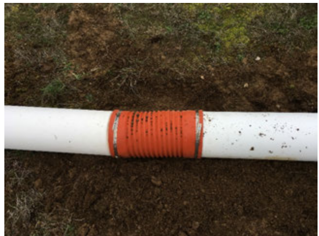
After Hose Replacement at N-3
