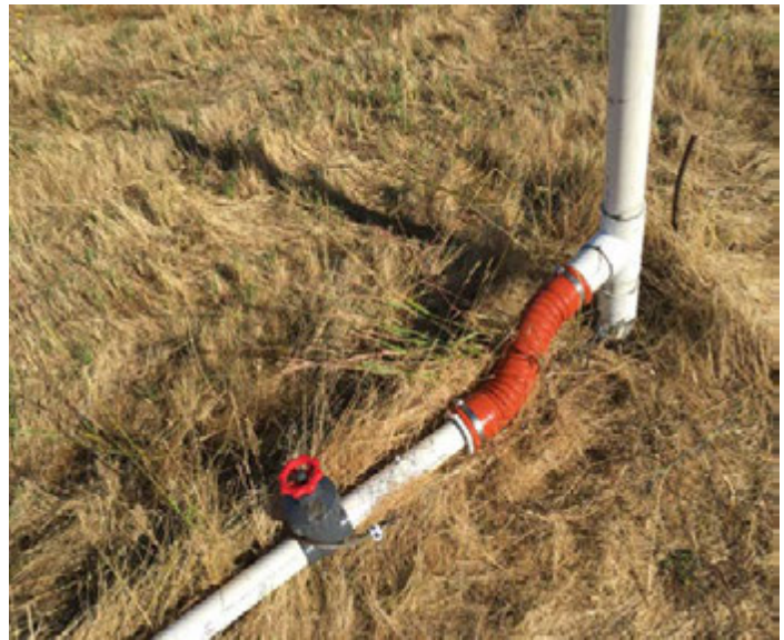
After E9A Well Head Repairs
