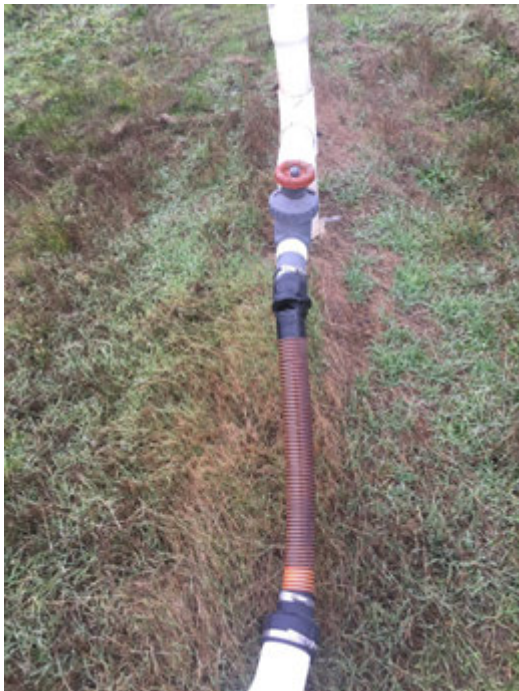
Before Hose Replacement at E-7
