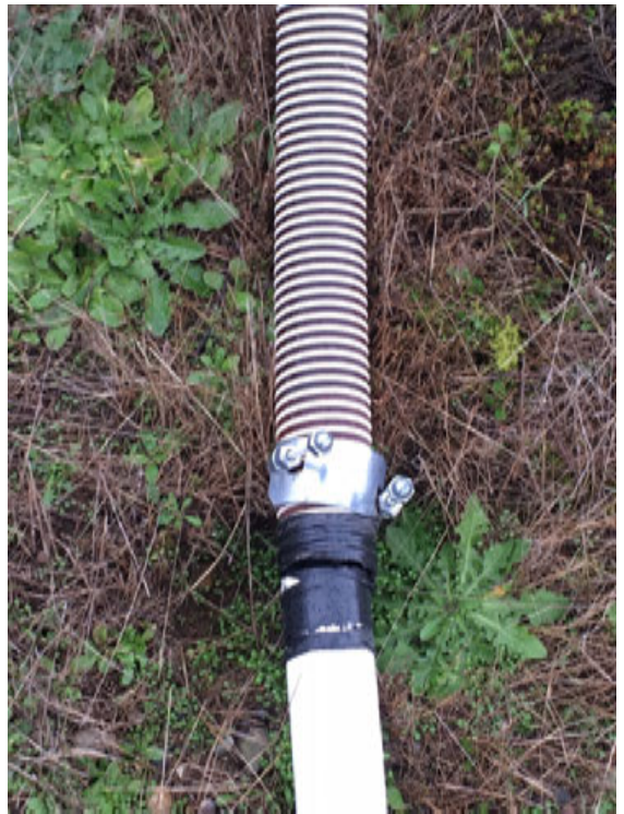
Before Hose Replacement at N-37
