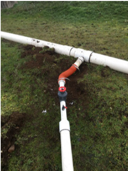
After Hose and Valve Replacement at N-65
