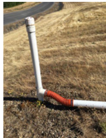
After Replaced 3-in LFG Hose at N25
