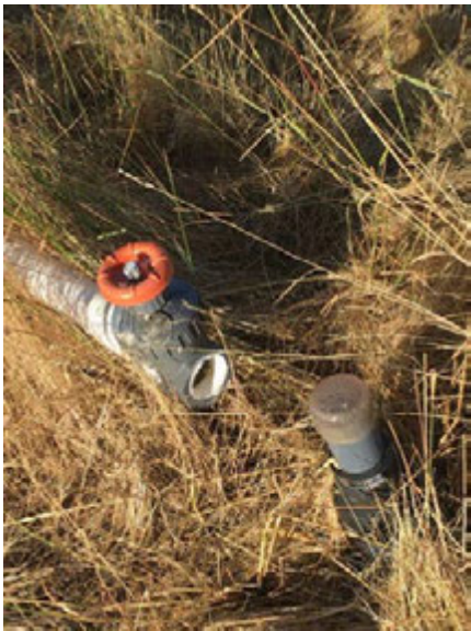
Before E9A Well Head Repairs
