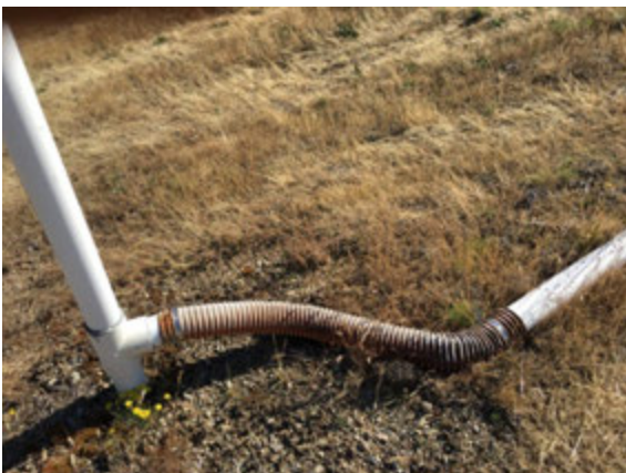
Before Replaced 3-in LFG Hose at N25
