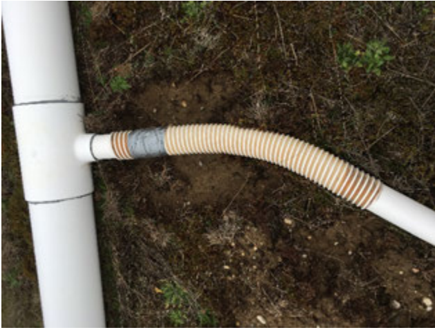
Before Hose Replacement at N-3
