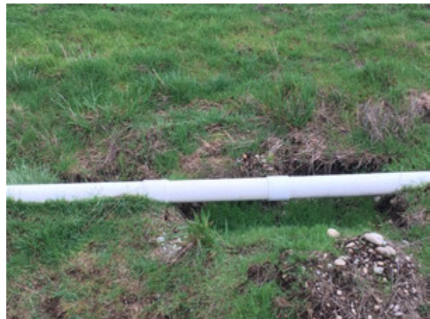
After 12-in Lateral Installation at E-39
