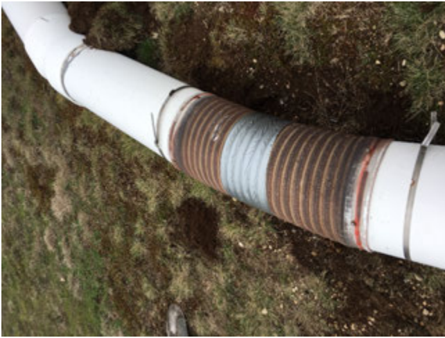
Before Hose Replacement at N-15
