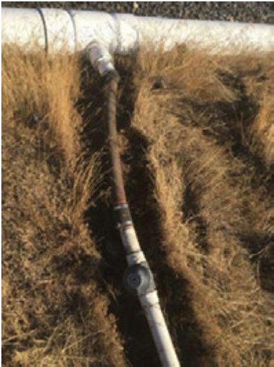
Before Well Head at E16 Repair
