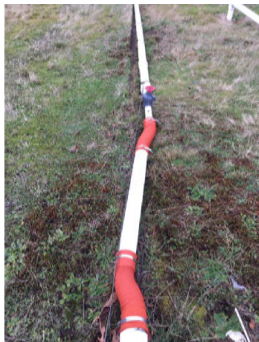
After Replacement at N-23
