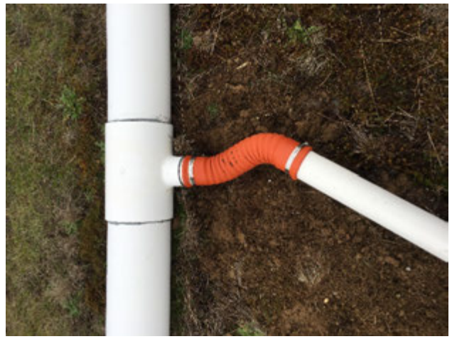
After Hose Replacement at N-3
