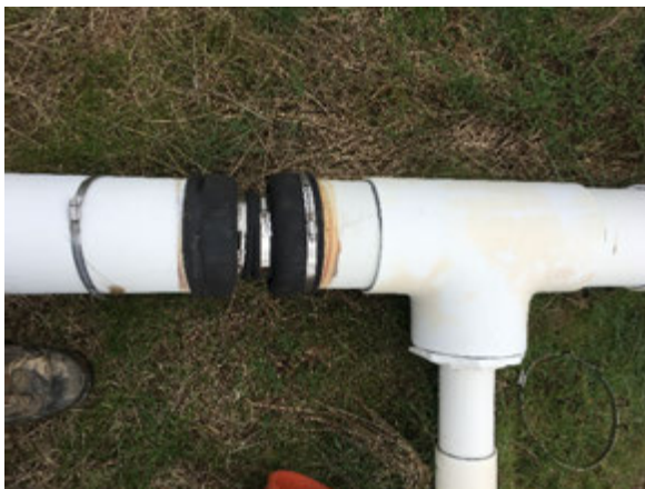
Before 6-in Hose Installation at E-7
