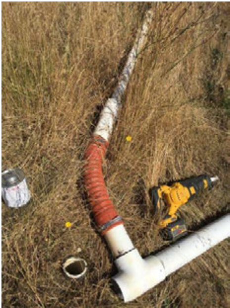
Before Repaired 3-in PVC T at E22
