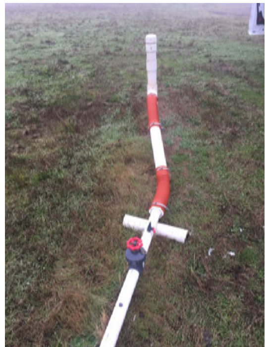
After Hose Replacement at E-7
