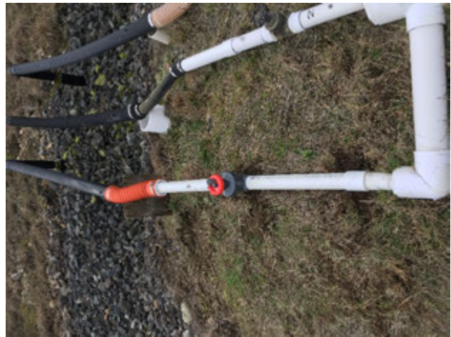
After Hose and Valve Replacement at N-48
