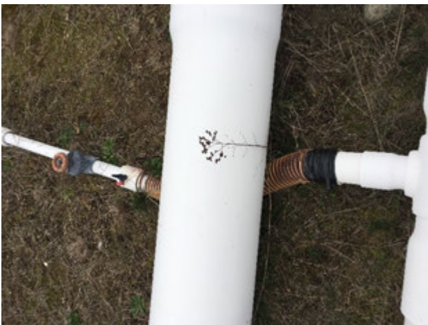
Before Well Head Replacement at N-4
