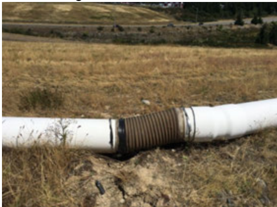
Before 12-in x 36-in Hose Installation at N12
