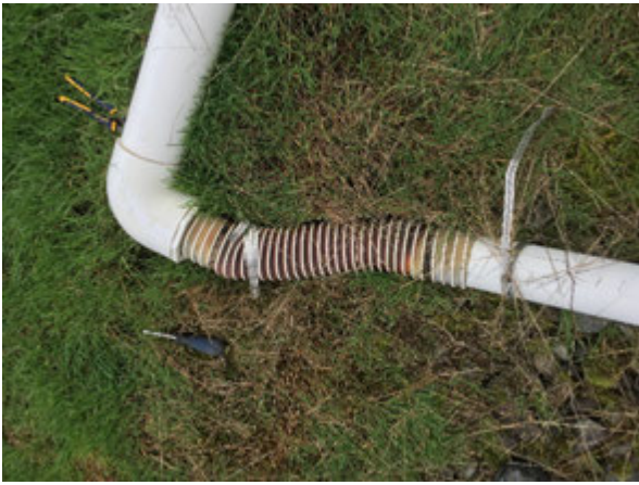
Before 4-in Lateral Installation at E-39
