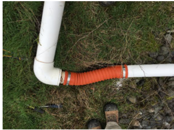
After 4-in Lateral Installation at E-39
