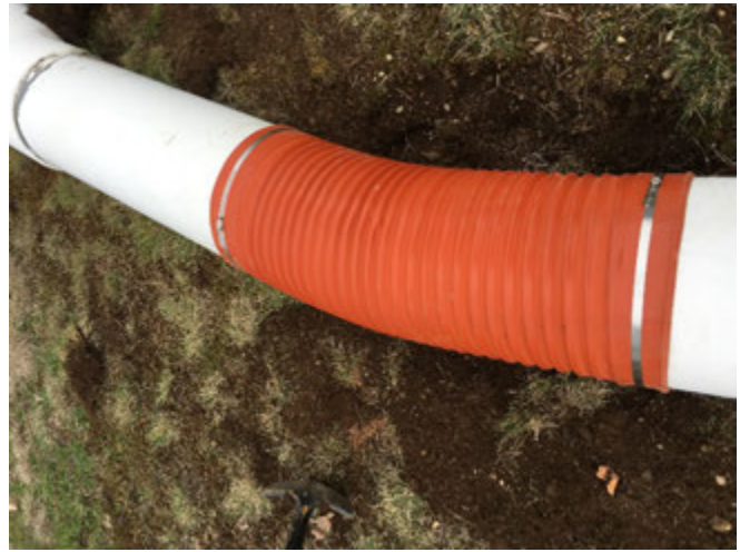
After Hose Replacement at N-15
