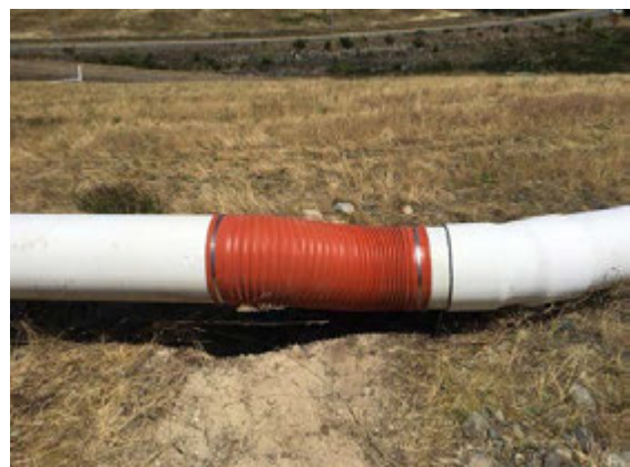
After 12-in x 36-in Hose Installation at N12
