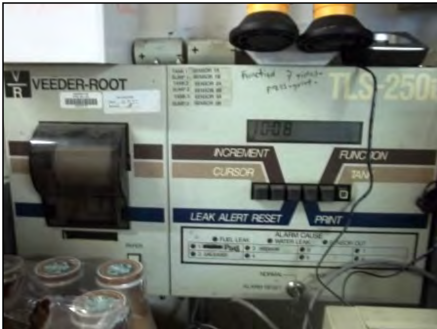
12 : Veeder-Root UST systems monitor
