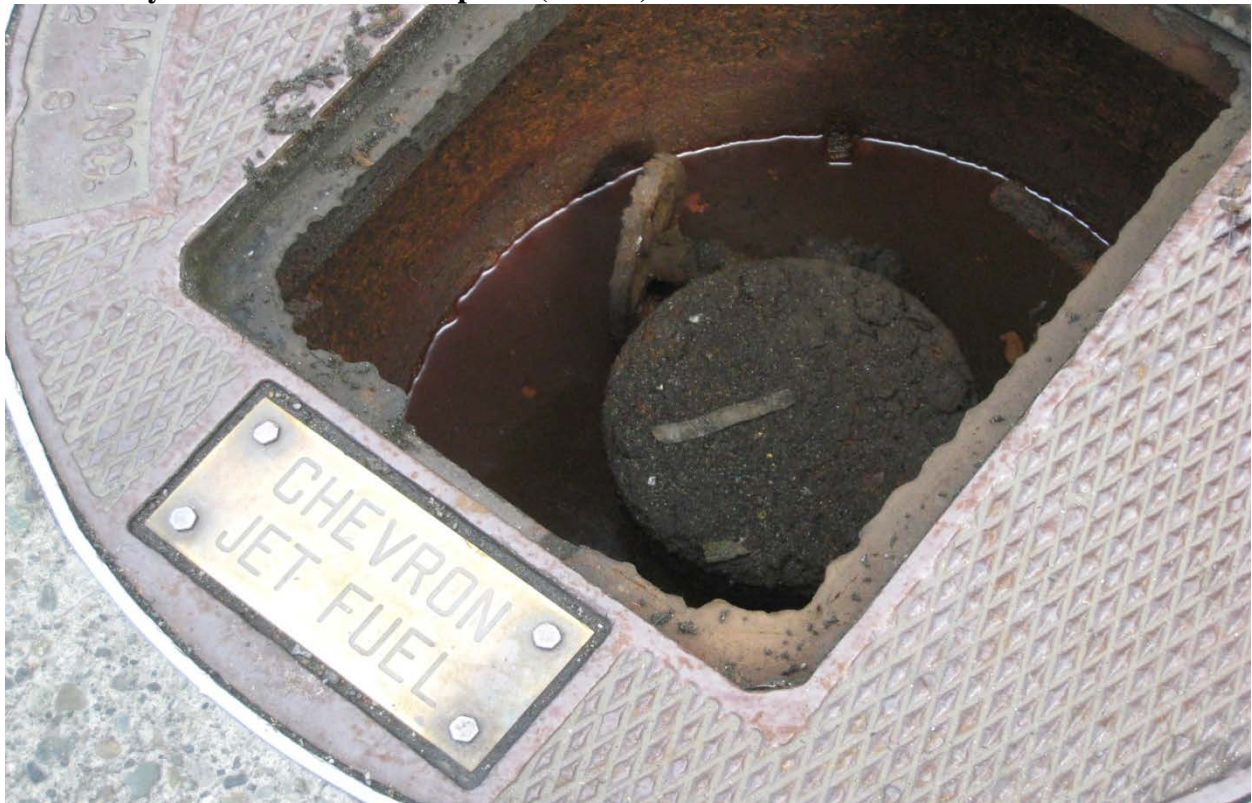
Photo 4: Hydrant fuel line access point (bucket) with cover off. Others have no water.
