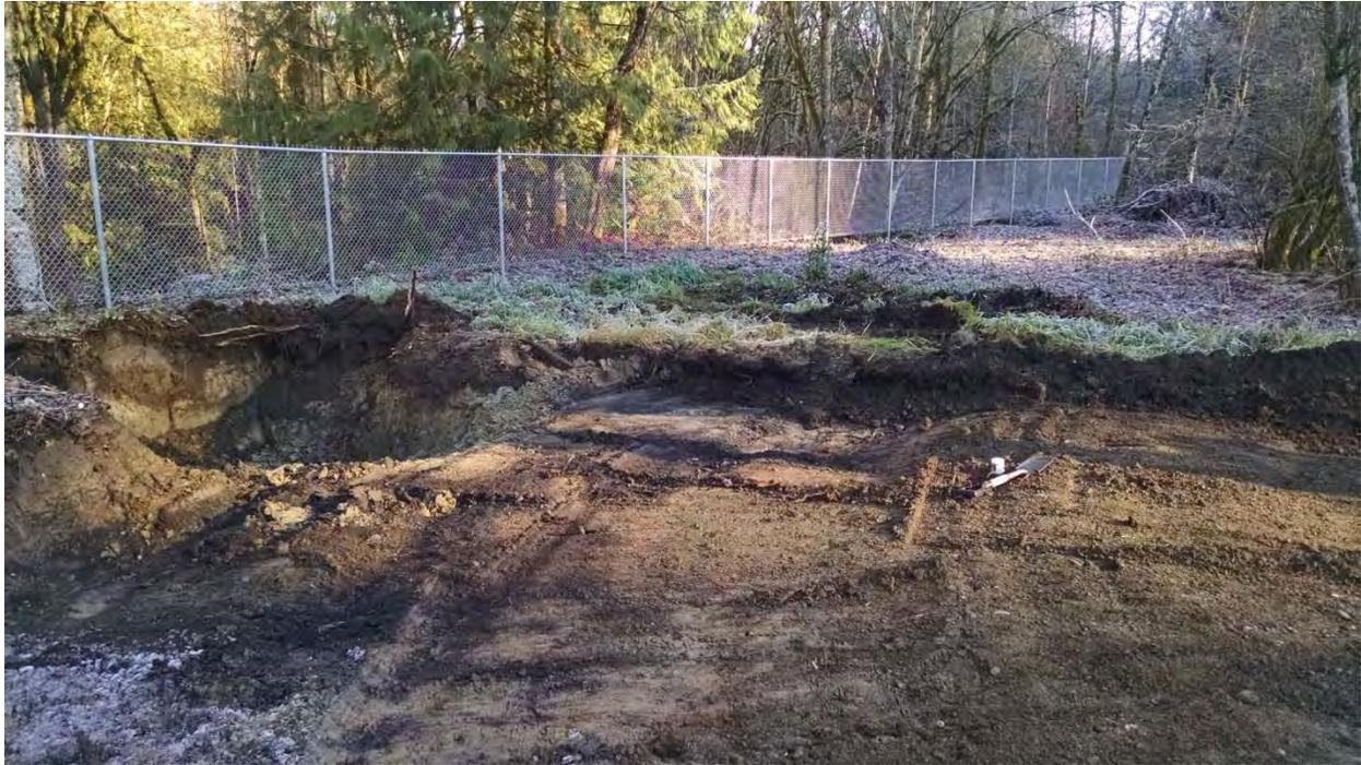
Expansion of northeastern corner of excavation, including deeper soil removal due to debris (as of December 5, 2018)
