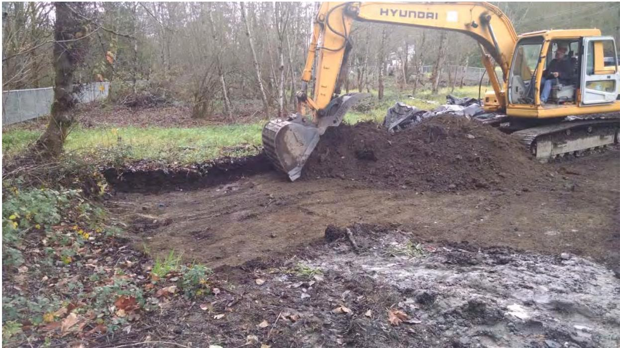
Northeast corner of excavation (as of November 28, 2018), looking east. Area required deeper excavation due to presence of debris below surface.
