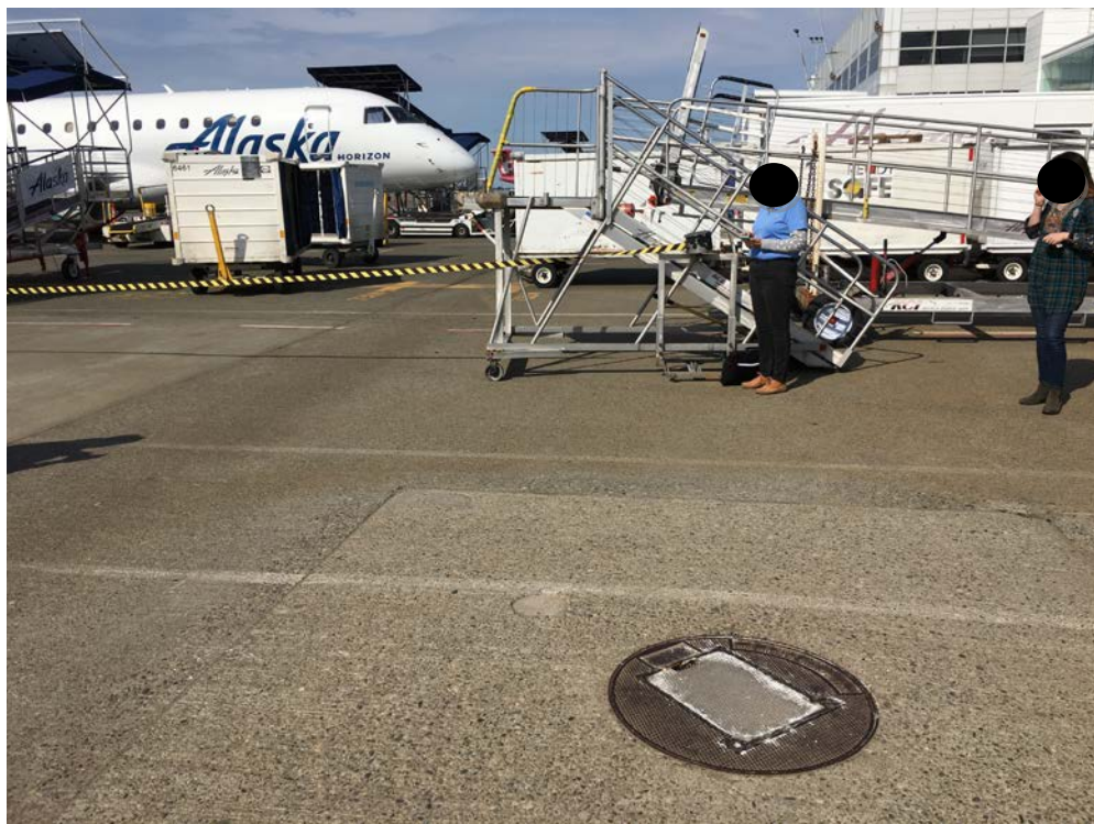
Photo 3: Closed hydrant fuel line access pit (filled with concrete with metal lid on top).
