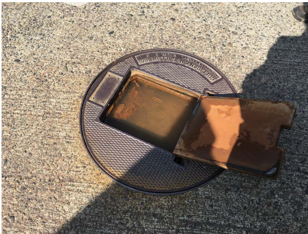
Photo 4: Closed hydrant fuel line access pit (filled with concrete with metal lid on top).
