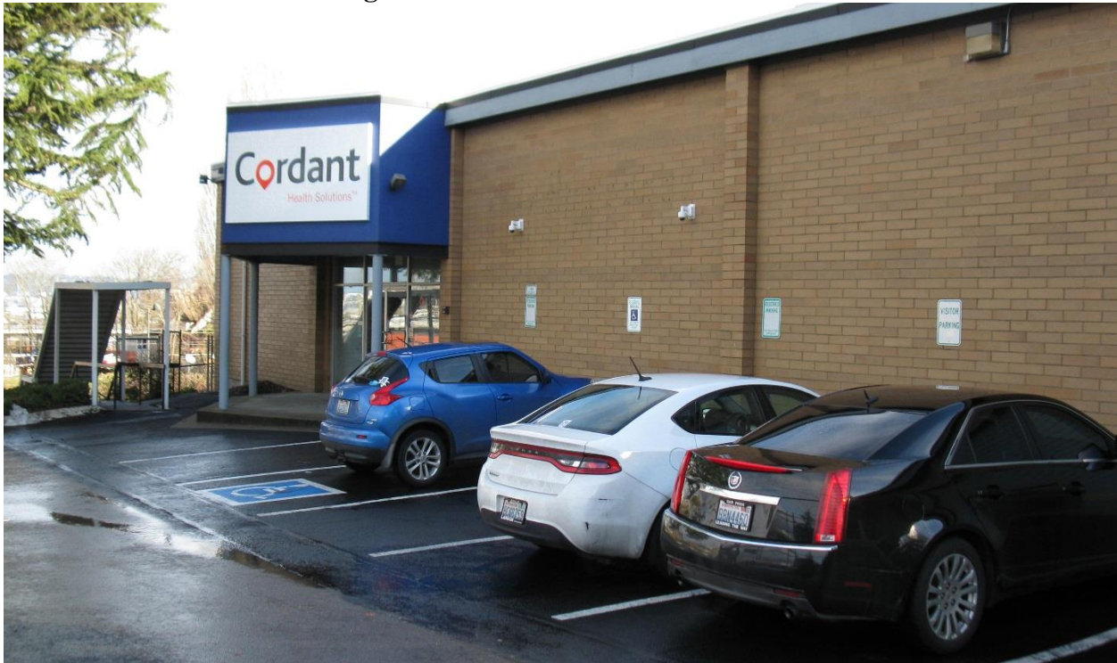
Photo 1: Front of the Building – From Northeast
