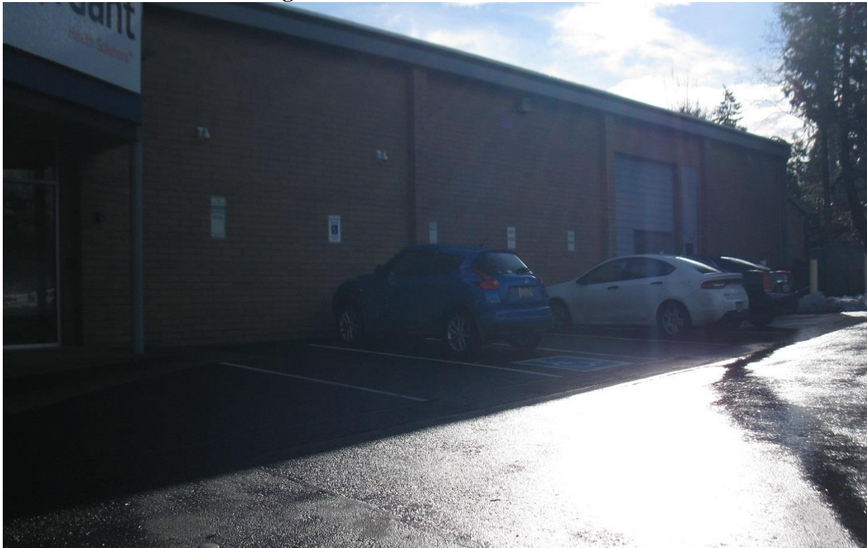
Photo 2: Front of the Building – From Southeast
