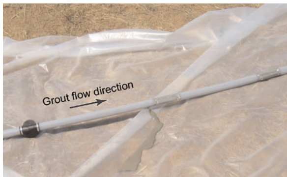
Figure 6 Grout exiting vent hole during pre-installation grouting.
