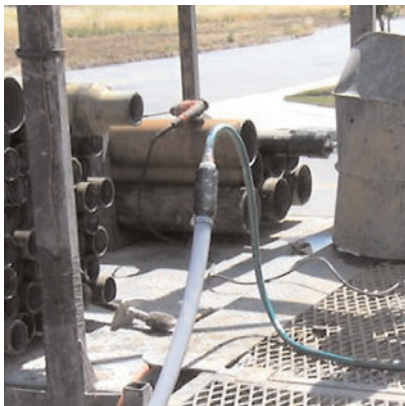
Figure 5 Pre-installation grouting of CMT by injection using a grout boot device.
